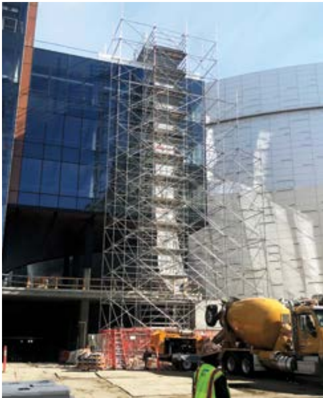
Fig. 3: Self-supporting scaffold tower
