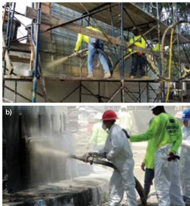
Fig. 4(a) and (b): CROM nozzlemen certification testing
