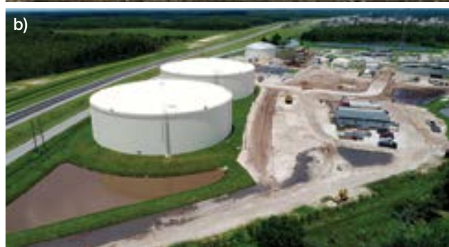
Fig. 3(a) and (b): CROM prestressed concrete tanks
