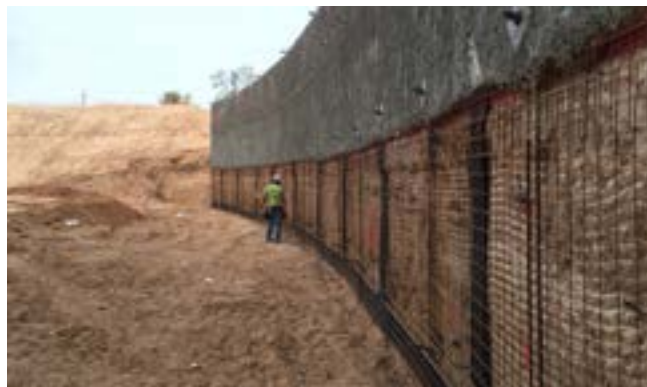
Fig. 3: Soil nail facing at Phoenix Children's Hospital on radius walls
