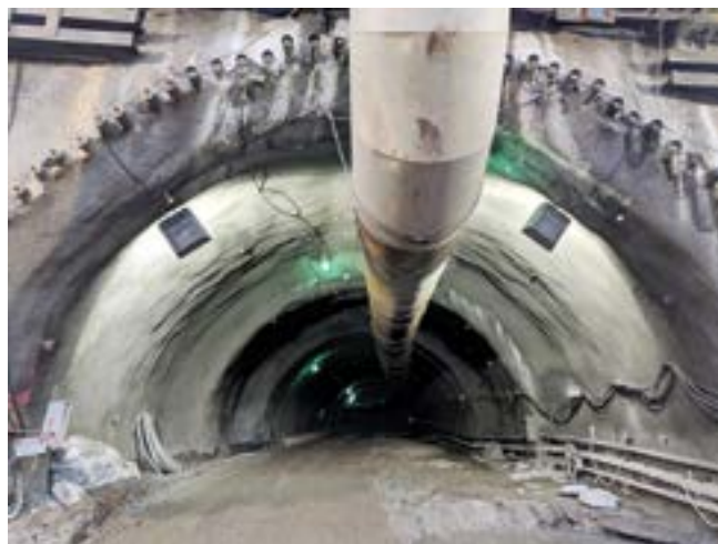
Fig. 2: Plymouth Tunnel East Portal top heading excavation
