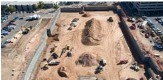
Fig. 1: Aerial view of basement soil nail shoring and radius wall
