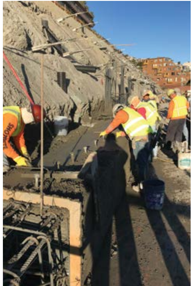
Fig. 2: Grade beam during shotcrete installation
