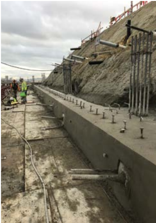
Fig. 3: Finishes on grade beam
