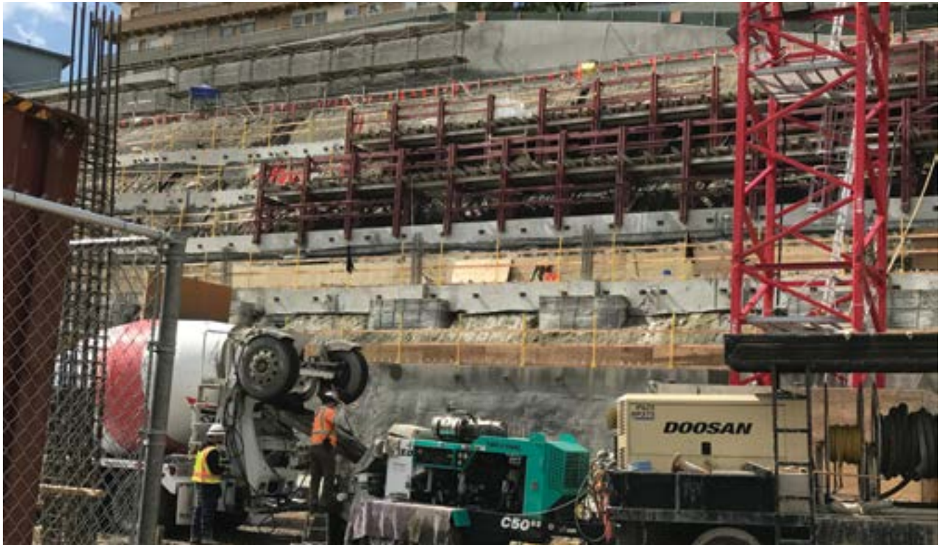
Fig. 5: View of the jobsite with multi levels of grades beams and rear retaining wall to the project
