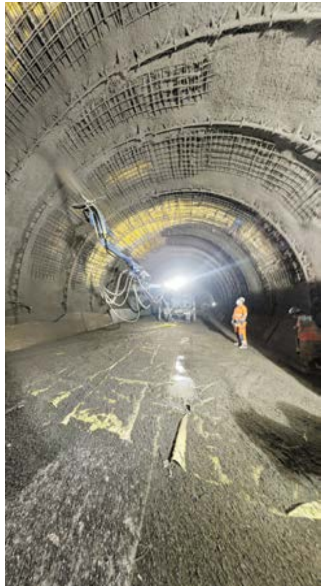
Fig. 7: Spraying secondary liner bays between arches
