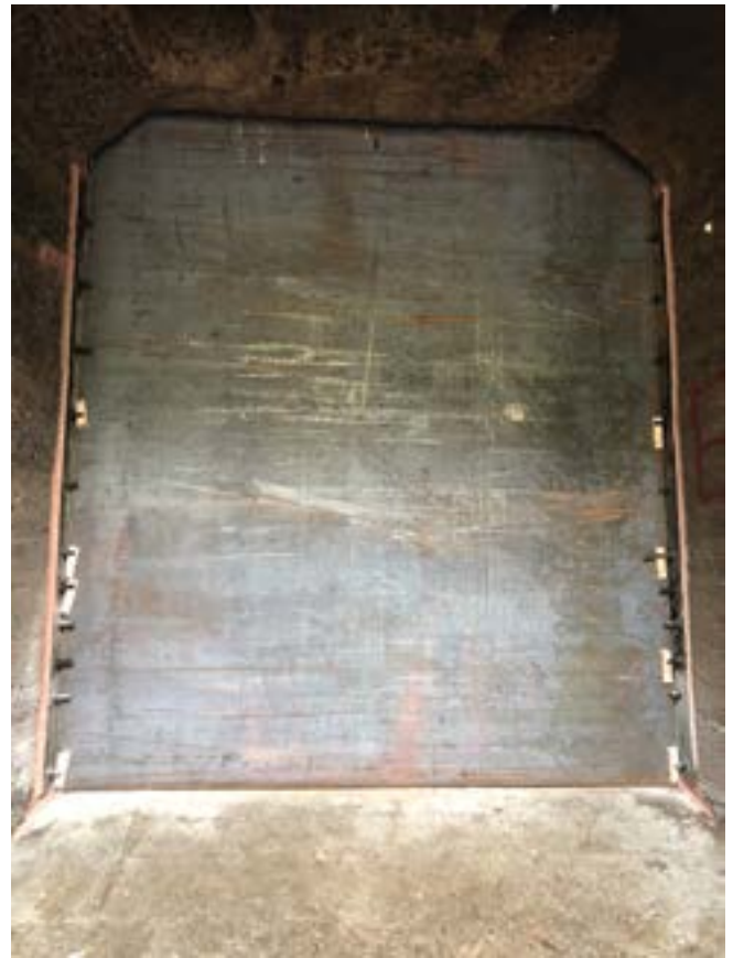
Fig. 1: Temporary safety bulkhead
