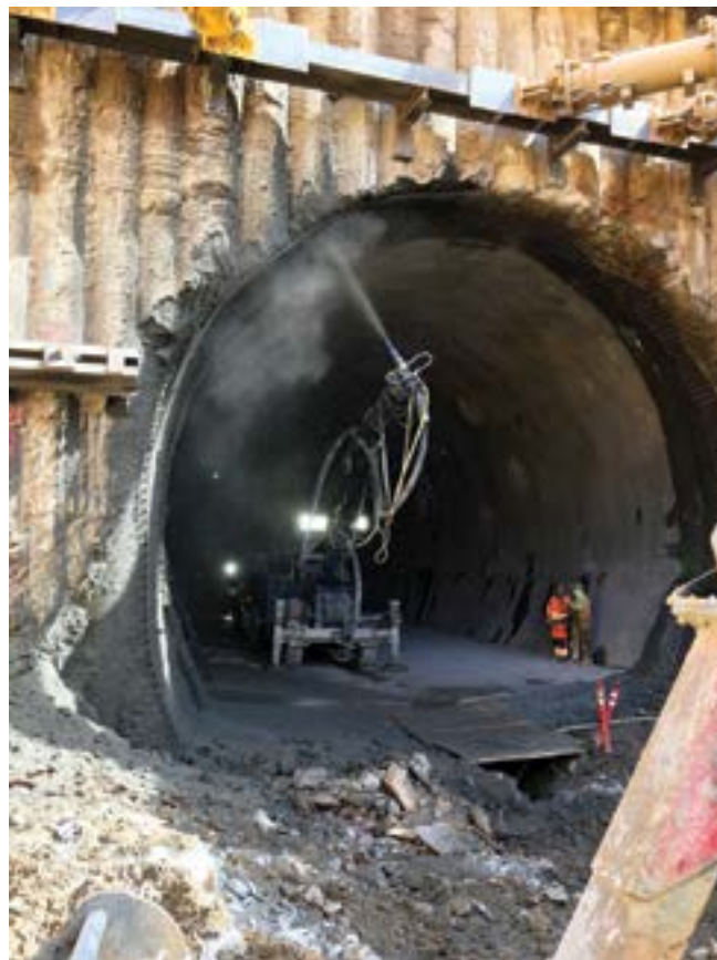
Fig. 4: Completion of initial lining after excavation
