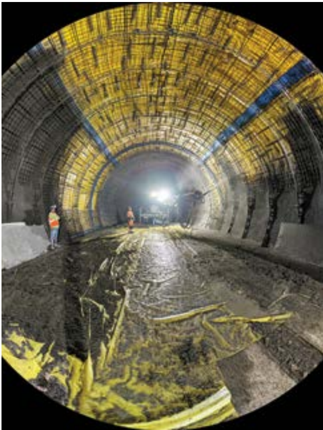
Fig. 9: Initial shotcrete application on PVC liner
