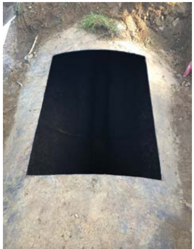
Fig. 2: Excavated manhole access
