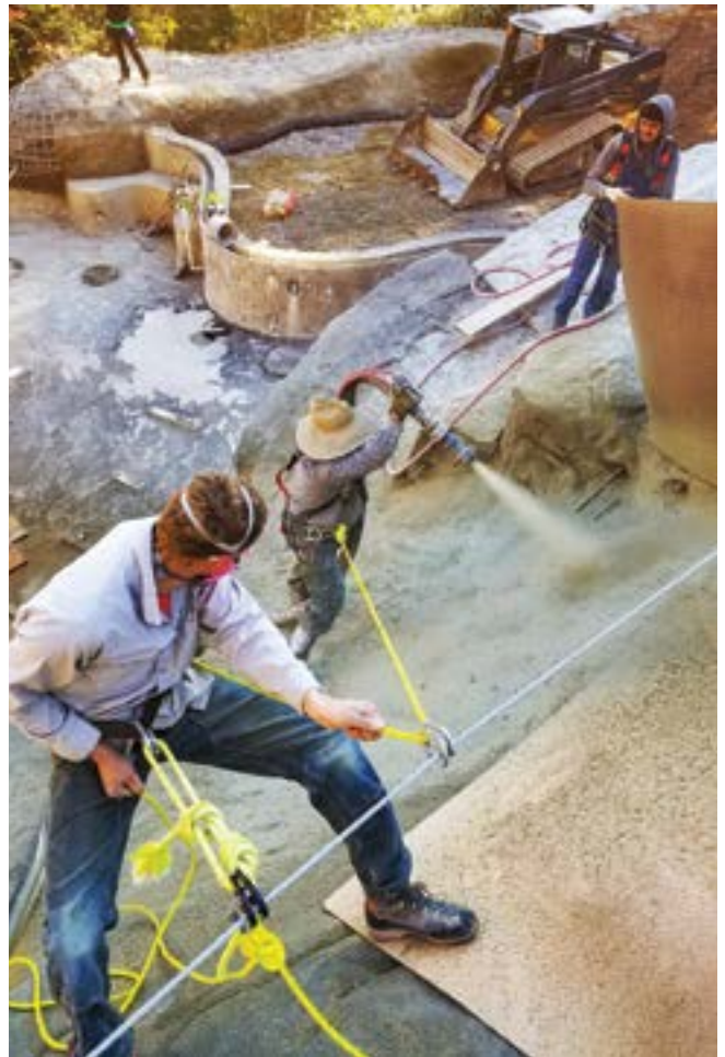
Fig. 4: Nozzlemaster shooting the steep rock face while being suspended on belay
