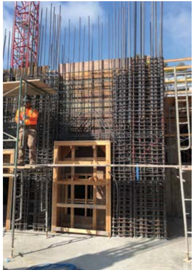
Fig. 4: Typical shear wall and boundary elements
