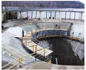
Fig. 2: Scaffolding for Glory Hole Spillway
