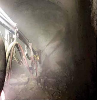
Fig. 2: The admixtures play an important role in the production of this underground shotcrete placement
