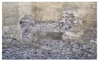
Fig. 6: Severe surface scaling on the concrete
