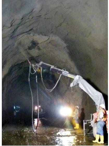
Fig. 1: QUIKRETE Shotcrete MS used for a tunnel relining
