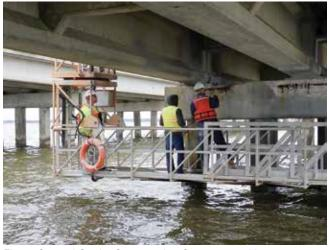
Fig. 4: Coastal Gunite Construction Company and Inspector testing for continuity
