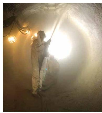
Fig. 5: Dry-mix shotcrete application in hydro penstock
