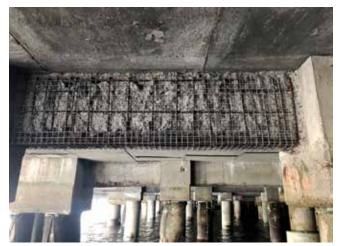
Fig. 2: A Type 3 repair with preparation completed. The repair is awaiting the application of shotcrete
