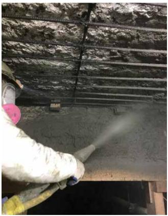
Fig. 4: Shooting on underside of pier
