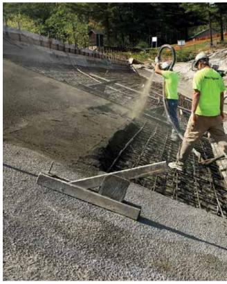
Fig. 3: QUIKRETE Shotcrete MS used for a dam rehabilitation
