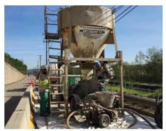
Fig. 7: Material hopper, predampener, and continuous-feed rotary gun setup for gunning prepackaged shotcrete repair mortar
