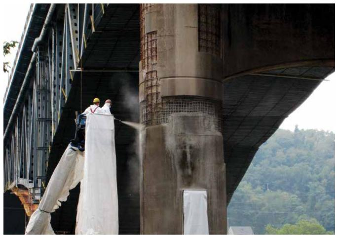
Fig. 2: QUIKRETE Shotcrete MS used for a bridge pier restoration
