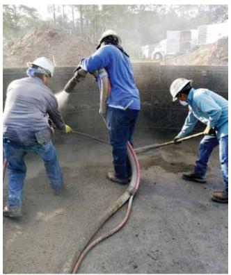
Fig. 6: Maintaining a clean substrate is a very active procedure. It helps to have a finisher using a Fresno to remove excessive rebound
