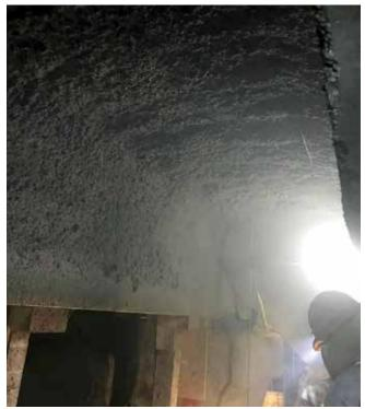
Fig. 3: Shotcreting in limited space under pier
