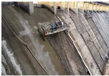
Fig. 6: Stevenson Dam Spillway resurfacing
