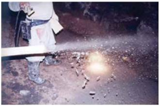
Fig. 4: Shotcrete is pneumatically projected concrete accelerated to high speed before impact on the receiving surface
