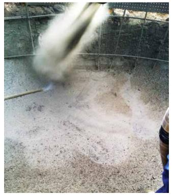
Fig. 5: Using an air lance is critical to maintaining a clean substrate during the shotcrete process. Without the air lance the substrate will develop a layer of overspray and rebound that will prevent bonding of the new material to the existing material
