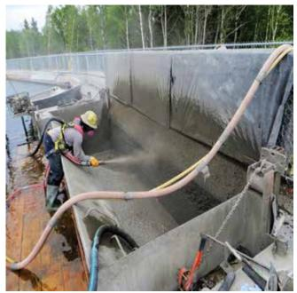
Fig. 1: Remote dam repair using dry-mix shotcrete and a cofferdam<sup>1</sup>
