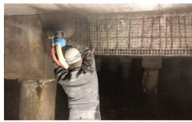
Fig. 3: An ACI Certified Nozzleman applying shotcrete to a Type 3 repair
