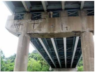
Fig. 3: When reinforcing bars close to the concrete surface corroded, the expansion of the rust spalled concrete off the rusted bars
