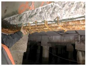
Fig. 1: A Type 3 repair after deteriorated concrete was removed
