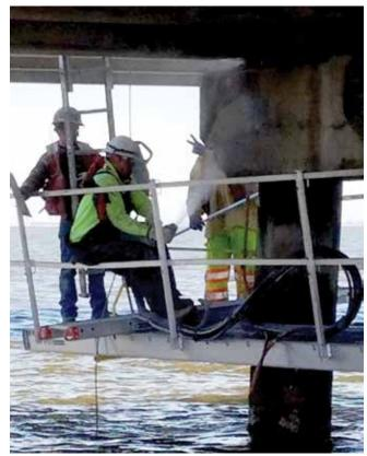
Fig. 3: Nozzlemen shooting back damaged bent cap
