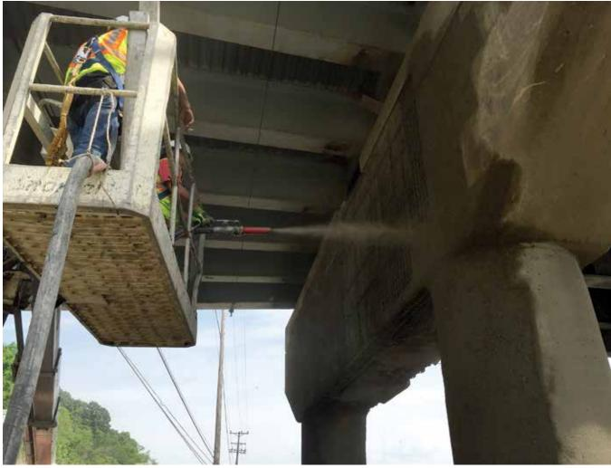
Fig. 4: Dry-process shotcrete placement on a bridge pier
