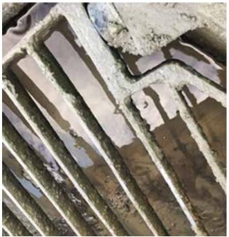
Fig. 1: Obviously too much water on top of the concrete in the hopper
