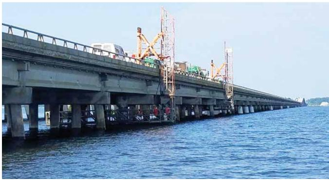
Fig. 7: Anderson Hydra-Platform Bridge Access Machines in use
