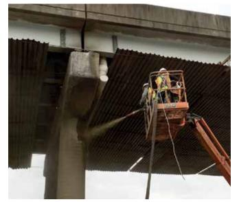
Fig. 8: Gunning of prepackaged material on bridge pier. We were required to repair one side of the piers at a time
