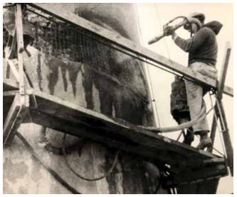
Fig. 1: Dry-mix shotcrete repair on a paper mill stack (image from 1960s)
