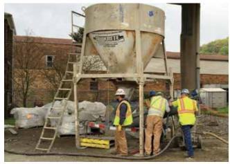
Fig. 6: Equipment setup for gunning prepackaged material
