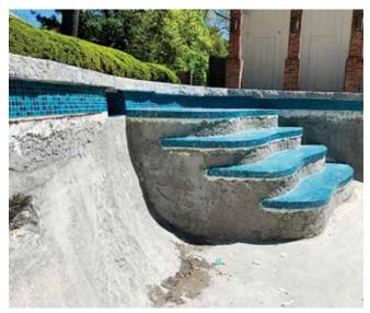
Fig. 3: Interlocking three-dimensional bond plane between new shotcrete and existing shotcrete
