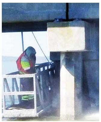
Fig. 5: Preparing to apply zinc anode
