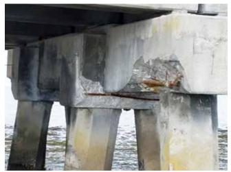
Fig. 2: Repair location on bent cap
