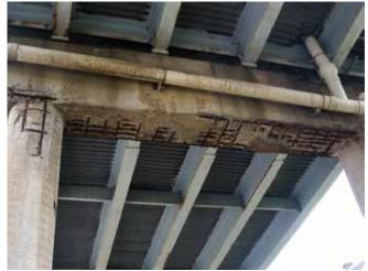
Fig. 2: All but one of the bridge piers had deterioration where repairs were necessary
