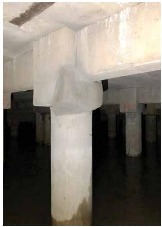
Fig. 4: A completed Type 4 repair
