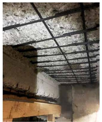
Fig. 2: Underside of pier ready for shotcrete
