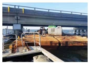
Fig. 8: Barge system for metalizing operations
