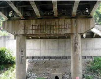
Fig. 5: Because of concerns about the condition of this pier the repairs were performed in four phases
