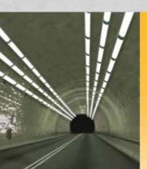
When Pittsburgh's 80-year-old Liberty Tunnels needed structural repairs, QUIKRETE® Shotcrete MS got the job done. Crews were able to complete their work within tight time constraints using the dry process with a pre-dampener. In fact, our shotcrete products were part of the American Shotcrete Association's "Outstanding Underground Project" for 2009 and 2010.
