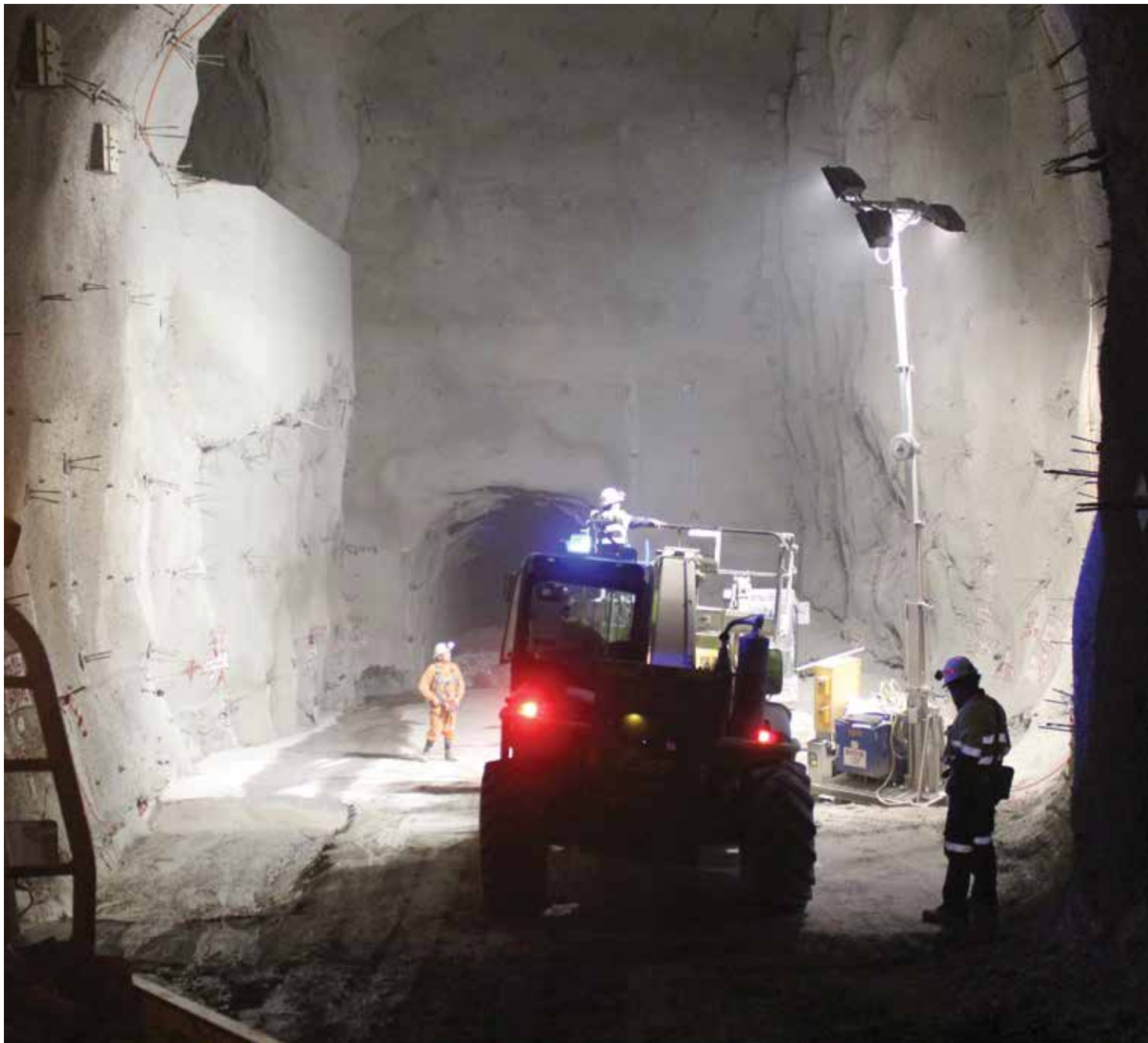
Fig. 4: Shotcreted transfer chamber
