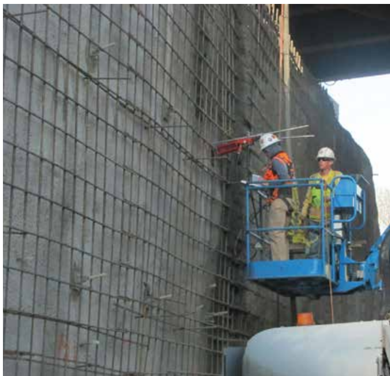
Fig. 3: Manlifts were used to address the wall because scaffolding was not an option so close to the railroad
