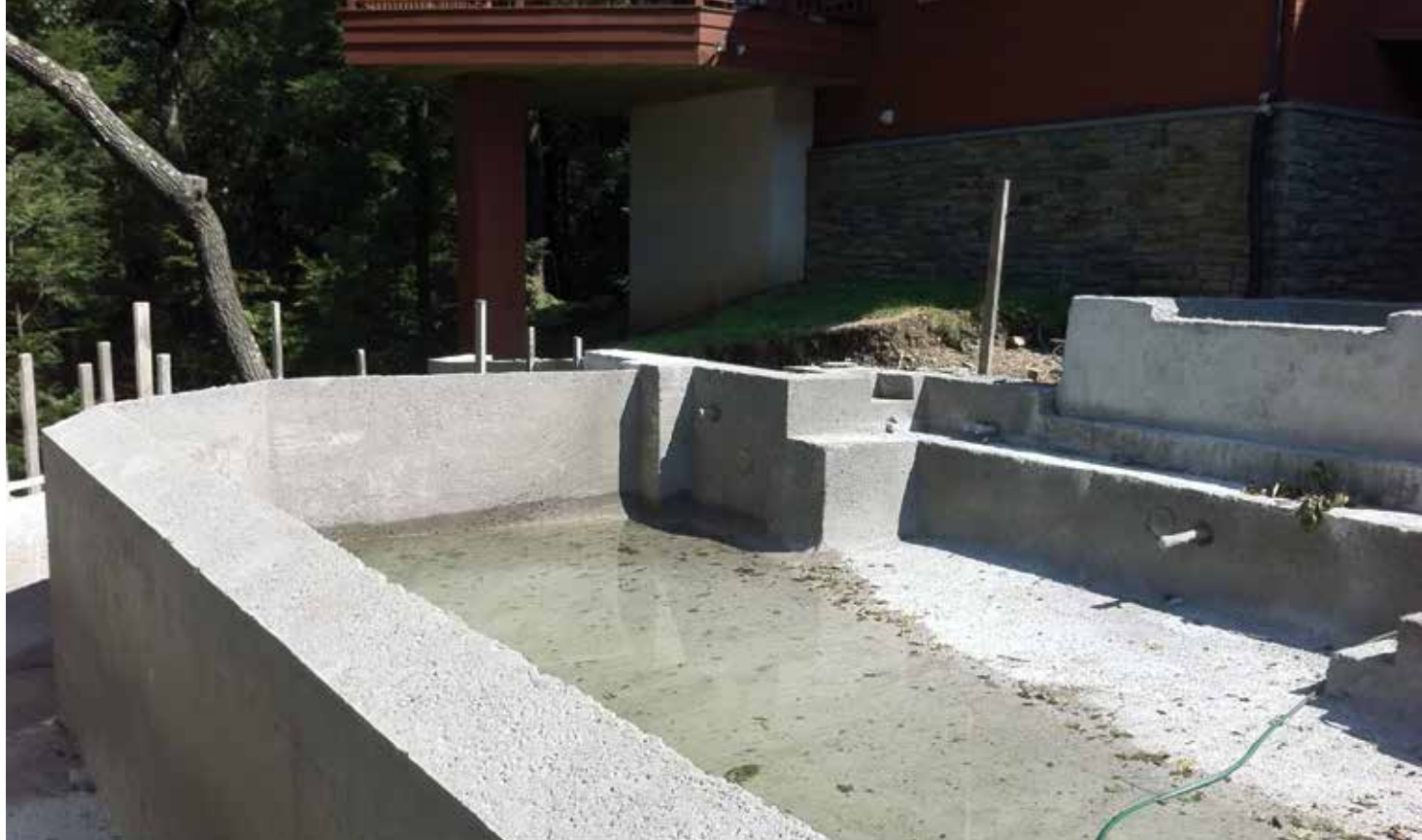
Fig. 8: Completed shotcrete structure undergoing 28-day wet cure to achieve high strengths of 6000 to 7000 psi (40 to 48 MPa)
