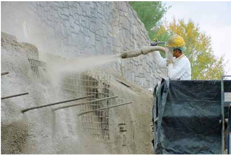
Fig. 6: Shotcrete placement
