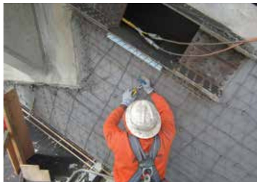
Fig. 4: Repairing mesh prior to shoot
