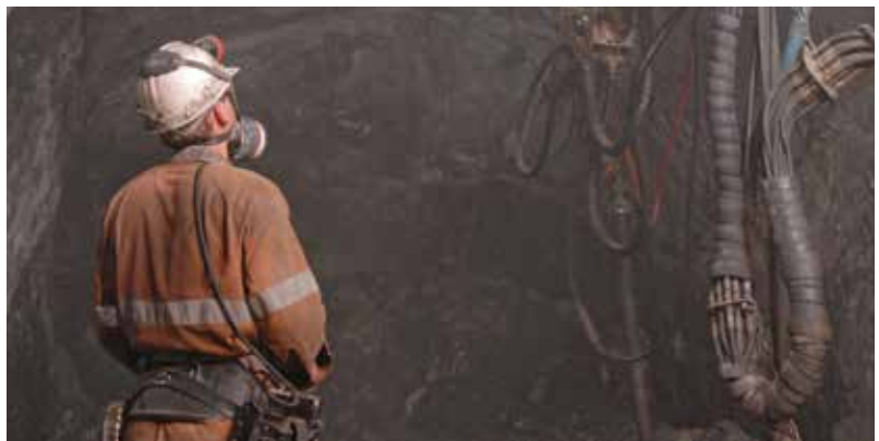
Fig. 5: Nozzlemán spraying heading with robotic spray rig
