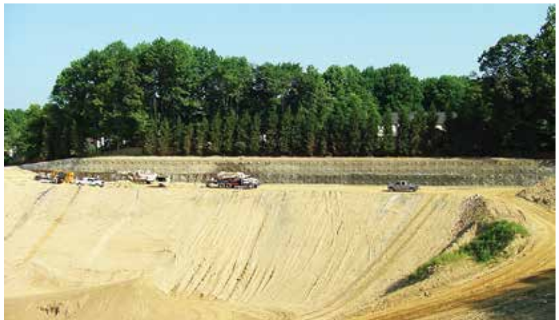
Fig. 4: Access roads were built and drilling commenced, closely followed by nail grouting and wire mesh installation
