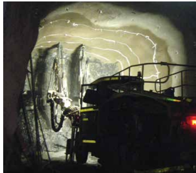
Fig. 2: Jumbo drill rig installing rockbolts through shotcrete
