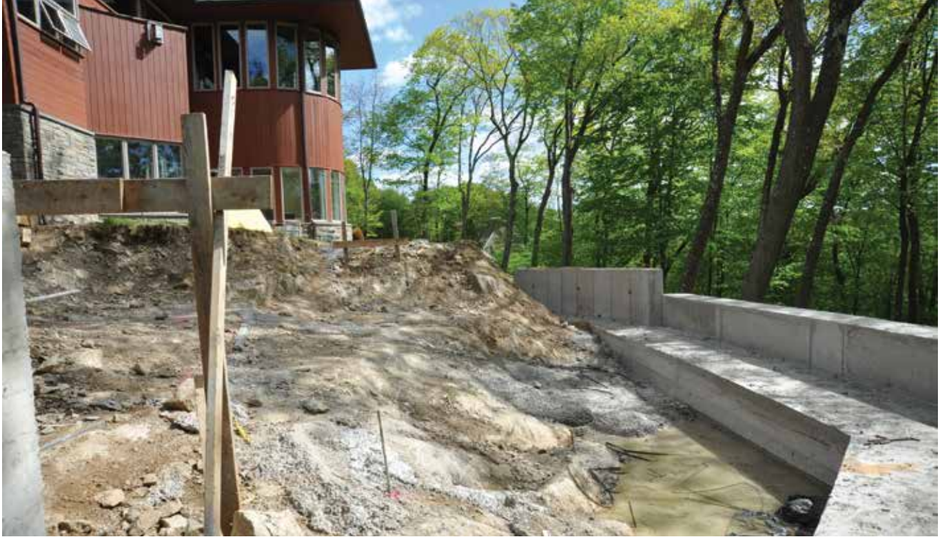
Fig. 5: Cast-in-place concrete footing to support pool structure
