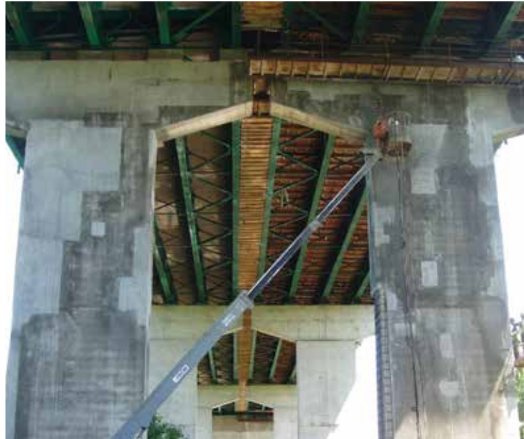
Shoring, forming, and casting this repair would be extremely difficult, but shotcrete makes it easy
