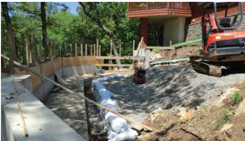
Fig. 7: Extensive formwork required for cast-in-place concrete
