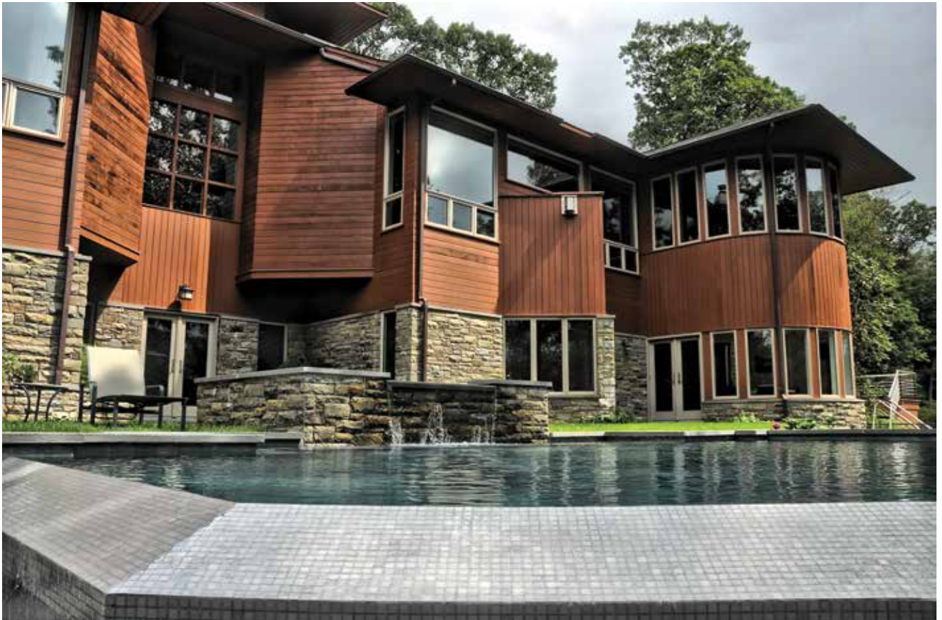
Fig. 10: Glass tile applied to weir wall and vanishing edge
