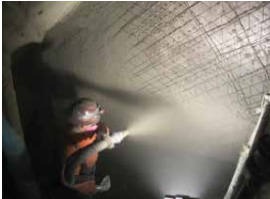
Fig. 2 and 3: Shotcrete placement inside the arches
