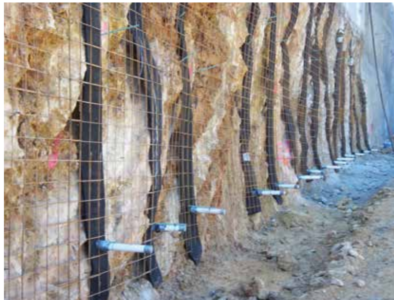
Fig. 1: Drain board and weep pipes were incorporated before applying the shotcrete to allow for drainage
