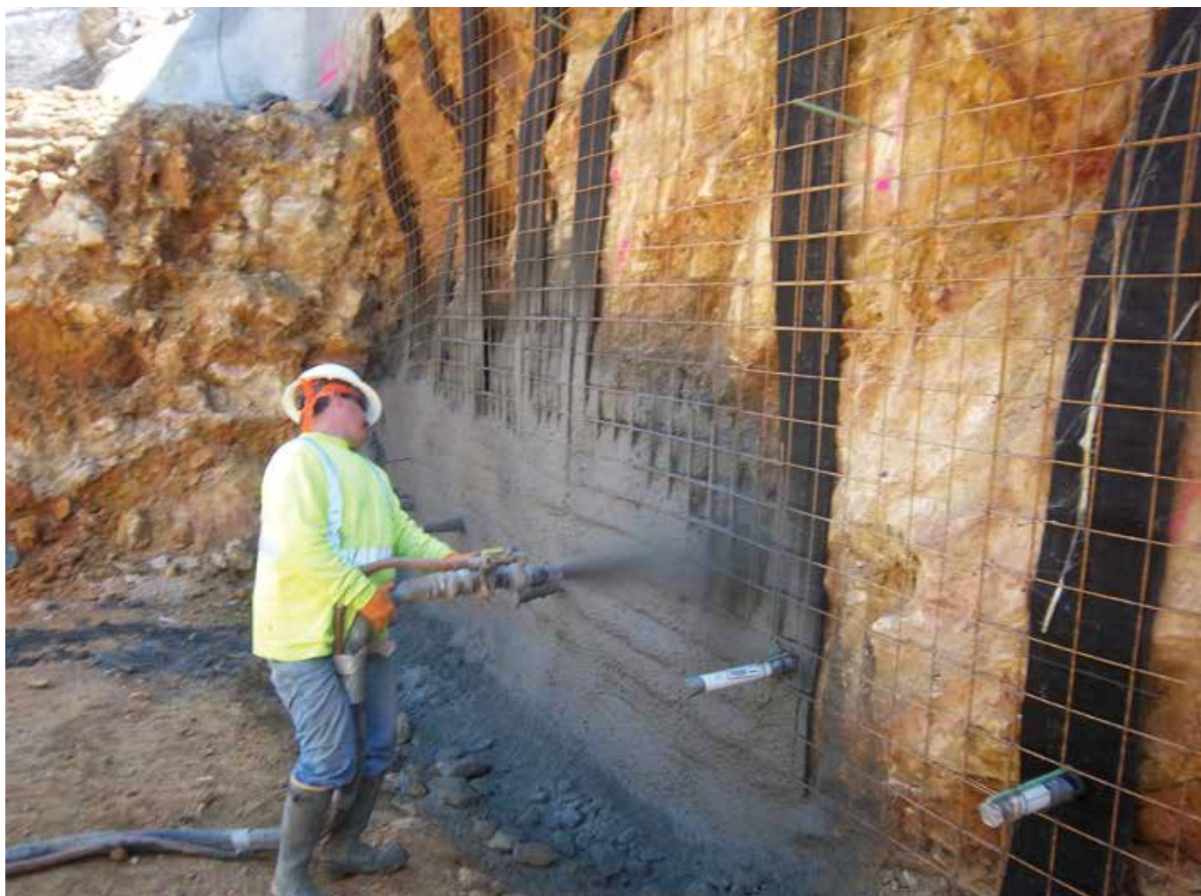
Fig. 2: An initial layer of shotcrete was applied to stabilize the drill bit during the drilling operation
