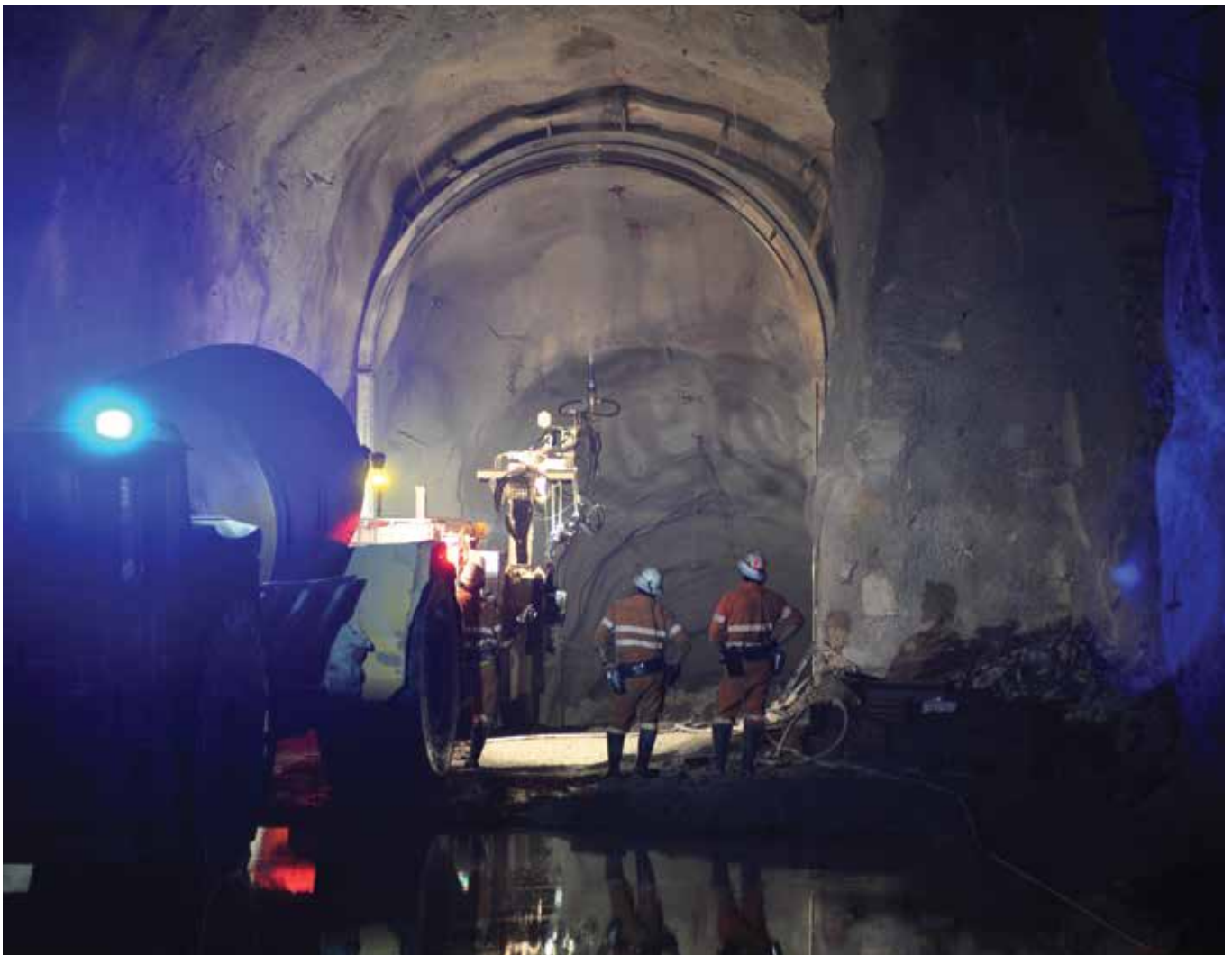
Fig. 10: Shotcrete rig and agitator truck in one of the many underground chambers
