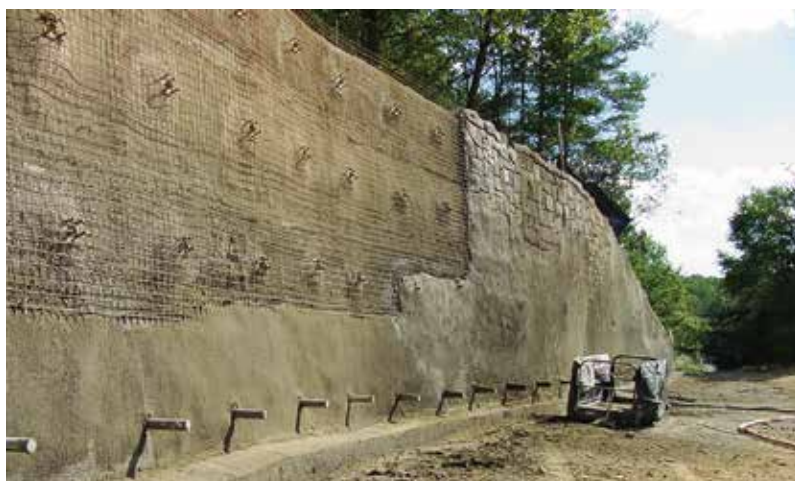
Fig. 2: Top wall being transformed with faux-rock finish
