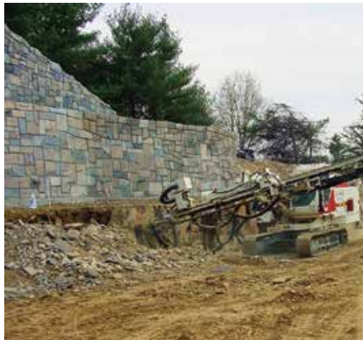
Fig. 5: Soil nailing
