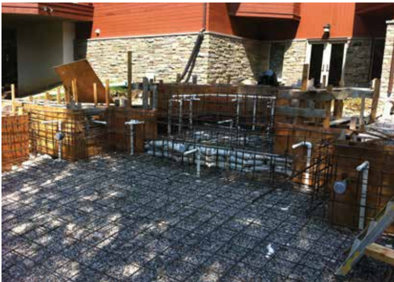
Fig. 6: Intricate but efficient formwork, steel, and plumbing installation prior to shotcrete placement
