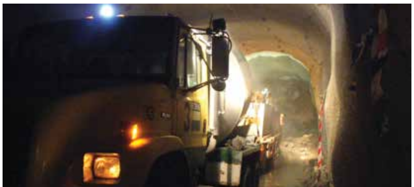
Fig. 7: Agitator truck reversing up to shotcrete spray rig
