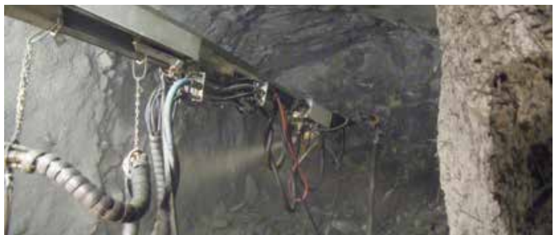
Fig. 6: Shotcreting in progress in undercut drill drive
