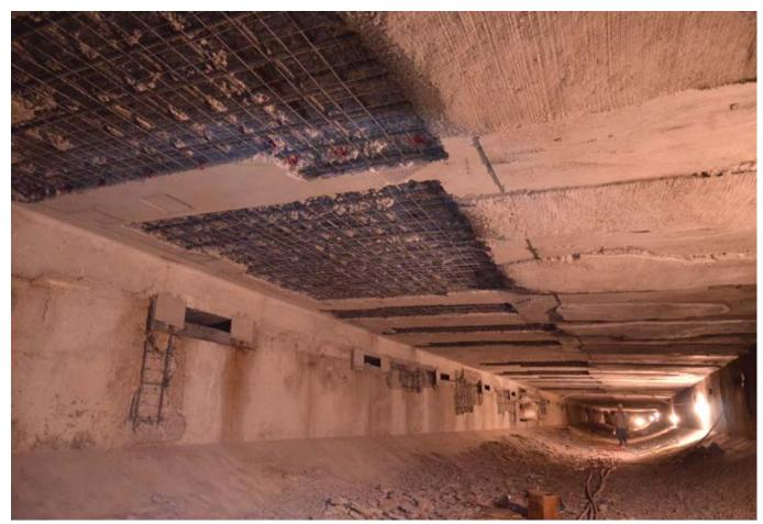
Fig. 4: Areas after hydrodemolition and hand chipping behind reinforcing steel ready for shotcrete
