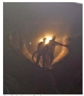
Fig. 3: In this confined space area in a power plant ash pit, dry-process shotcrete is being gunned in place
