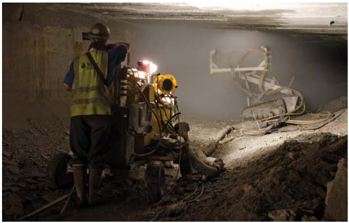
*Fig. 3: Hydrodemolition robot in action removing overhead concrete*
