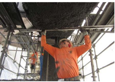
Fig. 8: Overhead finishing
