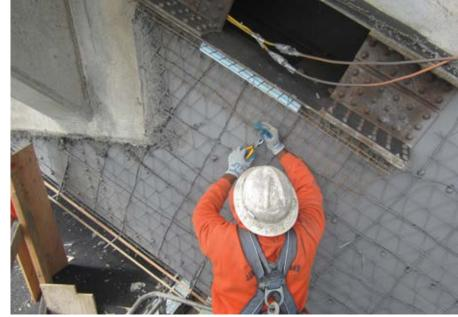
Fig. 4: Repairing mesh prior to shoot
