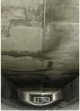
Fig. 6: Completed ceiling and wall rehabilitation
