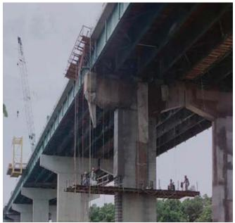
Fig. 2: 50 x 6 ft (15 x 2 m) platforms used to perform work
