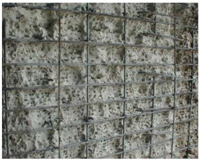
Fig. 1: A concrete surface after hydrodemolition
