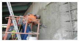
*Fig. 2: Screeding new rapid-setting, lowpermeability shotcrete*
