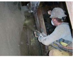
Fig. 3: Application of shotcrete on shaft wall
