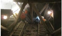
Fig. 2 and 3: Shotcrete placement inside the arches
