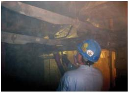
Fig. 4: Nozzleman shooting overhead in a tightly confined area. In areas where visibility and ventilation are concerns, adequate lighting should be provided and the appropriate personal protective equipment should be worn
