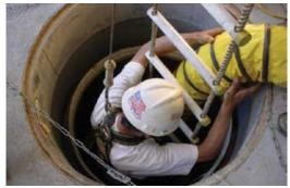
*Fig. 1: Worker entering a manhole opening into a confined space along the side of a ventilation tube*
