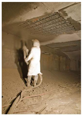
Fig. 5: Placing overhead wet-mix shotcrete
