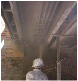
Fig. 4: Close-up of shotcrete placement
