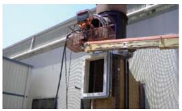
Fig. 2: In confined areas like this steel mill smokestack and ductwork, a refractory lining is being gunned in place using the dry process
