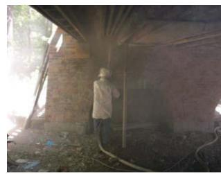
Fig. 3: Placement of shotcrete under confined working conditions
