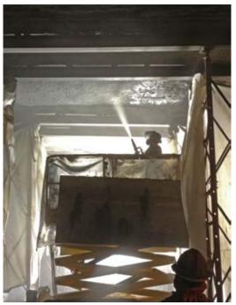
Fig. 3: Nozzleman shooting on the scissor lift between the temporary shoring
