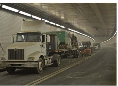
Fig. 1: Mobile shotcrete equipment in tunnel (work is underneath road deck)
