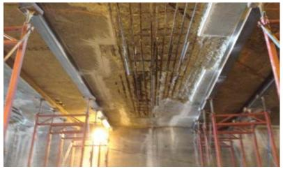
*Fig. 1: Shoring towers at 8.5 ft (3 m) apart made for tight access between the exposed deteriorated concrete*
