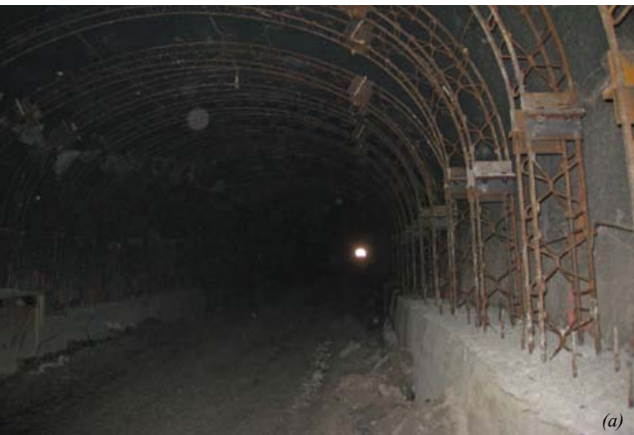
Fig. 1: (a) and (b) Steel lattice trusses in place and ready for shotcrete
