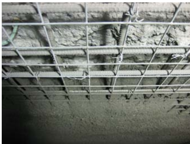
Shotcrete encapsulating the reinforcing bar
