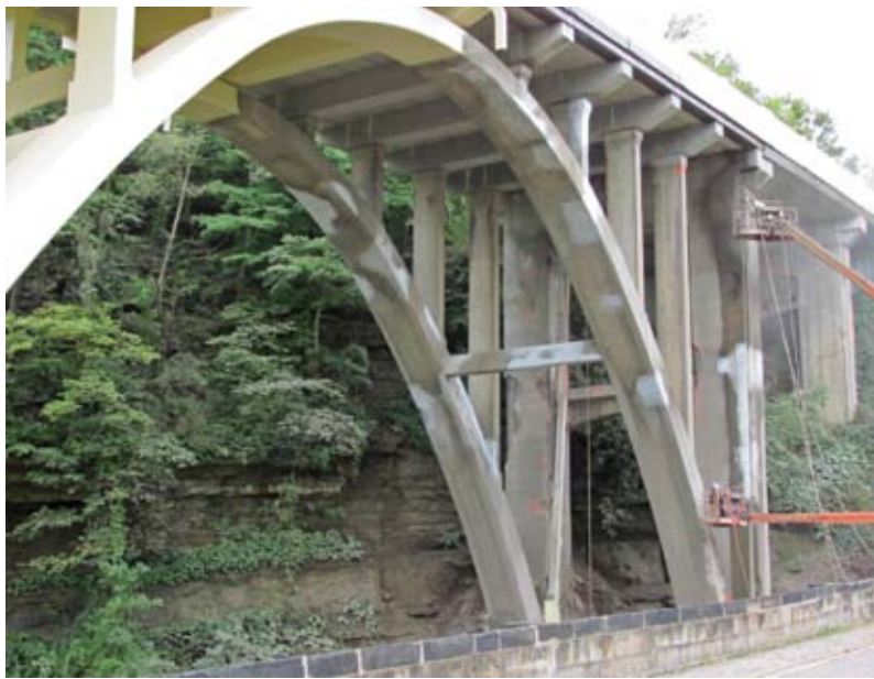
Fig. 4: Open spandrel arch and spandrel column rehabilitation
