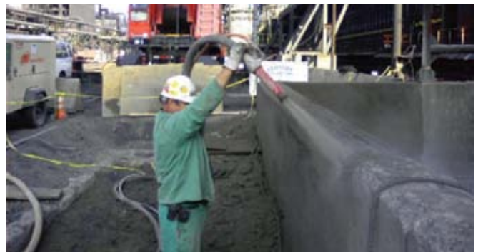
In this dry-process shotcrete repair of an industrial sump, the repair mortar is gunned in place without the need to make or install forms
