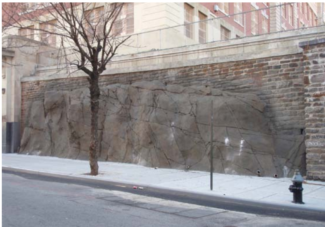
Fig. 6: Final stabilized rock mass
