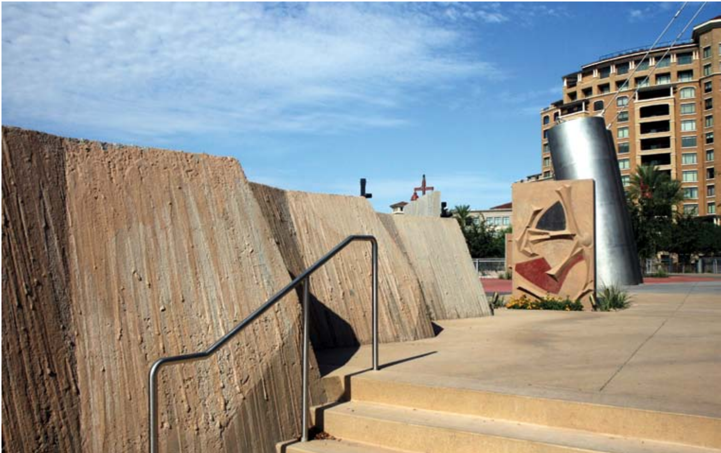
Drip method and earth-cast wall
