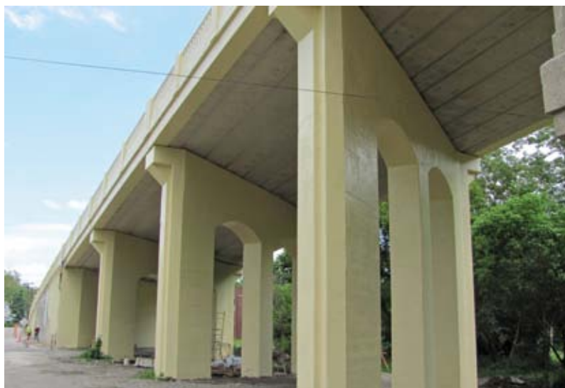
Fig. 3: Rehabilitated columns with tintable epoxy urethane sealer
