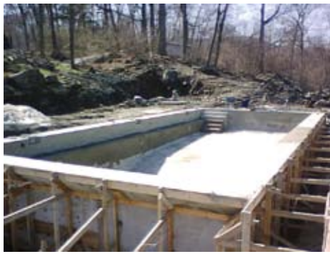
Pool shotcreted, waiting for forms to be stripped
