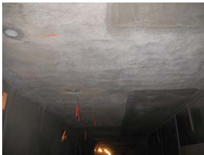
Core testing for bond and compressive strength was taken from these locations
