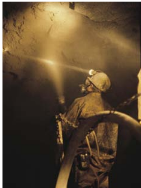
Nozzleman applying shotcrete to back in order to provide ground support during the mining process
