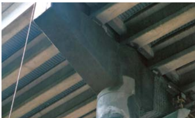
On this pier hammer head, the shotcrete is easily gunned in place without the need for forming
