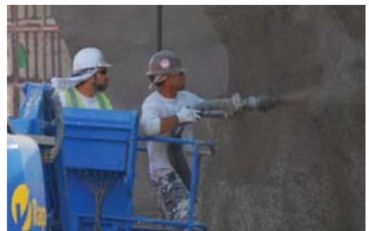
Fig. 2: Shotcreting by Imagineering
