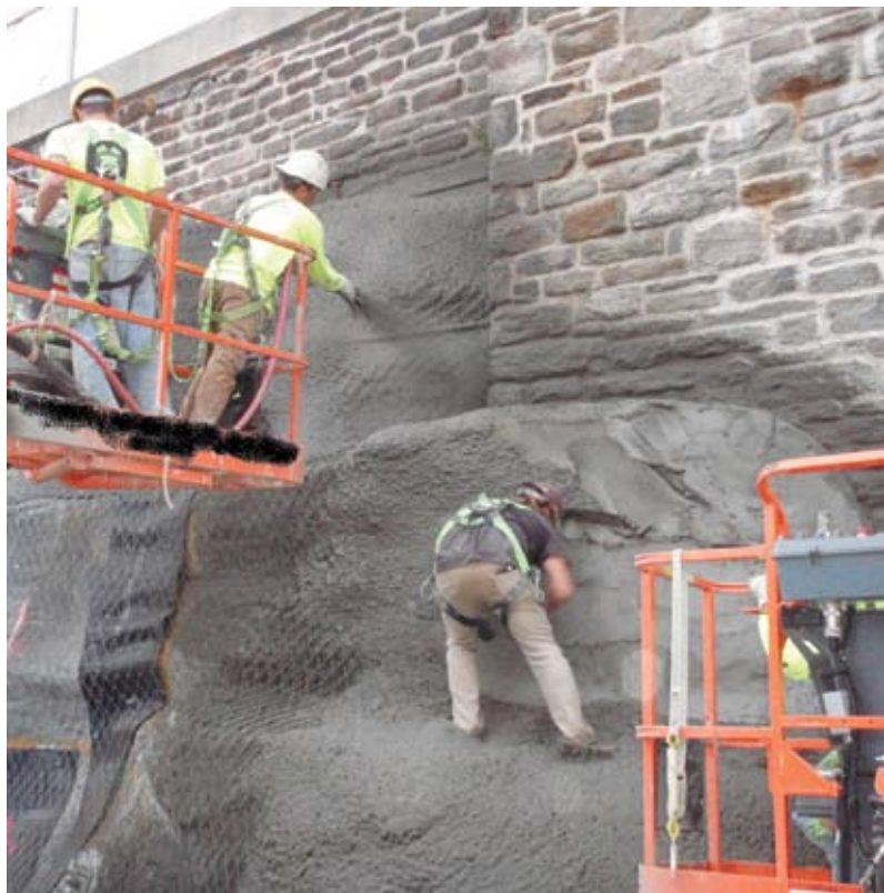
Fig. 4: Applying and sculpting shotcrete
