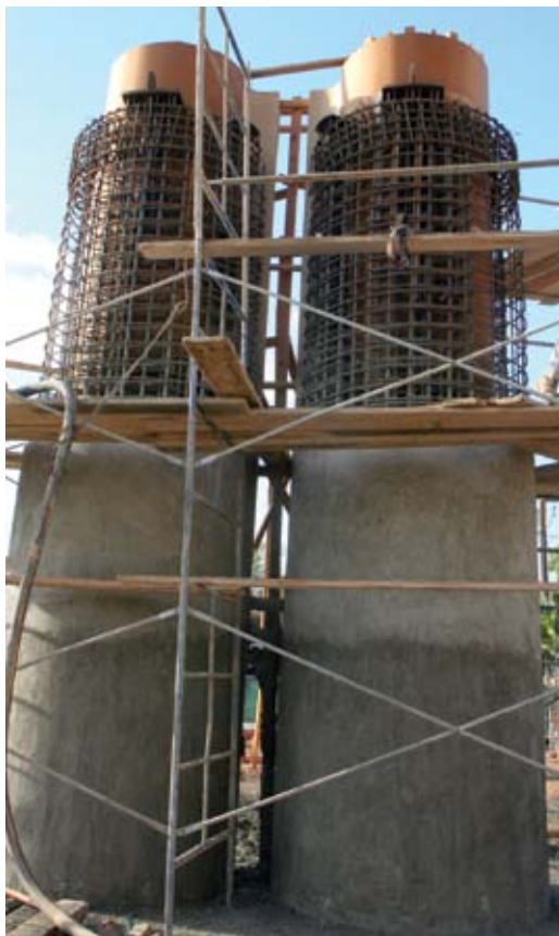
Anchor pylons shot using a template
