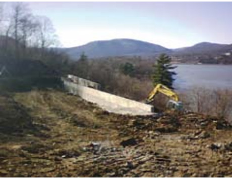
Shotcrete walls in place before being backfilled
