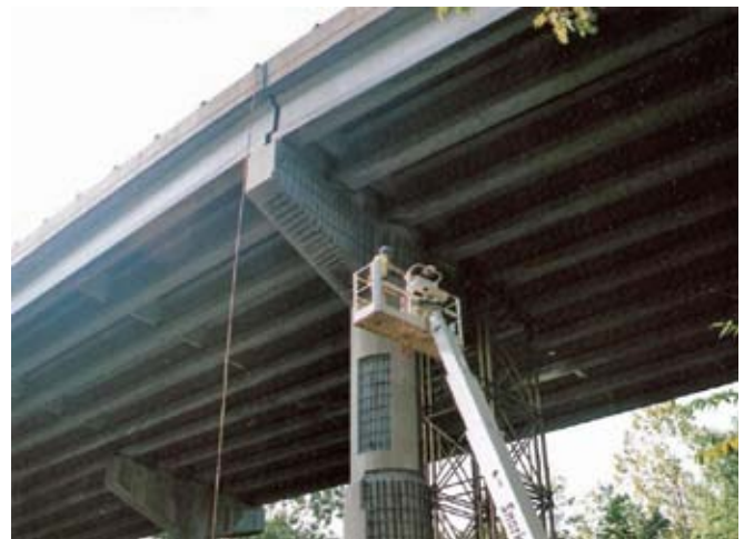
The deteriorated concrete on this bridge pier has been removed, the reinforcing bar exposed, and the surface prepared prior to the shotcrete placement. The use of shotcrete eliminates the need for forming and labor costs involved
