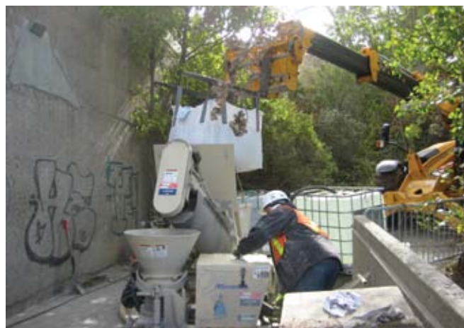
Equipment setup. Bulk bags were used
