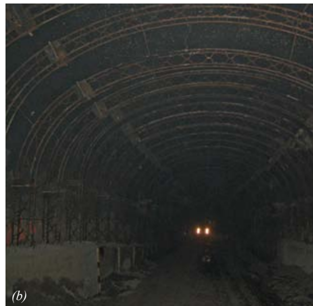
Fig. 1: (a) and (b) Steel lattice trusses in place and ready for shotcrete
