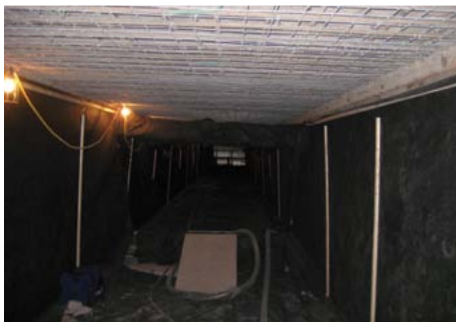
Underside of deck ready for shotcrete placement
