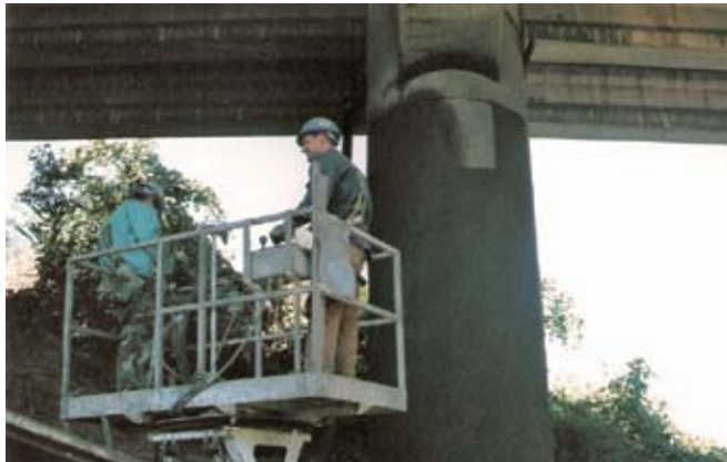
Shotcrete can easily conform to rounded or irregular shapes and varying depths, as illustrated by this freshly gunned circular-shaped bridge pier
