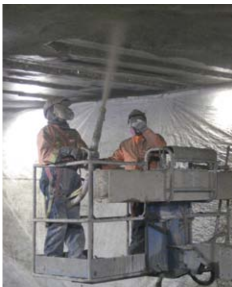
Nozzleman applying shotcrete overhead to repair concrete soffit in tunnel
