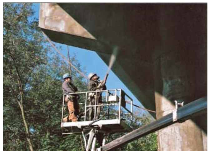
Shotcrete can be efficiently gunned overhead in concrete repair applications, where forming and material placement can be difficult and expensive, as evidenced by this dry-process shotcrete repair
