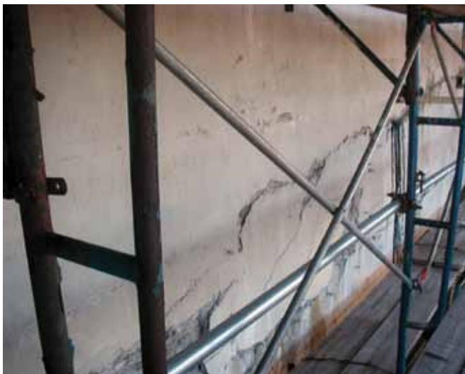
Typical minor concrete spalling
