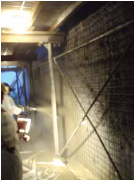
Prepackaged fiber-reinforced wet-mix shotcrete was applied
