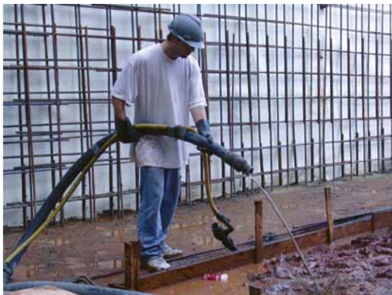
Fig 2: Line lubricant discarded outside the work area
