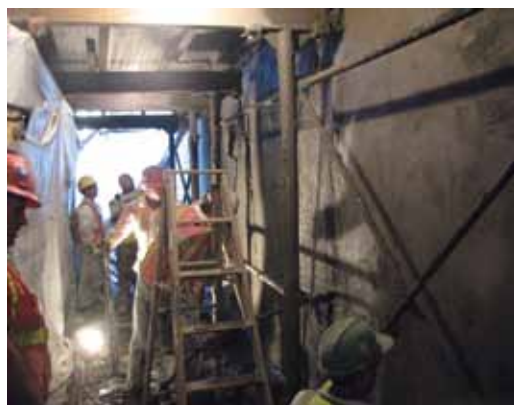
Wet-mix shotcrete was the only acceptable method the engineer would entertain to minimize and control the dust and rebound
