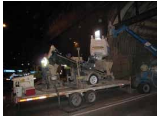
The 3000 lb (1361 kg) bulk bags were predampened as a part of the installation process
