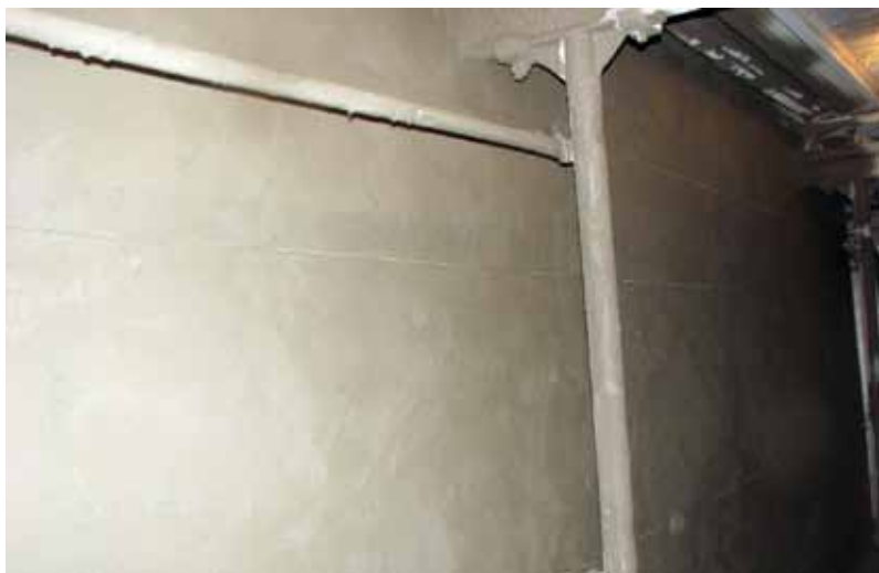
The uniformed float finish provided an excellent textured surface for the coating adhesion
