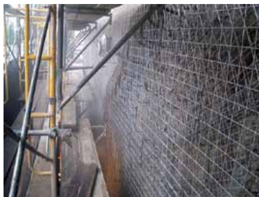
Double and triple mats of 4 x 4 in. (100 x 100 mm) welded-wire reinforcement installed in severely deteriorated locations
