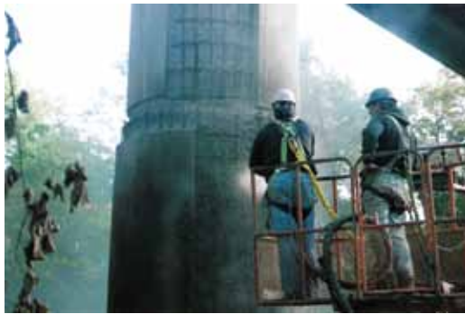
With good surface preparation and gunning practices, shotcrete provides an excellent bond to the existing substrate
