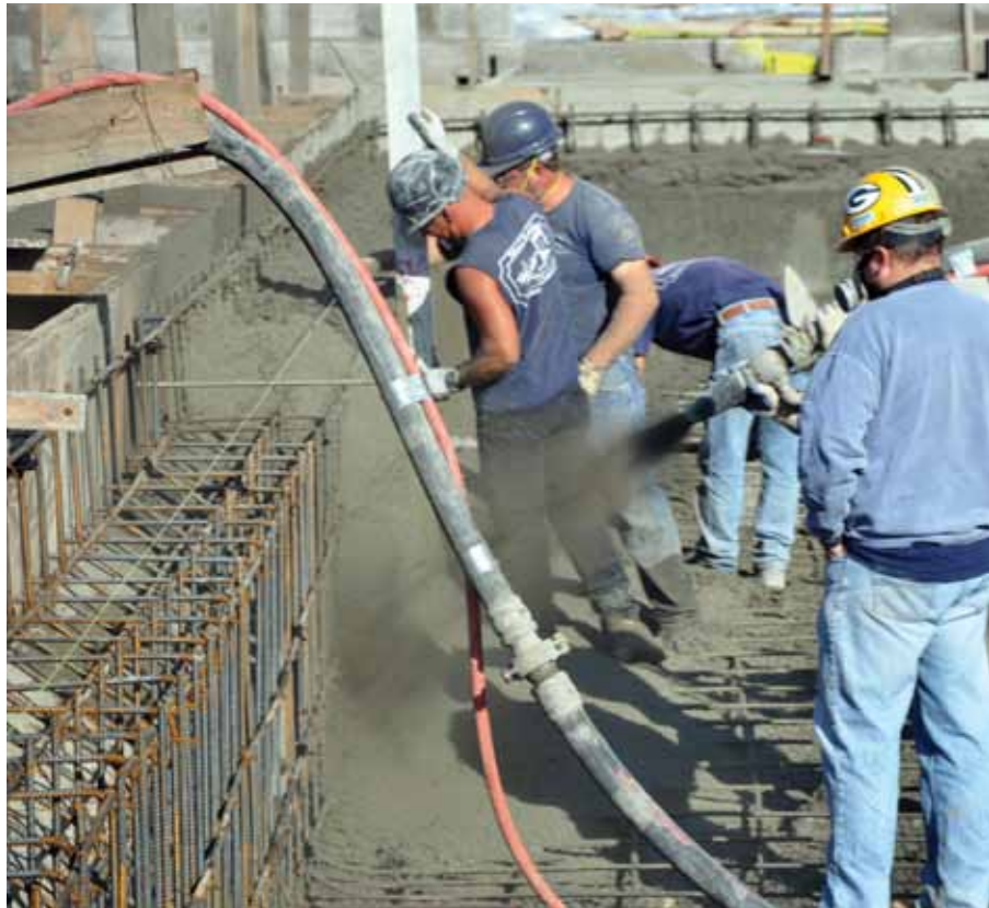
Shotcrete phase of the lap pool
