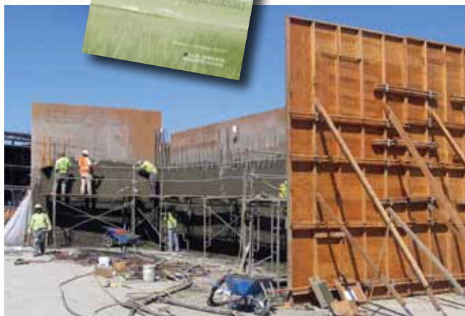
Shotcrete sprayed in place against one-sided forms saves 50% of the forming required in cast-in-place installations
