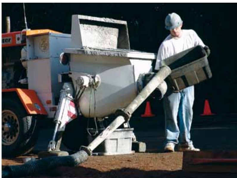
Fig 1: Line lubricant added directly to placement system
