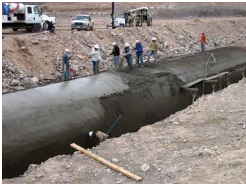
Shotcrete placement on arch culvert at Inspirada in Henderson, NV
