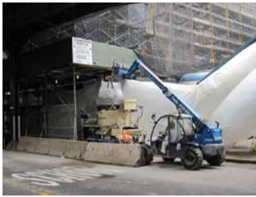
A self-contained machine was selected—one that far exceeded the necessary requirements for mixing volume and pumping distance and was capable of mixing bulk bags
