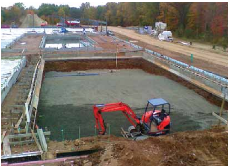
Foreground: competition pool using sustainable formwork in forming and excavation phase. Background: watertight lap pool in curing phase
