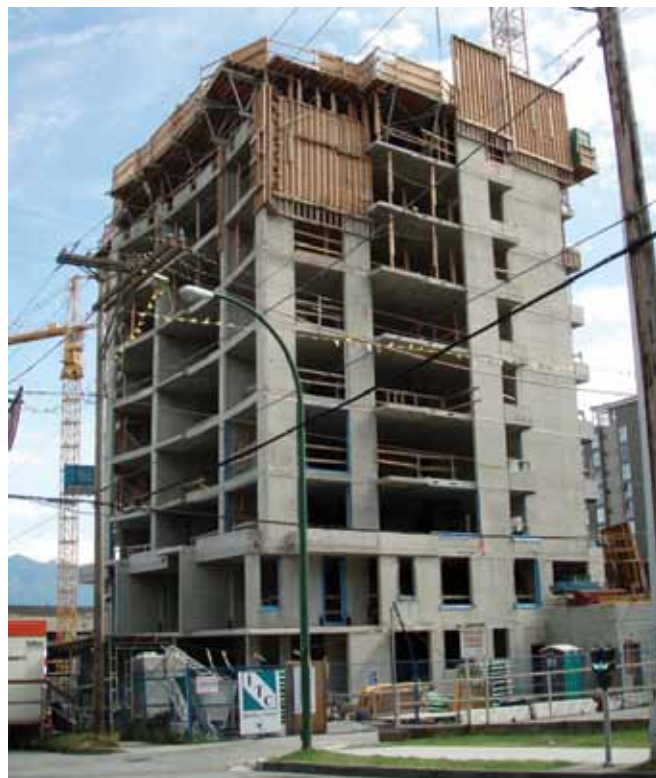
Panels are set in place on this high-rise to create one-sided backstop forms to gun shotcrete against
