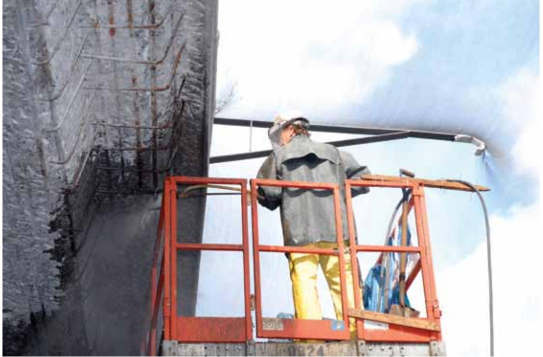
Fig. 6: The nozzleman is battling the “wind-tunnel effect”
