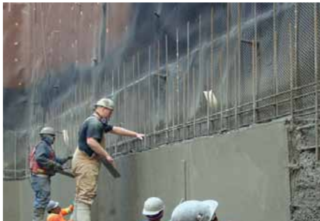
In many cases, when there is a structure or substrate to gun against, shotcrete can be gunned in place without the use of forms, eliminating forming costs altogether
