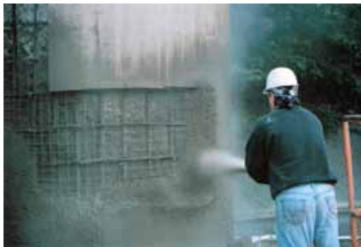
The dry process of shotcrete being gunned on a pier can provide a better bond without using bonding compounds. The nozzleman is filling in the corners first and working toward the middle of the repair area so he doesn't trap rebound in the corners
