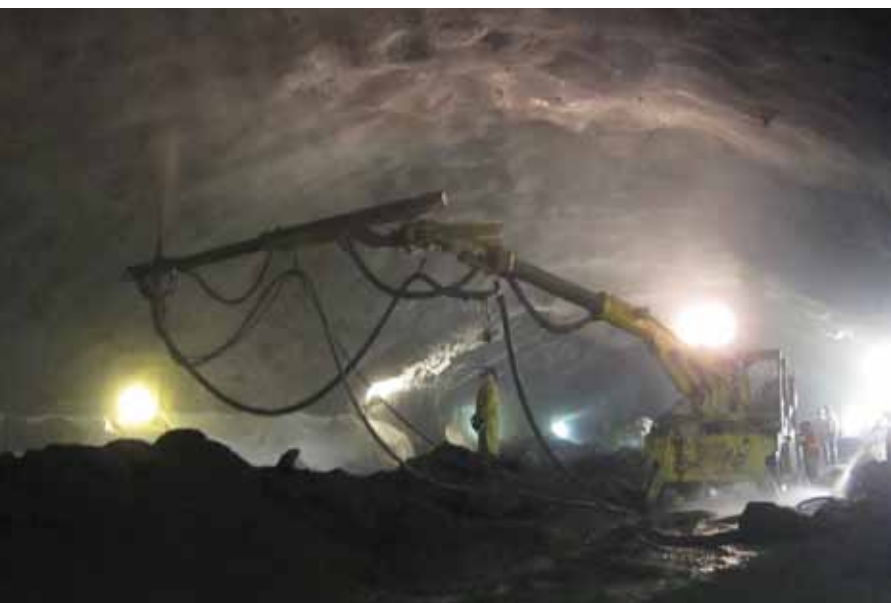
Modern transit projects require large caverns for stations. Shotcrete and modern shotcreting equipment make this possible
