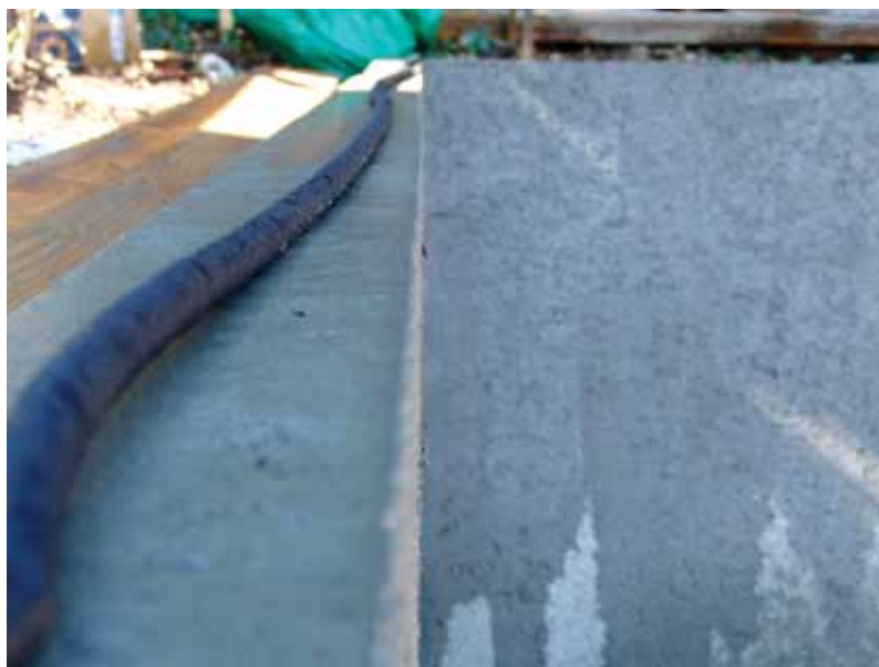
Fig. 2: A soaker hose can be useful in establishing saturated conditions prior to the application of an additional layer of shotcrete
