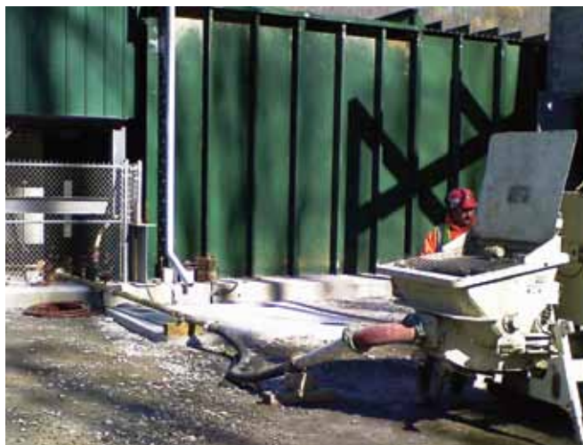
Pump with 3 in. (76.2 mm) pipe to shaft
