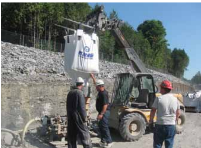
Fig. 4: The flexibility offered by preblended, bulk-bag materials also allowed the shotcrete crew to carry an inventory of shotcrete material on site
