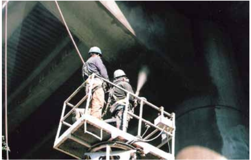
Overhead dry-process shotcrete being placed on the underside of a pier hammerhead in Pittsburgh, PA
