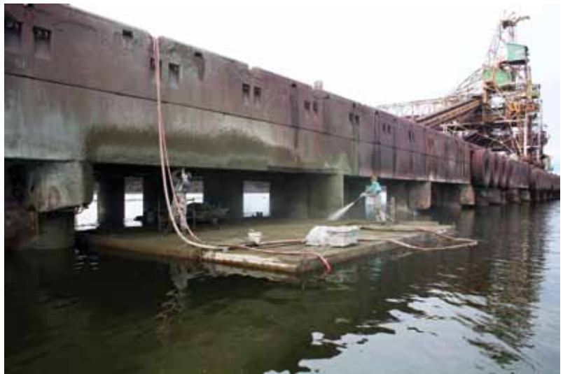
Barge platform supporting both a finisher and a nozzleman, working in tandem to complete the repair patch before moving to another area
