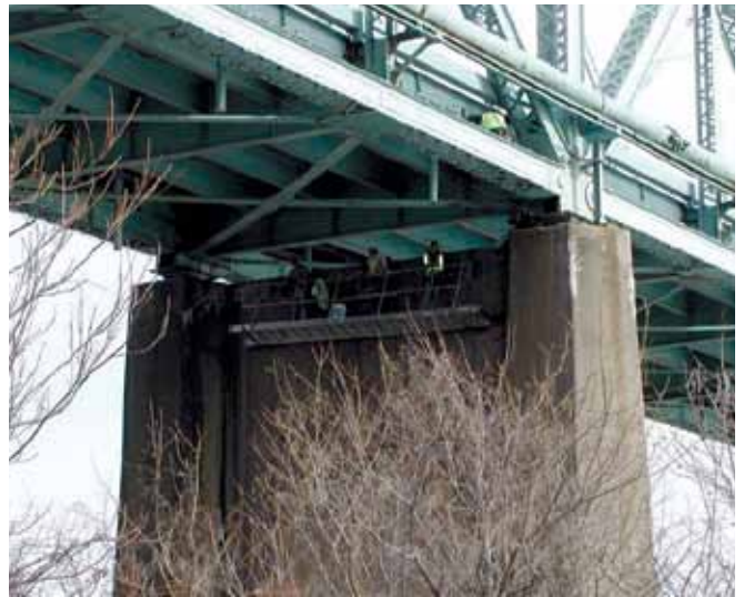
Rigging setup for access to bridge pier
