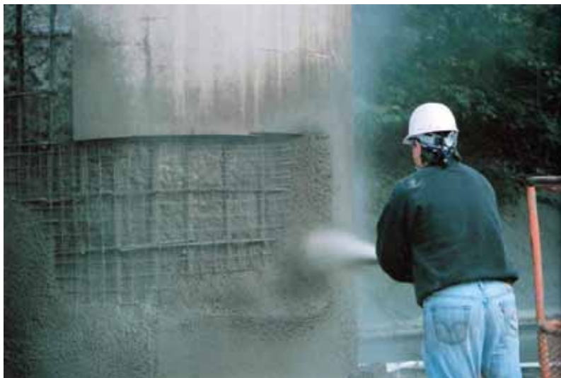
Nozzleman gunning dry-process shotcrete—filling the edges of the repair area first—and working toward the middle to avoid trapping rebound in the corners
