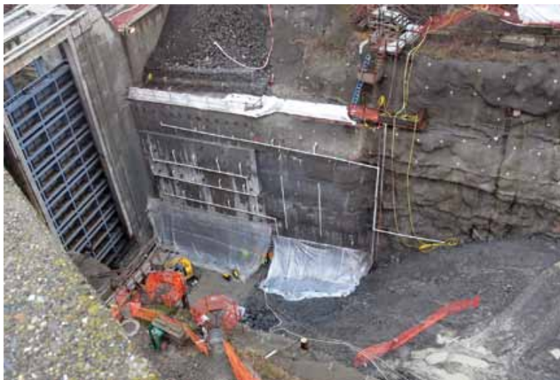
Phase I and Phase II jobs combined, as the shotcrete contractor finishes the bottom lift under the heat tent during Phase II
