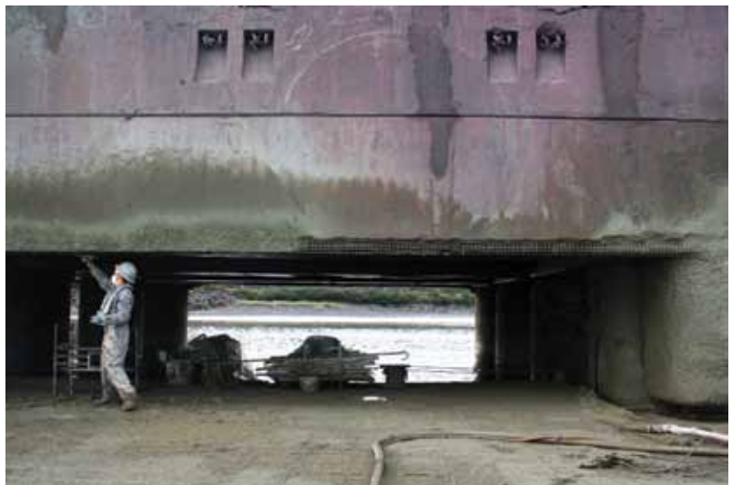
Concrete finisher creating an edge on the repair patch during high tide. The securely fastened metallic trellis can be seen in the uncompleted section
