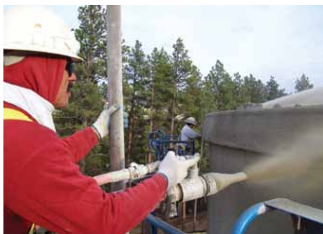
Fig. 9: Shotcreting dome ring
