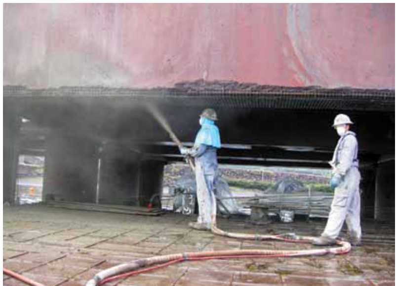
Nozzleman applying the initial coat of shotcrete to a repair 3 to 6 in. (75 to 150 mm) deep using the dry-mix process during high tide
