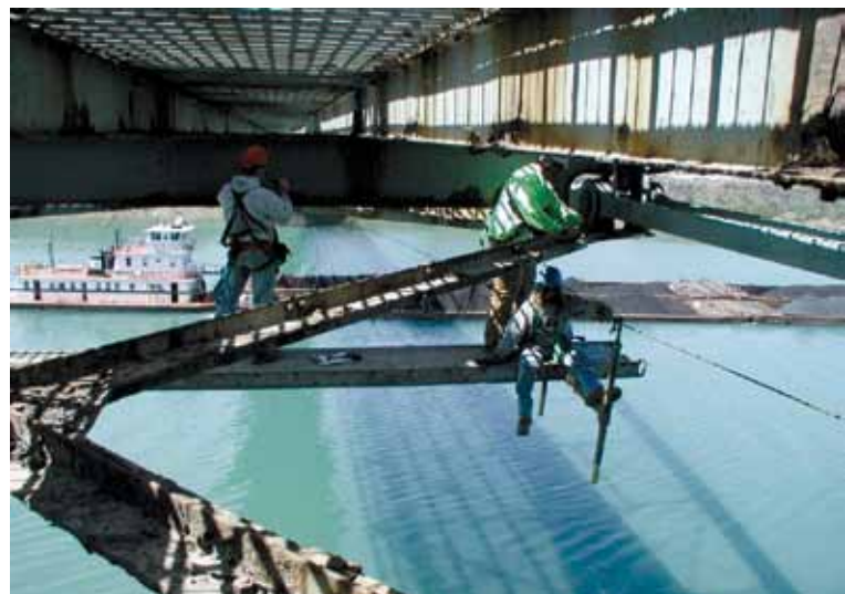
Cable rigging under bridge super-structure
