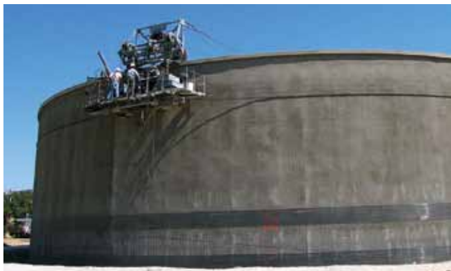
Fig. 2: Wrapping prestressing wire on circular prestressed tank Photo courtesy of Preload Company
