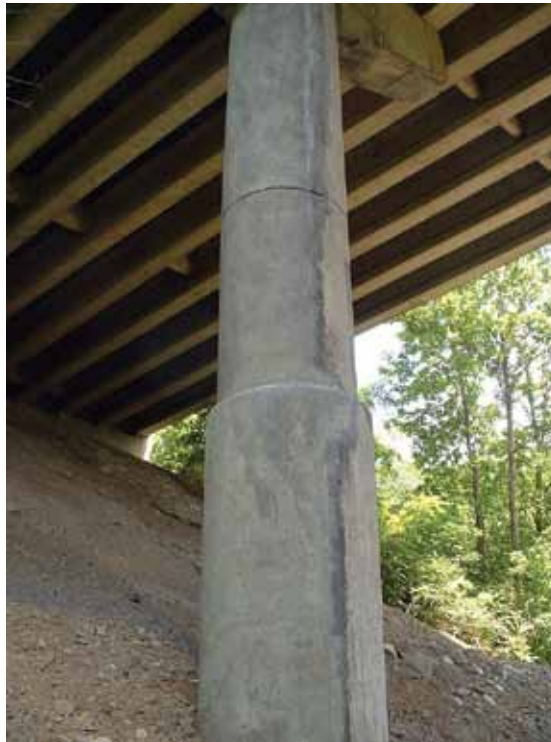
Shotcrete easily conforms to the circumference of this round bridge pier and works well with irregular shapes and configurations
