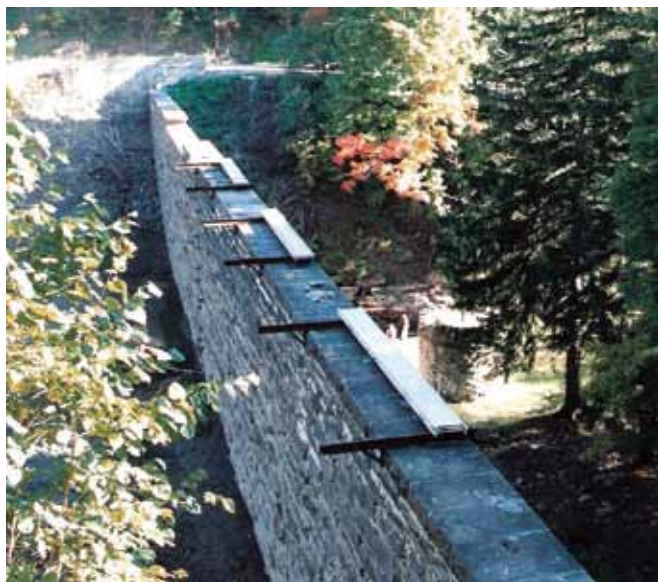
Outriggers in place across the top of a dam with stages positioned to be rigged
