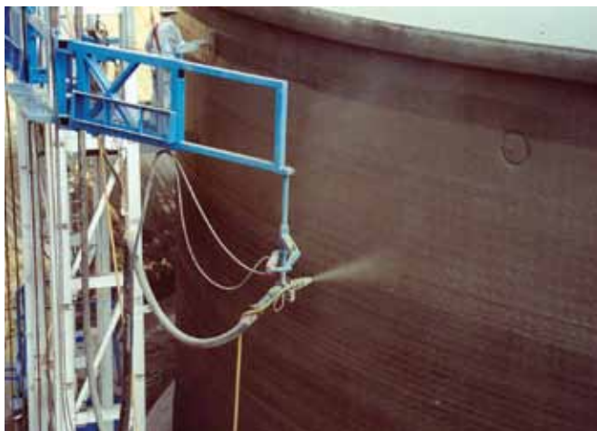
Fig. 6: Remotely operated nozzle on automated wrapping/shotcreting machine
