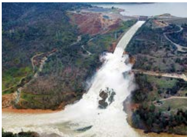
Fig. 1: February 2017 Oroville Dam main spillway is damaged
