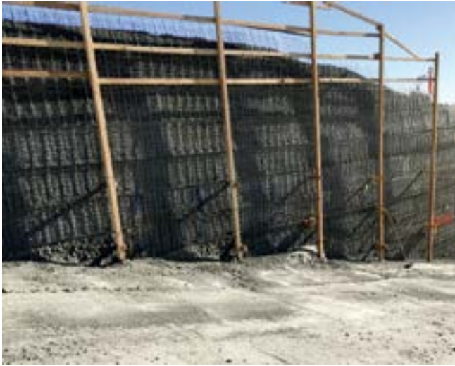
Fig. 5: Shotcrete substrate of RCC berm and WWF reinforcing
