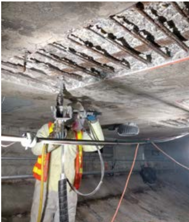
Fig. 5: Working in the air ducts provided for tight work spaces for the entire crew. Cruz devised methods to ease human comfort while working in these situations. Crew chipping away deteriorated concrete (Photo courtesy of Cruz)
