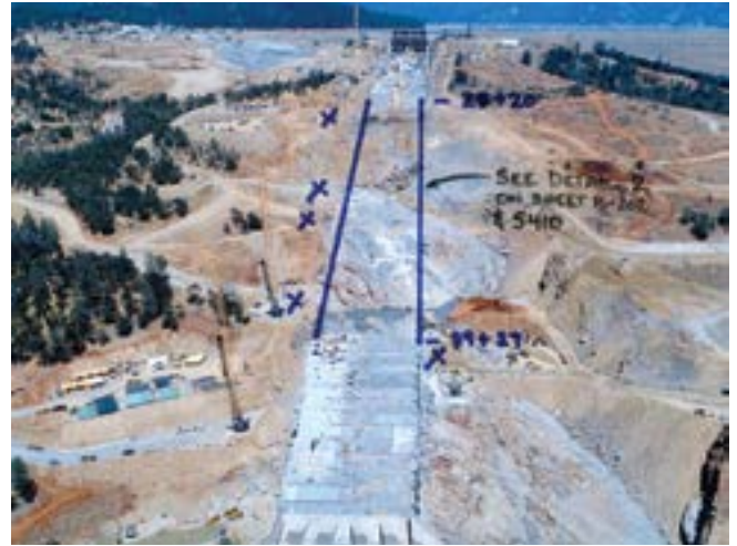
Fig. 6: Deep trench in middle third of main spillway chute, temporary shotcrete walls
