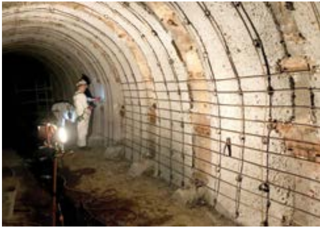
Fig. 3: Installing second mat of steel
