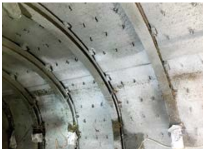
Fig. 1: Installing first shotcrete layer
