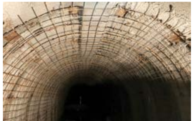
Fig. 6: Second mat of steel installed
