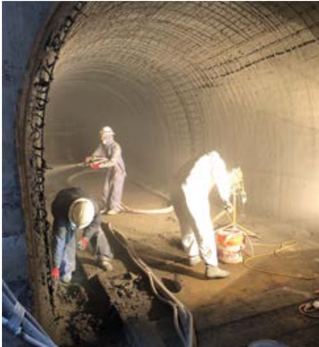
Fig. 7: Placement of second layer of shotcrete
