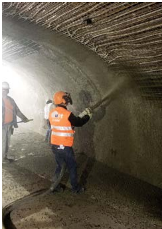
Fig. 2: MAPEI's UTT products have commercial as well as industrial applications. Its additive technology was added to shotcrete to create the walls of this high-tech wine cave
