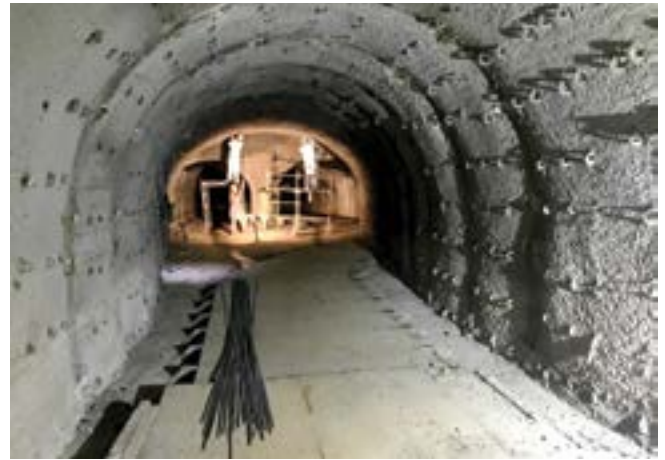
Fig. 4: Single bore prepared to receive second mat of steel
