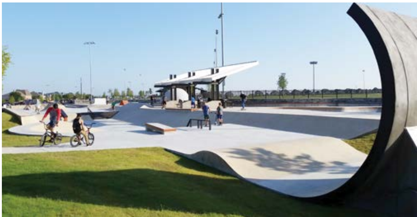
Fig. 4: Over-vertical, cantilevered concrete wave feature in foreground
