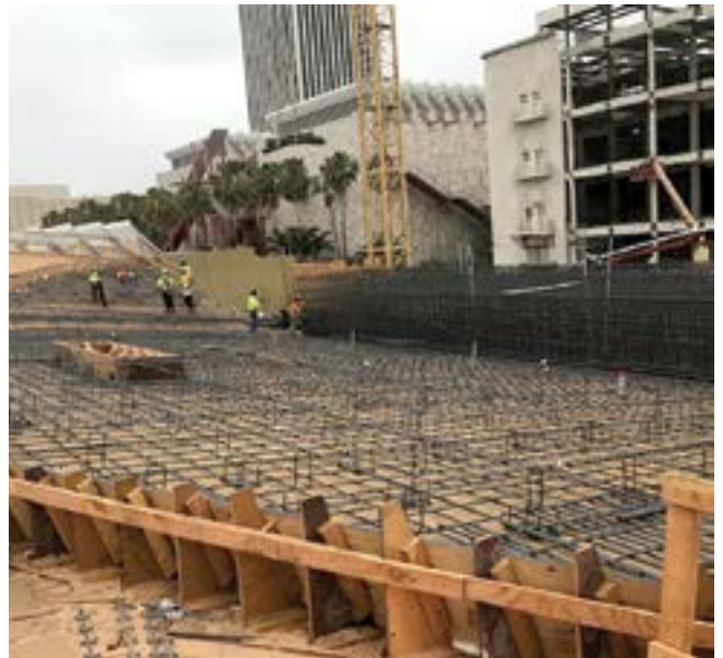
Fig. 5: Superior Gunitite preparing to shoot the wing slabs
