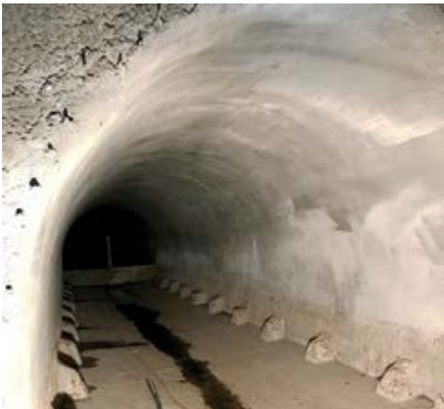
Fig. 10: One barrel of double barrel section completed
