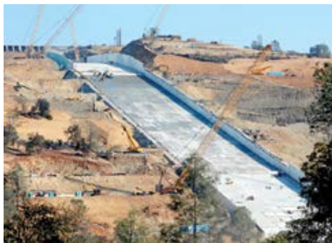
Fig. 2: Middle third of the 3000 ft (900 m) main spillway chute
