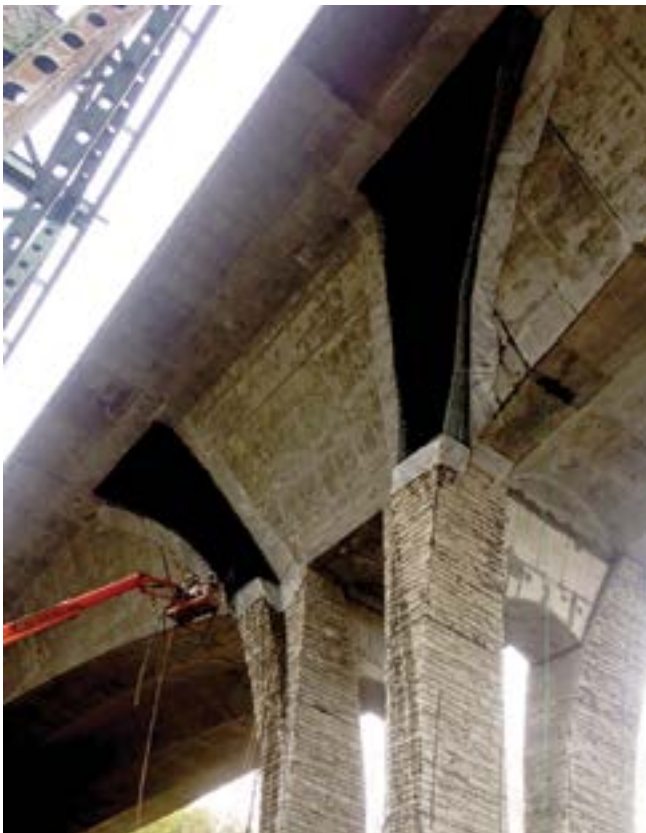
Fig. 1: Two fins at the northern pier prior to being shot. Reinforcing bar and stayform
