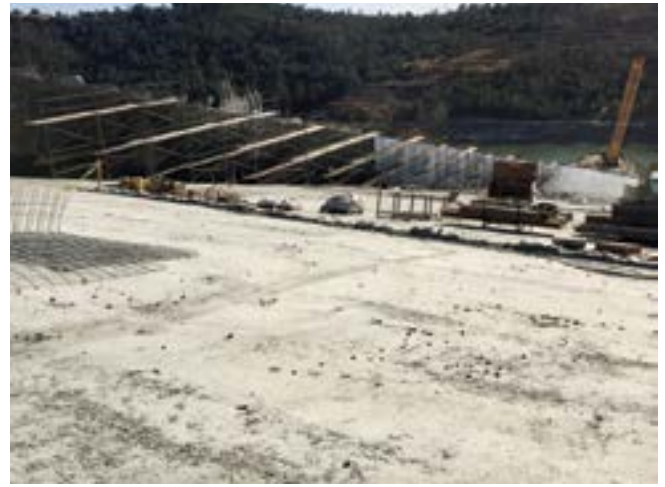
Fig. 4: Staggered and tiered work platforms on 25% slope
