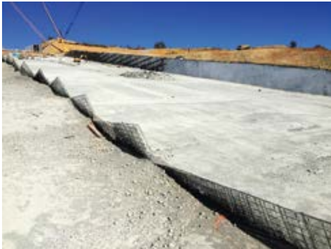
Fig. 3: RCC berm supporting main spillway walls
