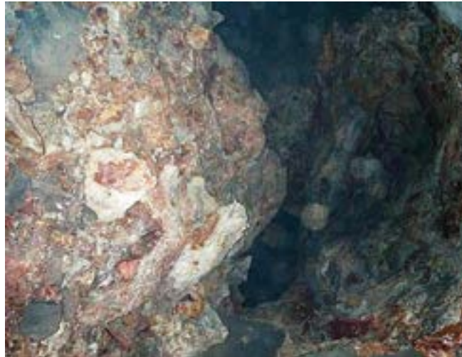
Fig. 4: Very-thin shotcrete caused a mine collapse
