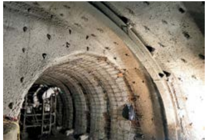
Fig. 5: First layer of shotcrete installed with preexisting support bents still in place
