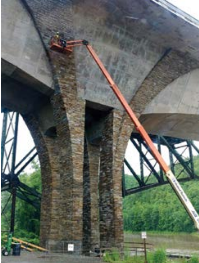
Fig. 8: Staining the piers
