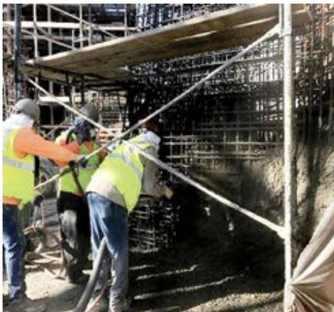
Fig. 1: Superior Gunite on site shooting the mockup
