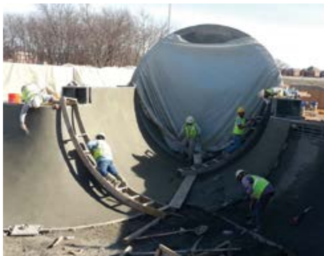
Fig. 5: Second (final) concrete layer with Class A steel-trowelled finish. Over-vertical concrete capsule protected from overspray
