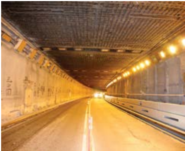
Fig. 2: Preconstruction, highlighting the light trenches ready for wet-mix shotcrete (top left), hollow wall niches (right wall) and exposed ceiling for patch repair (Photo courtesy of Judlau)
