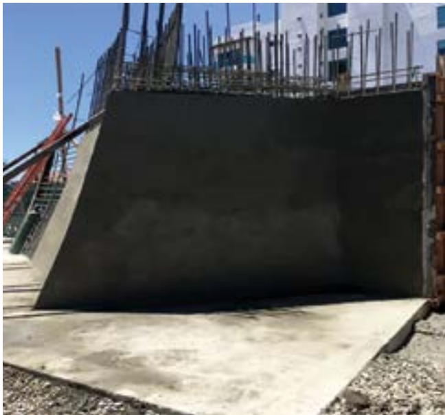
Fig. 4: Trapezoidal columns shot by Superior Gunitite
