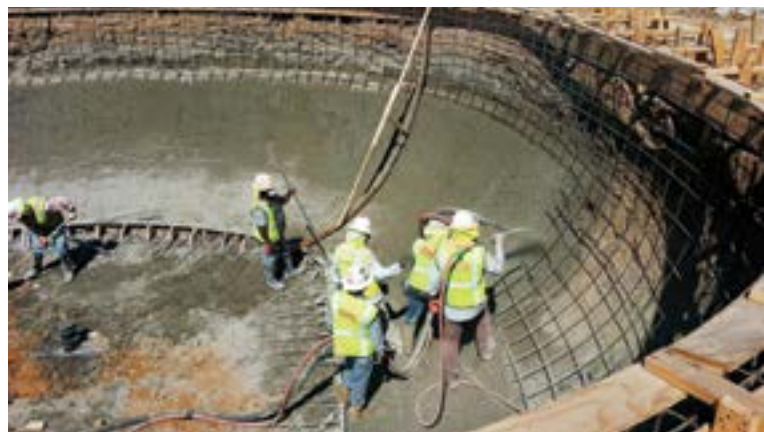
Fig. 3: Proper shotcrete preparation, crew positioning, and concrete placement. An initial layer placed early in the project assures protection of the compacted subgrade from damage due to adverse weather
