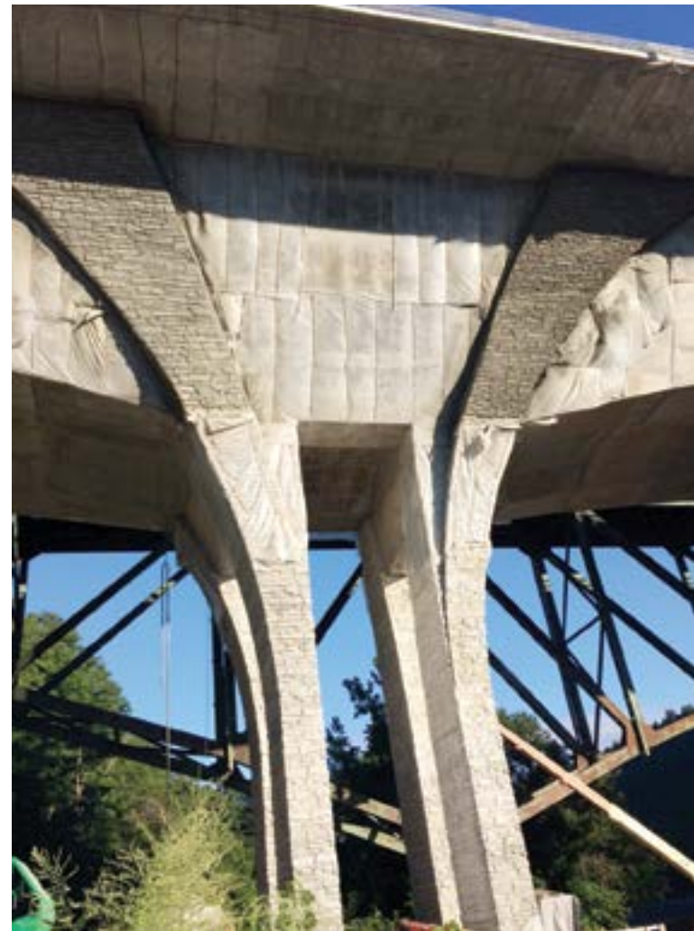
Fig. 7: Finished fins. Darker material is shotcrete, lighter is precast panels
