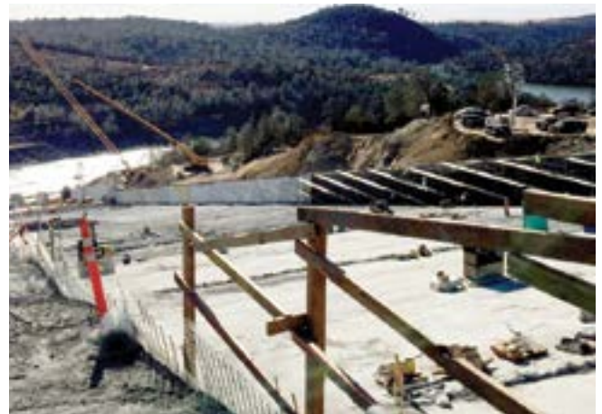
Fig. 7: View looking down spillway chute at temporary shotcrete walls
