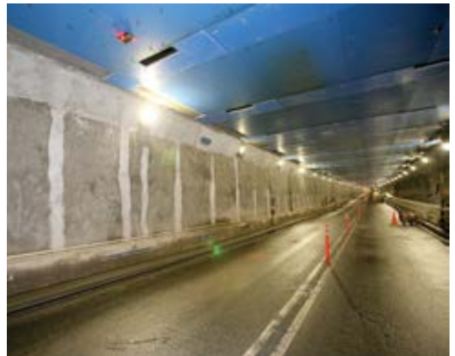
Fig. 4: Post-construction image of shotcrete, light trenches have been repaired (top left), the drainage chases have been chipped out and replaced (vertical lines) and ceiling has been patched and encased with fireproof panels (Photo courtesy of Judlau)
