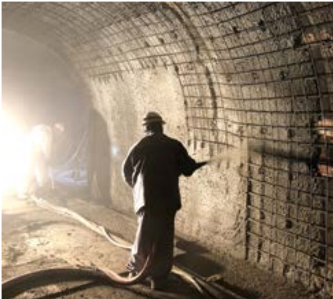
Fig. 9: Placement of second layer of shotcrete
