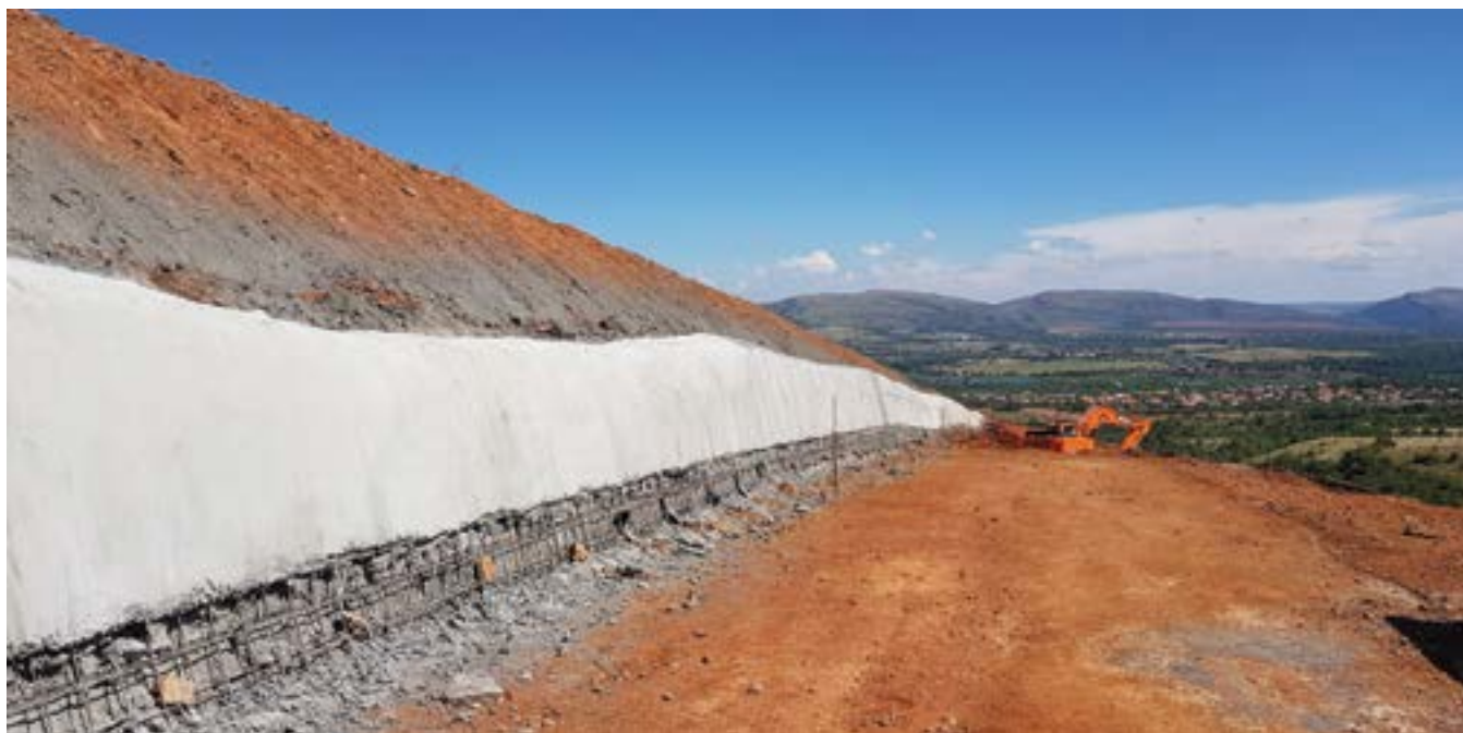
Fig. 1: Shotcrete finish—woodfloated and brushed
