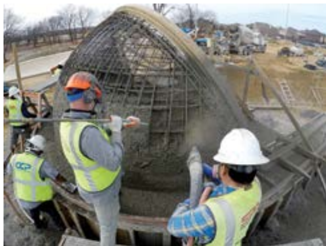
Fig. 6: ACI Certified Nozzleman and blow pipe operator. Stucco lathe placed between reinforcement curtains. Shotcrete pump and equipment in background
