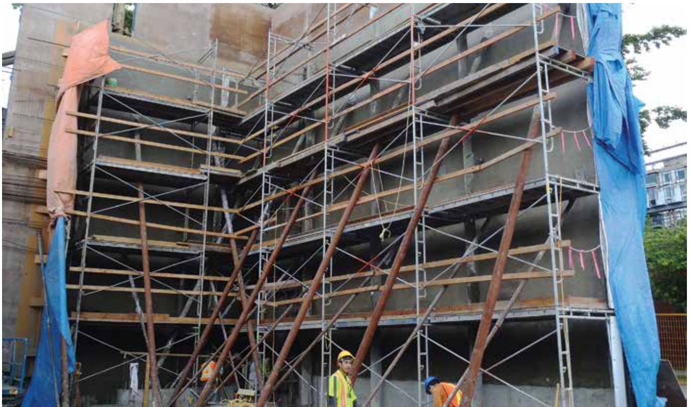
Fig. 8: Tall shoot panels braced from the shot side due to property line constrictions
