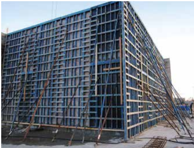
Fig. 7: Tall, light one-sided shoot panels with pinwheeled corners and uneven base; not possible with form and pour
