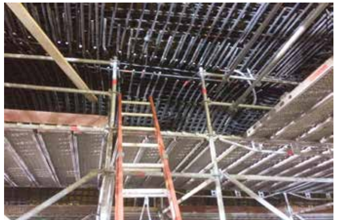
Fig. 4: Tunnel and cross-passage intersection arch reinforcing bar upper-level arch of TT#1 structure
