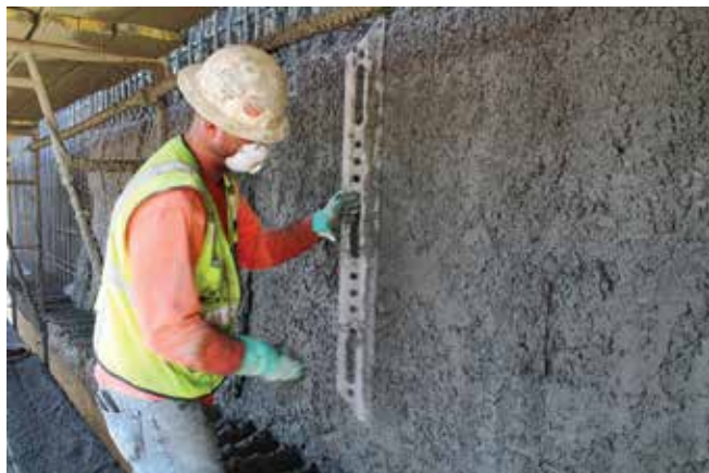
Fig. 5: Rod, float, and trowel work to tolerance wall thickness to ground wires
