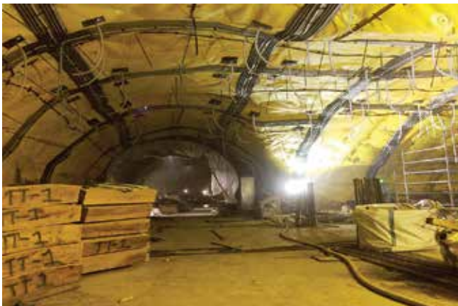
Fig. 2: Waterproofing membrane installed after build back and smoothing has been completed in the upper-level arch of TT#1 structure
