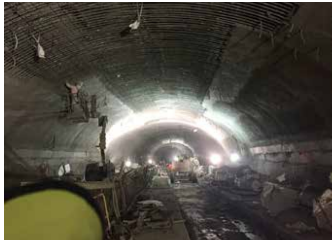
Fig. 10: Installation of GCT 1/2 arch with rod finish, working from boom lifts
