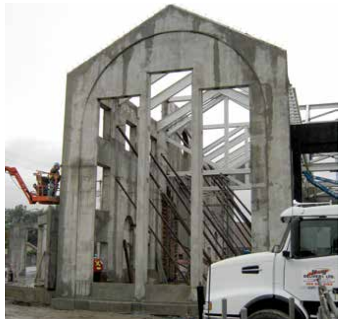
Fig. 6: Finished shotcrete structure using only one-sided shoot panels, eliminating the risk of voids in the slender pillars that can occur when using form-and-pour
