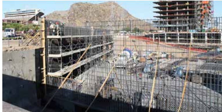
Fig. 2: Buesing Corp. setting ground (piano) wires from scaffolding (reinforcing bar curtain by concrete subcontractor)
