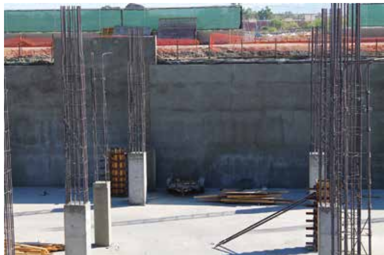
Fig. 7: Completed shotcrete finish walls in the background (CIP columns by concrete subcontractor in foreground)
