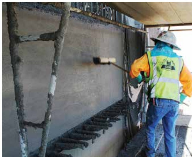
Fig. 6: Applying a light broom finish
