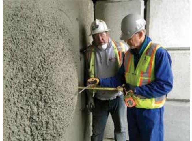
Fig. 7: Measuring thickness of natural fiber mixture (WNF) beehive
