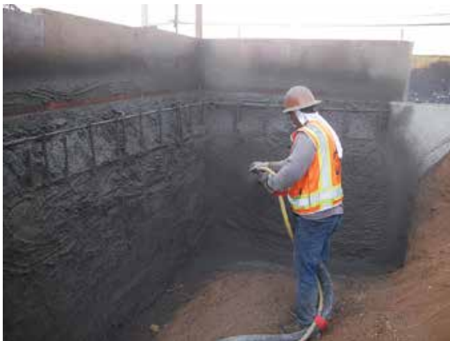
Fig. 15: Bench-gun shooting L-shaped wall
