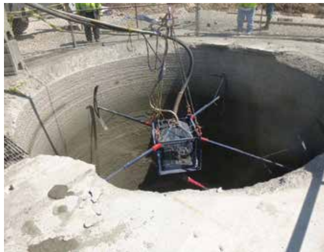
Fig. 3: Shaft lining with the spider
