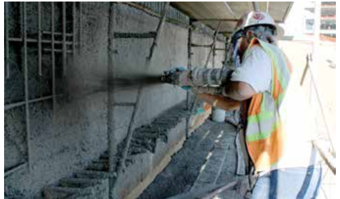
Fig. 3: Nozzleman shooting shotcrete (wet-mix) for structural finish wall
