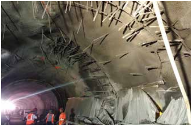
Fig. 1: Upper-level arch section of three-level structure TT#1. Overbreak reinforcement dowels and grade control wires
