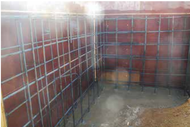
Fig. 14: Formwork and reinforcing bar for L-shaped wall
