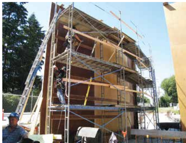
Fig. 2: Architectural reveals and recessed panels on single reskinned shoot panels for curved wall prior to reinforcing bar placement
