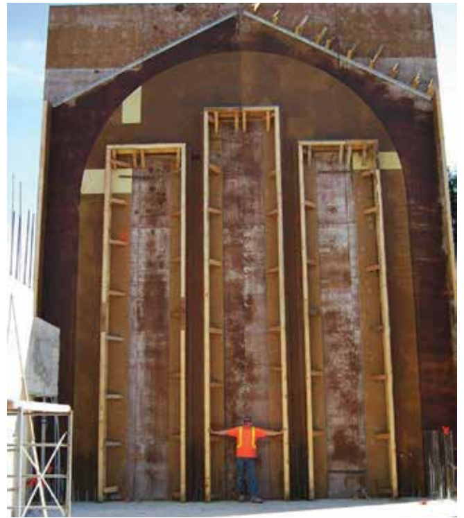
Fig. 5: Complex shoot panel formwork for a church; notice the lack of internal bracing required in the window breakout
