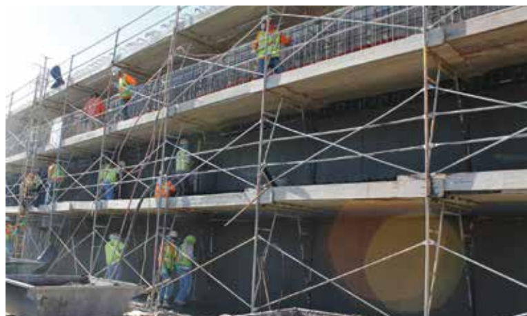
Fig. 4: Multiple shotcrete activities on three levels of scaffolding
