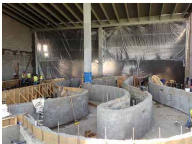
Fig. 1: First section of lazy river placed
