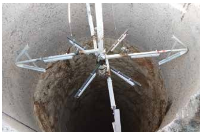
Fig. 1: Positioning and ready to begin the video. Note the bars of lights so we can get a very clear picture of what the shaft looks like
