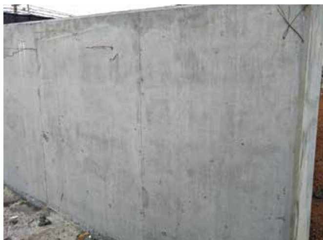
Fig. 18: Stripped face of L-shaped wall is defect-free
