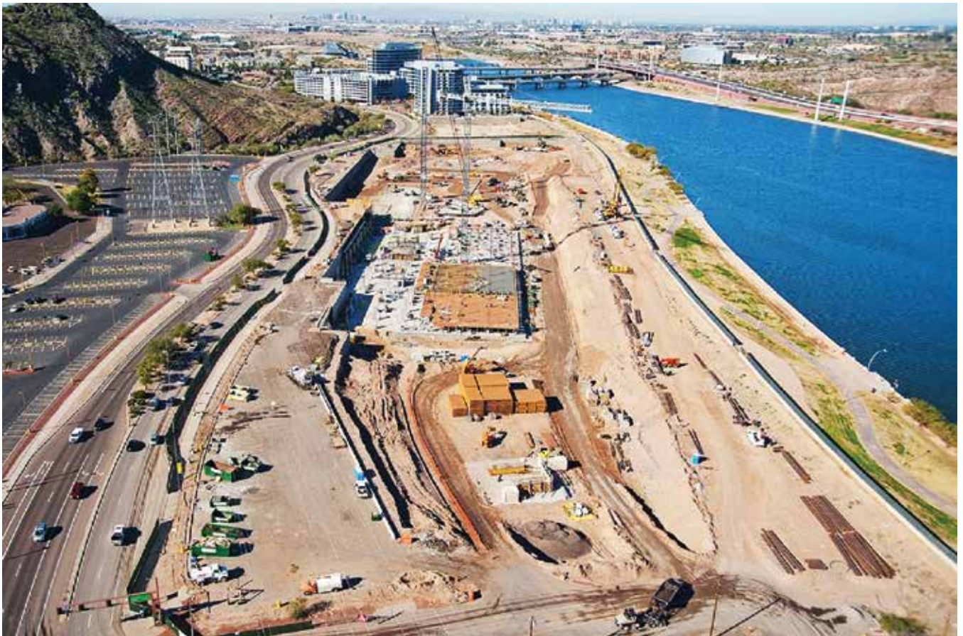
Fig. 1: Aerial view of Buesing Corp.'s mass excavation, shoring, and shotcrete finish wall work in progress
