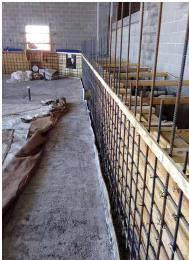
Fig. 3: Leisure pool ready for shotcrete application
