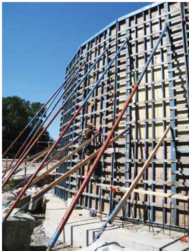
Fig. 1: Tall segmented radius, one-sided "shoot panels" for curved wall forming
