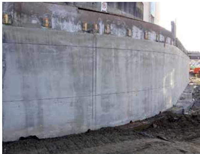
Fig. 9: Finish troweled curved wall, with post saw-cut architectural reveals
