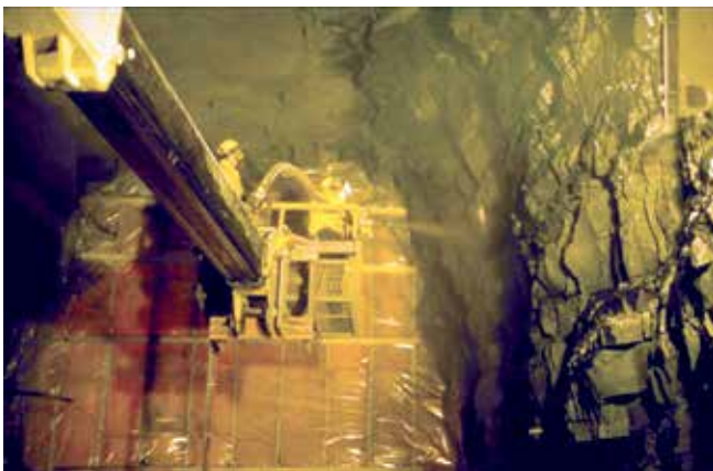
Fig. 6: Hand application of dry-mix shotcrete in a tunnel in British Columbia, Canada, in the 1970s
