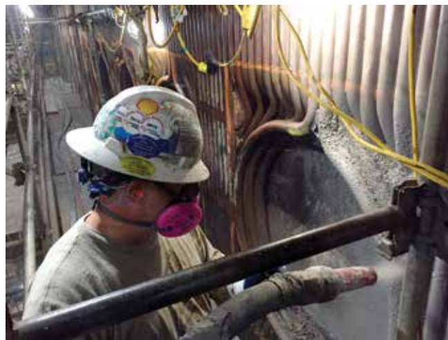
Gunning a high-temperature refractory with the dry-mix process in the burners of a coal-fired power plant. The refractory material did not use portland cement
