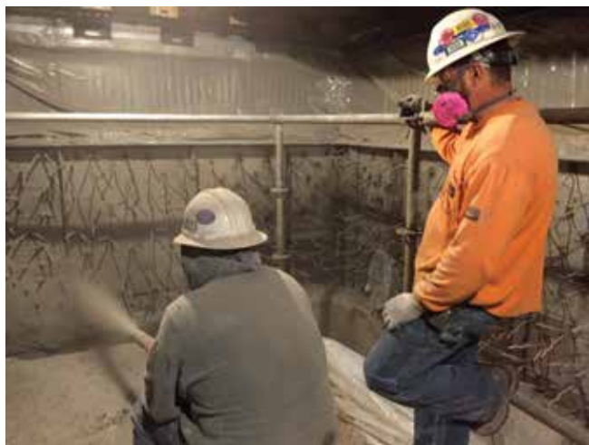
A 9 in. (225 mm) thick dry-mix process installation of high-strength 2600°F (1400°C) refractory in a power plant ash hopper
