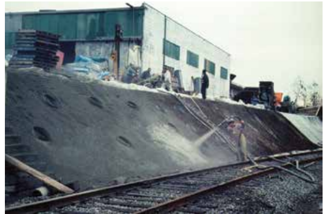
Fig. 4: Dry-mix steel FRS lining of a railway embankment in Burnaby, BC, Canada, in 1978
