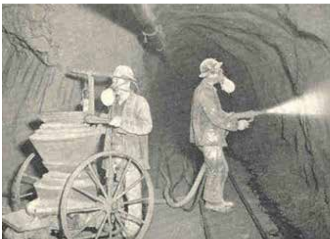
Fig. 2: Lining a tunnel with gunite using a double-chamber gun in the 1920s
