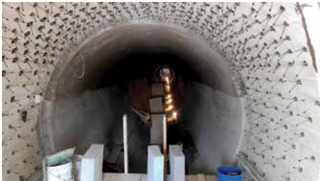
Refractory-lined 0.25 mile (0.4 km) long tunnel was placed with shotcrete
