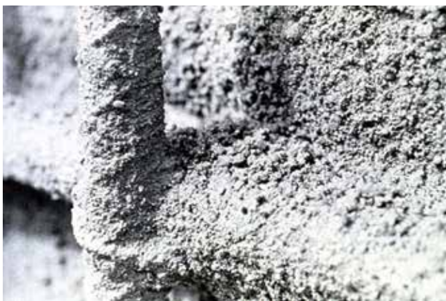
Fig. 2: Visual observation during shotcrete observation may note improper shooting techniques, resulting in inclusion of voids or rebound materials with low integrity where it matters most. Laboratory tests of panel cores do not address this issue, as it is related to shooting technique in this location. Visual examination for cracking patterns, supplemented by hammer sounding (ASTM C4580-12) to detect hollow/delaminated areas for closer study, and possible coring for laboratory testing where relevant properties can be determined
