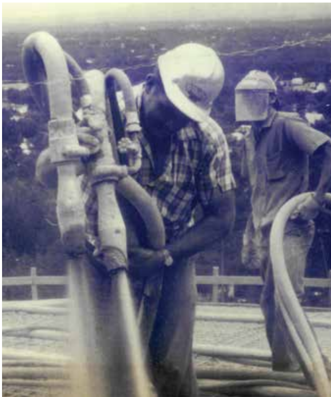
Fig. 2: Placing dry-mix shotcrete using dual nozzles to increase production when shooting a free span 3 in. (76 mm) thick dome circa 1965
