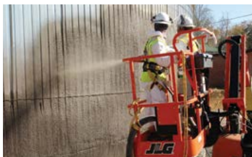
Fig. 4: Application of wet-mix shotcrete to steel shell diaphragm of prestressed concrete tank wall
