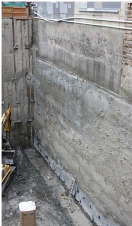
Fig. 2: 41 ft (12.5 m) deep shotcrete underpinning below the bottom of an existing building footing on the east elevation
