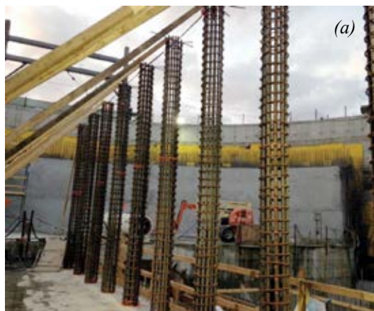
Fig. 2: Round columns. Most had: (a) a roof to wire and support; and (b) some did not
