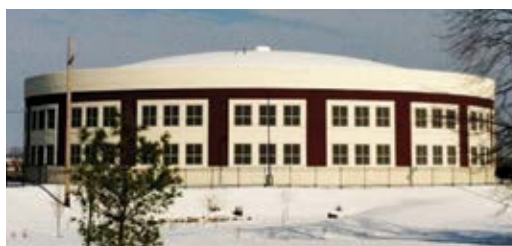
Fig. 3: 6.0MG wet weather storage tank built by Preload in 2013 for the Metropolitan St. Louis Sewer District and winner of numerous awards, including the 2014 ACEC Missouri Grand Award, the 2013 Keystone Award by the Associated General Contractors (AGC) of St. Louis, and the 2013 Quality Concrete Award by the Concrete Council of St. Louis
