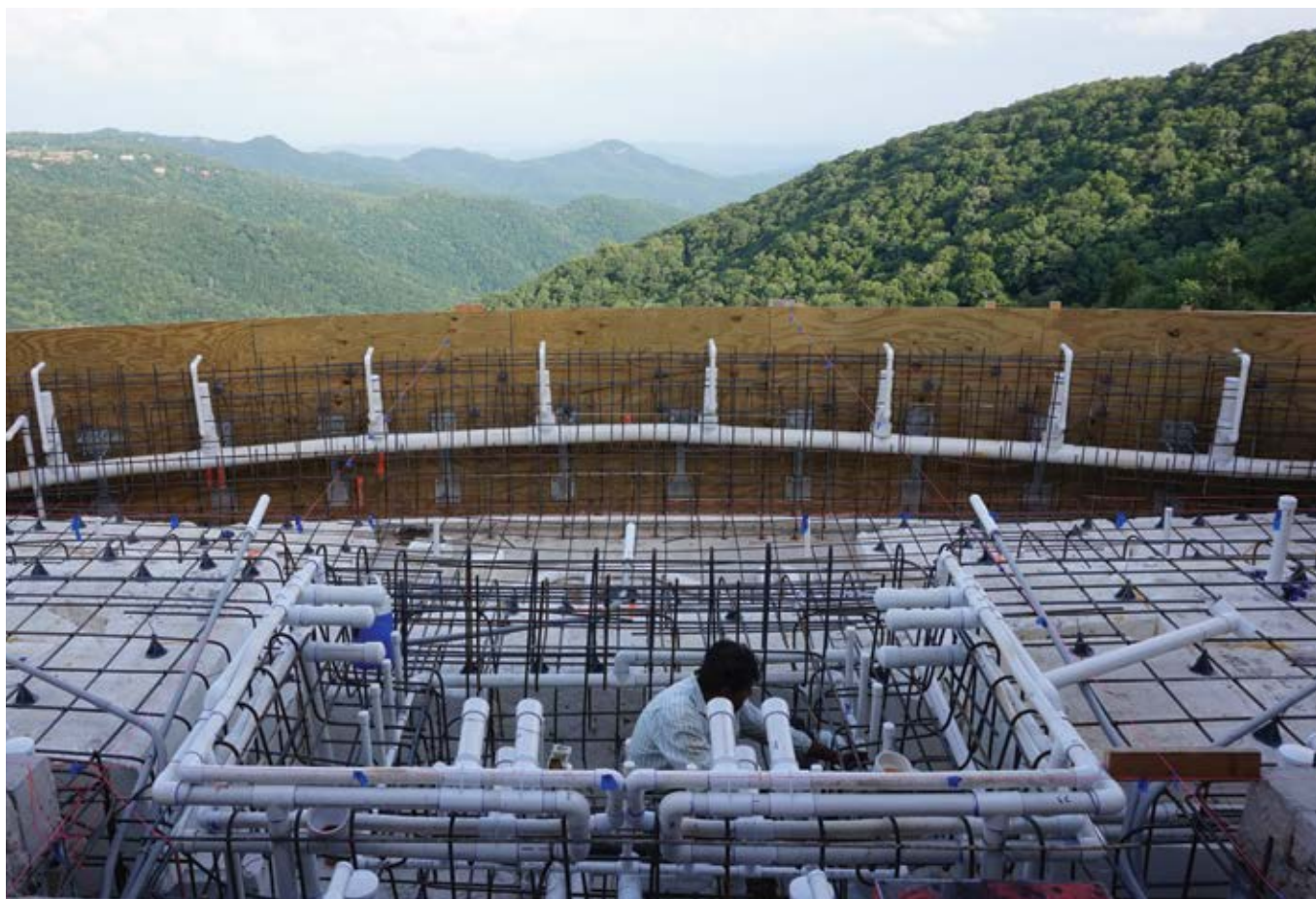
Fig. 3: Some of the intricate plumbing and steel work
