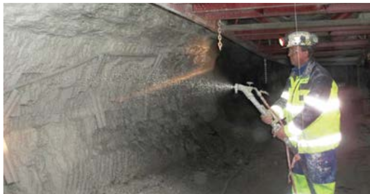
Fig. 4: Squeeze pump underground spraying
