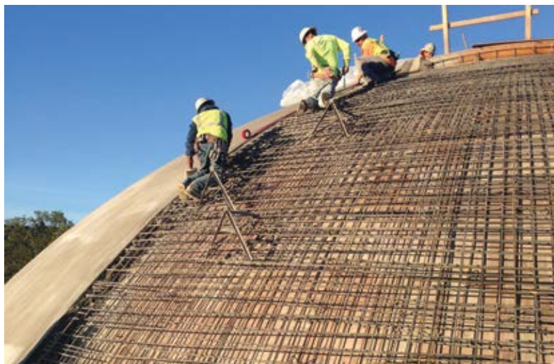
Fig. 3: Large dome shotcrete preparation
