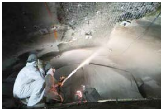
Fig. 5: Proof that dry-mix shotcrete, placed in a confined location, can be relatively dust-free by using a well-maintained dry shotcrete rig (with a pre-dampening unit and gun)
