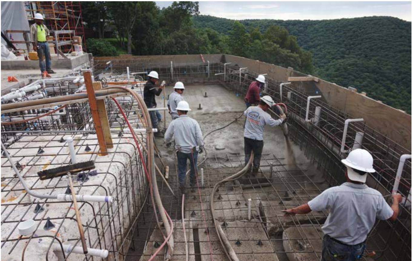
Fig. 5: The use of a blow wand, seen in the hands of the gentleman with the red shirt, is critical to maintaining quality throughout the project
