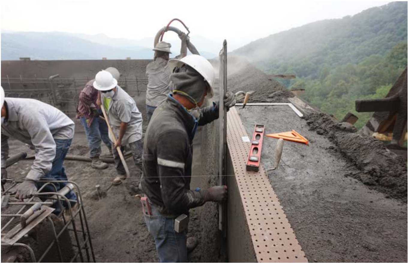
Fig. 1: Shooting the negative-edge trough while the finishers quickly work with the silica-fume-enhanced concrete and remove rebound and trimmings from the project
