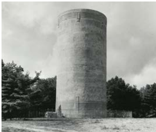
Fig. 1: Early prestressed shotcrete storage tank—circa 1936—in continuous maintenance-free service for more than 70 years
