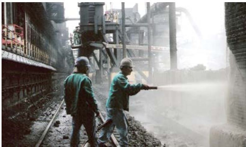
Fig. 4: During the shotcrete repairs to this coke plant quench tower, the railroad tracks are locked out with a derailer to prevent the use of the track while work is being done
