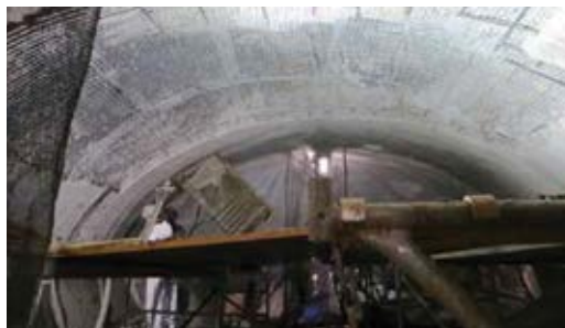
Fig. 2: The STM engineering team identified approximately 6540 ft 2 (600 m 2 ) of overhead area requiring removal and replacement, most of which ranged in thickness from 18 to 36 in. (450 to 900 mm)
