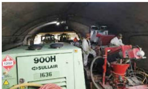
Fig. 3: Construction Interlag Inc. developed a system using two special flatbed train cars which were designed to carry all of the components, including the dry-mix shotcrete gun, pre-dampener, forklift, compressor, tool box, and enough bulk bags of shotcrete material to last the shift
