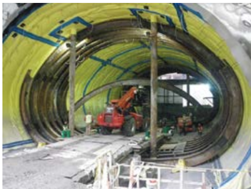
Fig. 4: Waterproofing and ring girders being installed
