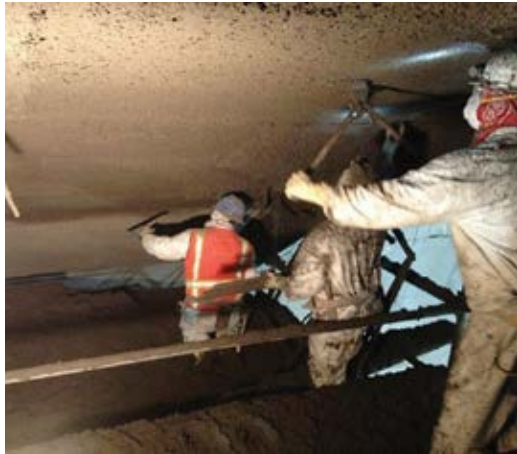
Fig. 8: Cutting of guides and finishing
