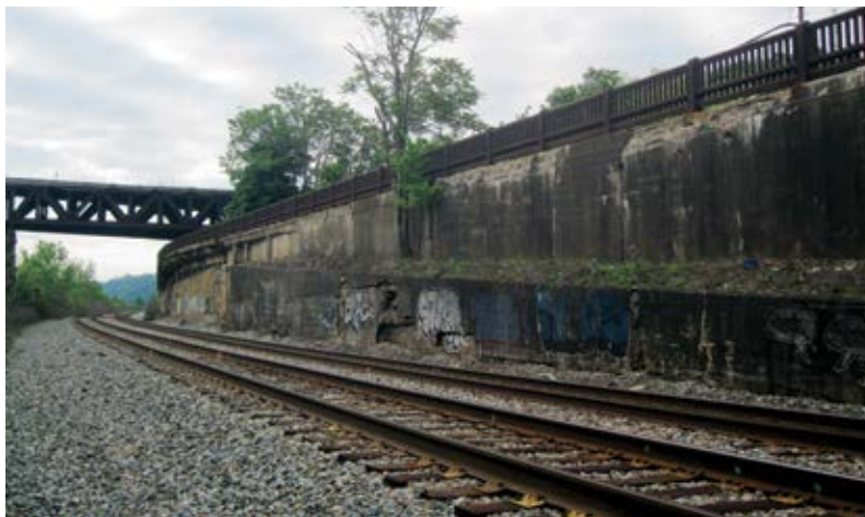
Fig. 2: In many cases, the shotcrete repair areas are close to the railroad tracks and special precautions have to be taken on active lines
