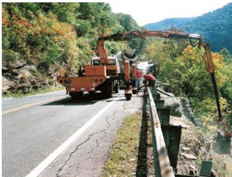
Fig. 1: A Snooper inspection crane being used for hillside access above railroad line during shotcrete placement
