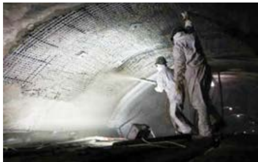
Fig. 1: The material specification called for a prepackaged, high-quality shotcrete mixture that would provide long-term durability
