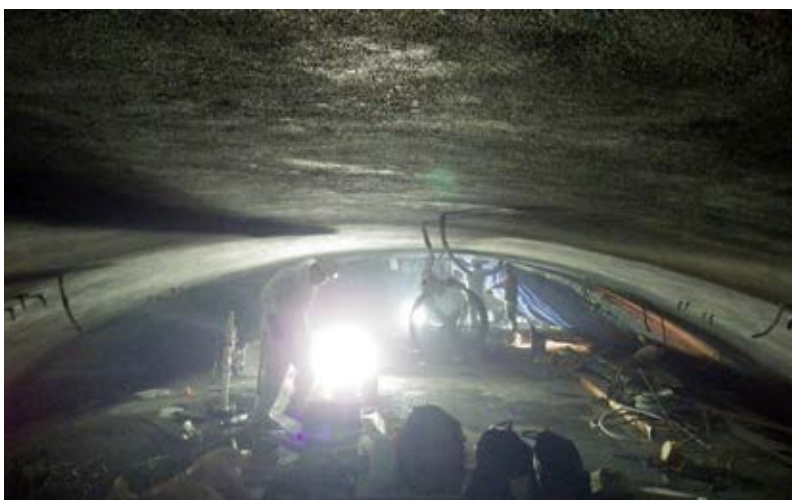
Fig. 3: Working on final panel—heat presented a challenge, requiring ventilation and close attention to curing
