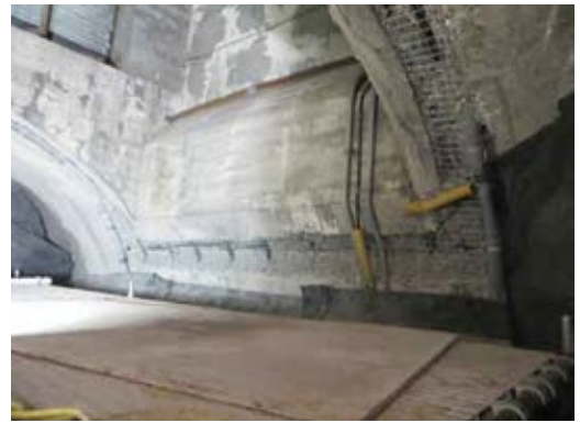
Fig. 4: Removal of deteriorated and delaminated concrete, installation of rock anchors and wire mesh, and ready for placement of dry-mix shotcrete
