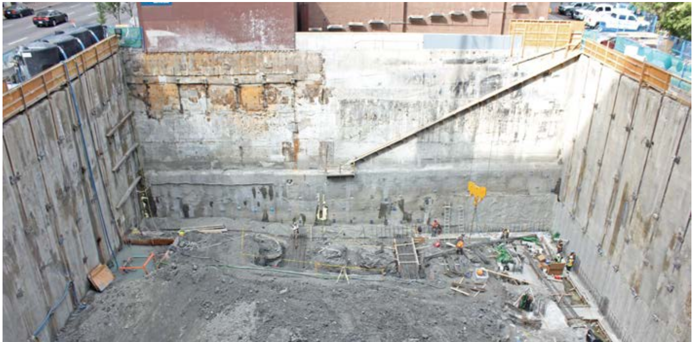
Fig. 1: 21.3 ft (6.5 m) deep shotcrete underpinning below an existing building footing on the west elevation at The Vogue, Calgary, AB, Canada
