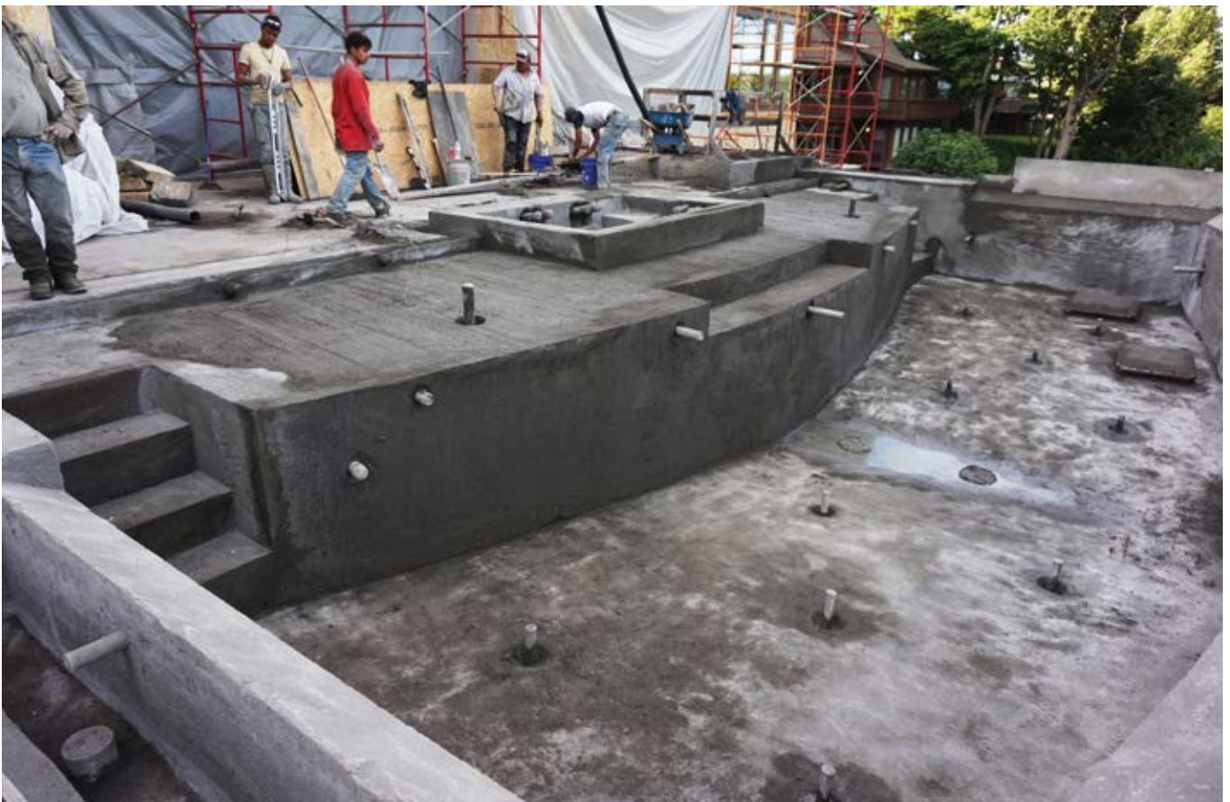
Fig. 2: The finished shell shortly after being shot
