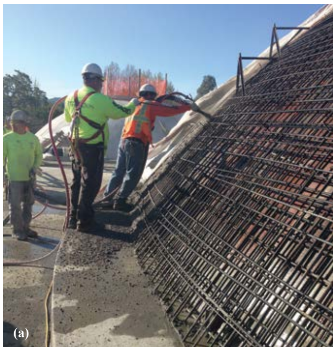
Fig. 2(a) and (b): Large dome shotcrete installation
