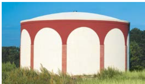
Fig. 2: Architectural treatment on top of shotcrete exterior for prestressed concrete ground storage tank, Fredrick, MD, 2009
