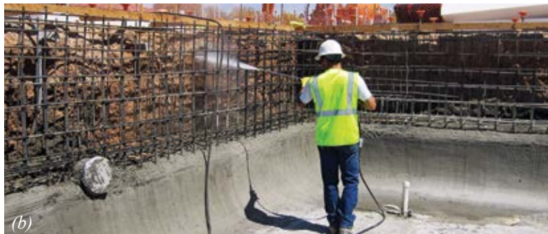
Fig. 8(a) and (b): Construction joints being prepared
