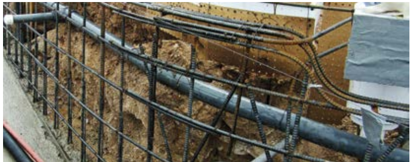
Fig. 6: When checking reinforcement, make sure the bars have proper clearance and cover. Reinforcing bars should be separated to meet the requirements of the project specifications and applicable local building codes. Stagger laps when possible to avoid bundling bars at contact laps, as seen at the top of the reinforcement in this image. Non-contact lap splices are preferred in shotcrete applications. Preconstruction shotcrete test panels may be required for contact laps that exceed No. 4 (No. 13M) reinforcement
