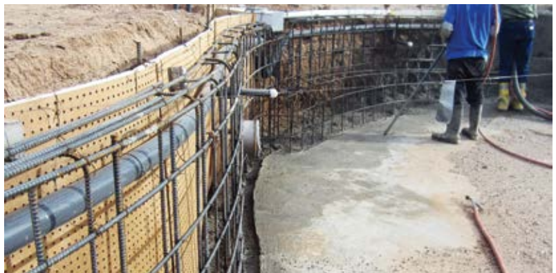
Fig. 7: Plumbing is a major component of most pools. Often, the plumbing components need to be placed in a way to allow for proper shotcrete placement. Enough room needs to be provided in the design for the plumbing, skimmer, lights, and reinforcing steel; pools take a lot of pre-planning with a qualified contractor and experienced crews
