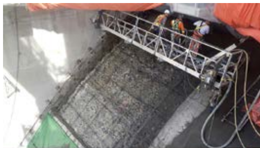
Hydro Dam Spillway Project. Spillway shotcrete resurfacing work had to be completed in three phases to maintain operation of the existing hydro facility
