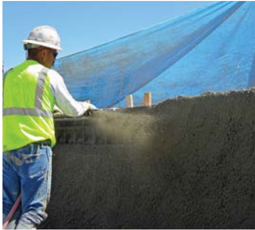
Fig. 4: Experienced ACI Certified Nozzleman shooting a beam—no cuttings will be reused in the structure. Also, note the blue tarp providing protection from overspray
