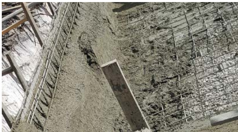
Fig. 1: A pool wall installed with wet-mix shotcrete before the pool floor has been placed. As a result, the pool floor is now contaminated with the rebound and cuttings from the shotcrete operation. This sloppy material sitting on the floor has not been vibrated or consolidated and must be considered as waste material and removed. Leaving this material in place would weaken the pool structure and significantly reduce the long-term durability of the pool shell. Unfortunately, incorporation of rebound and cuttings in the pool shell is the cause in 95% of swimming pool failures
