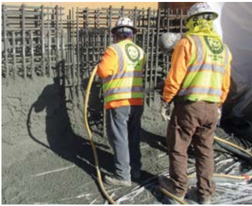
Fig. 2: Crew shooting preconstruction test panel
