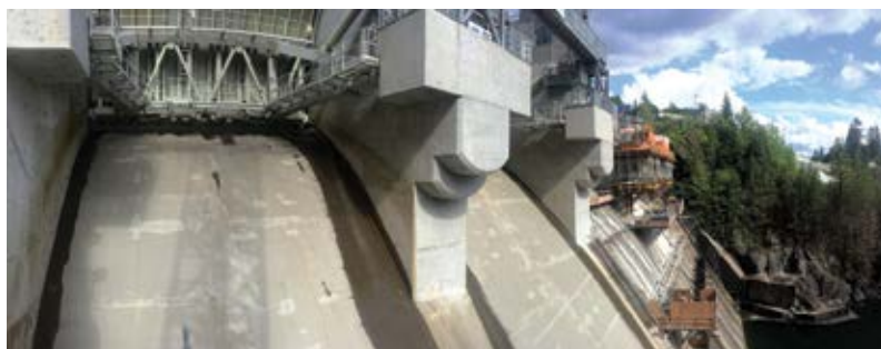
Hydro Dam Spillway Project. Spillway shotcrete resurfacing work had to be completed in three phases to maintain operation of the existing hydro facility
