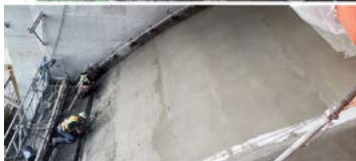
Hydro Dam Spillway Project. Spillway shotcrete resurfacing working off of a custom swing stage, before and after shotcrete
