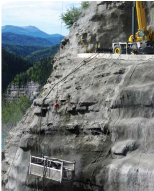
Northern British Columbia Hydro Dam. Spillway rock slope stabilization. Custom crane basket with wheels allowed the crew to stay in contact with the irregular rock profile while applying dry-mix shotcrete
