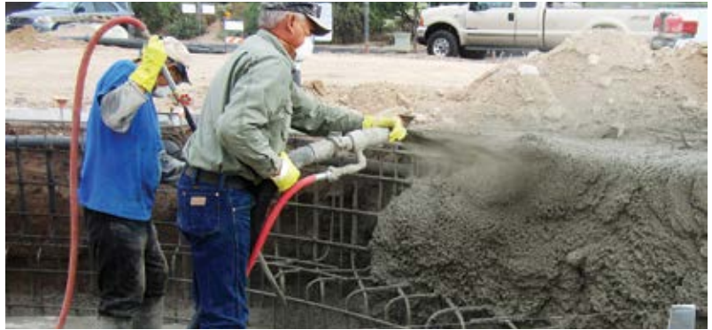
Fig. 5: ACI-certified nozzleman shooting walls with air-lance (blow pipe) tender cleaning the floor/wall joint before shotcreting so no rebound is used in the structure. Also, note the floor was completed first. The reinforcement at the bottom of the wall is for a bench that will be shot after the wall is complete. The contractor will need to clean all rebound and cuttings out from the bench area before shooting it
