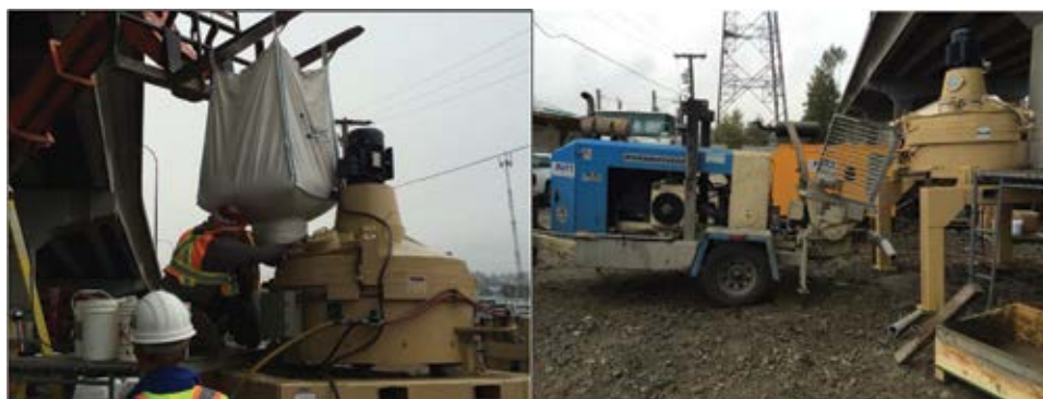
Fig. 1—Concrete pan mixer and wet-mix shotcrete pump (left) and after mixing, shotcrete was discharged into shotcrete pump (right).
