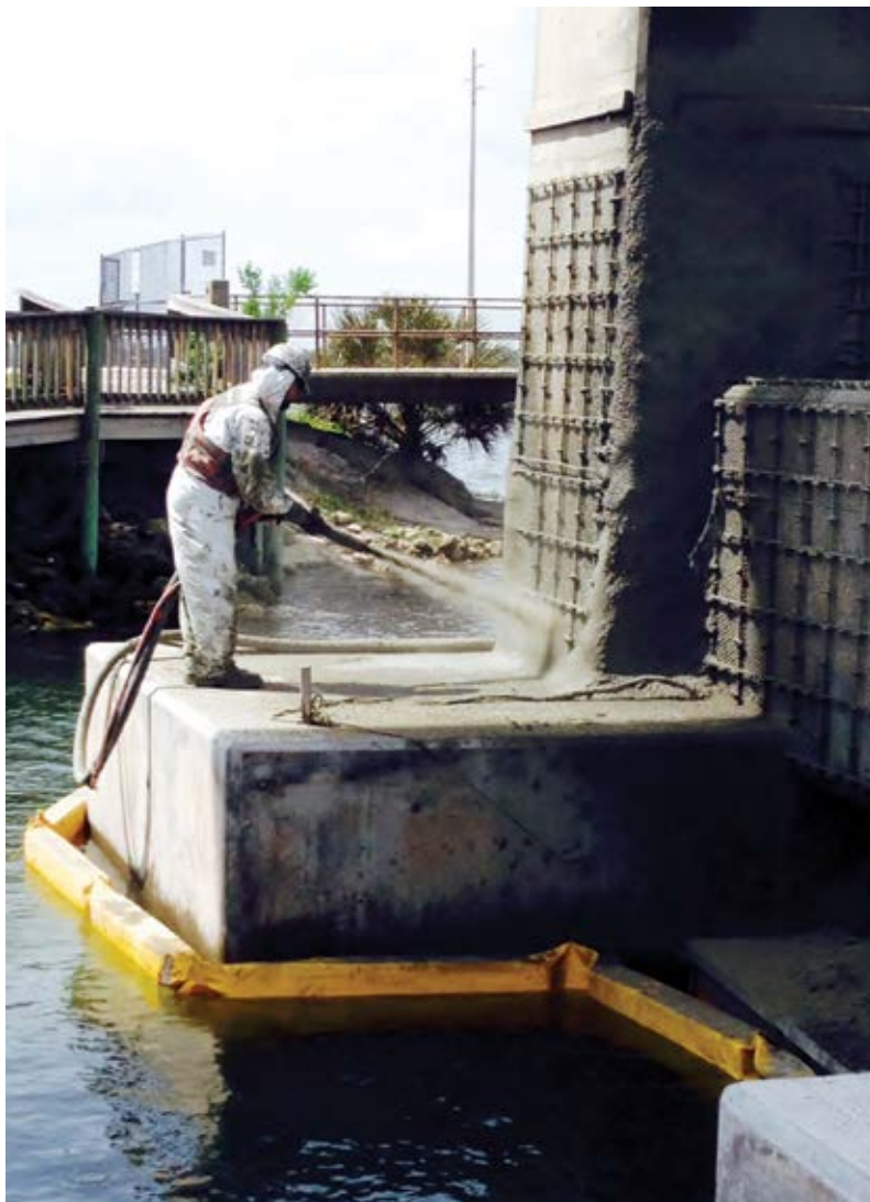
Fig. 2: Nozzleman shooting at a proper angle
