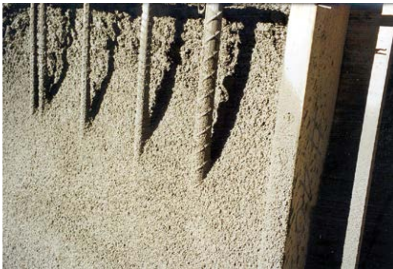
Fig. 3: Proper impact velocity and reinforcing bar encasement
