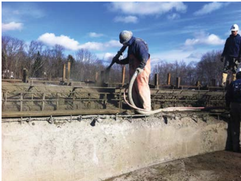
Fig. 1: ACI Certified Nozzleman applying wet-mix shotcrete
