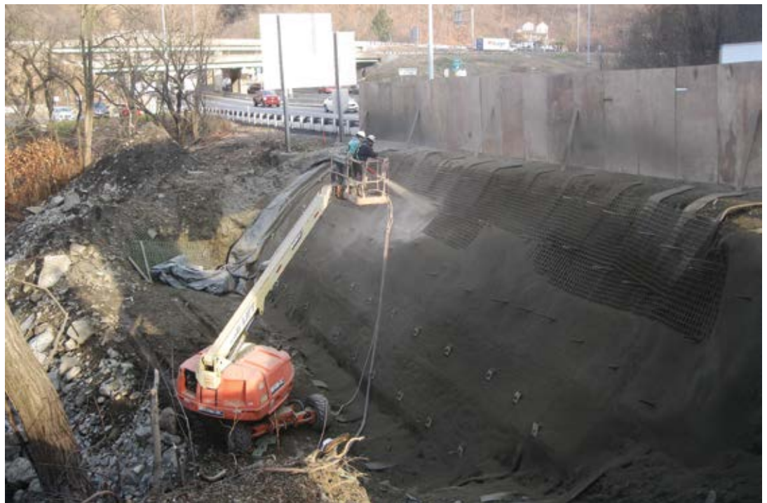
Fig. 1: Wooden barriers are installed in place along I-376 by the Fort Pitt Tunnel in Pittsburgh to protect traffic during the shotcrete placement of this soil nail wall
