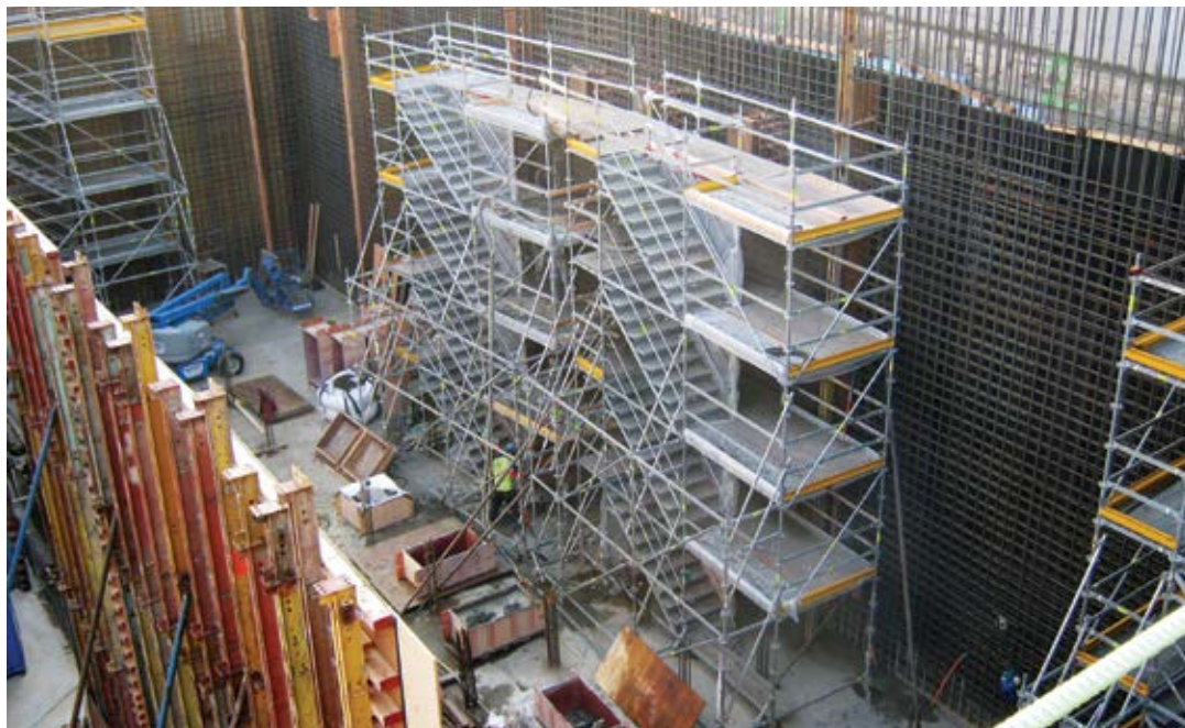
Fig. 2: Preparing to shotcrete the wall. The heavily congested reinforcing bar required for seismic reinforcement made application challenging. Photo courtesy Kryton International Inc.
