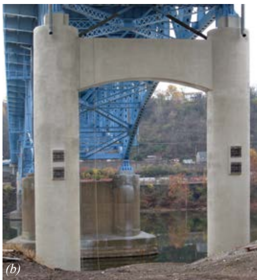
Fig. 1(a) and (b): Two large, round bridge piers being repaired and returned to their original contour using shotcrete
