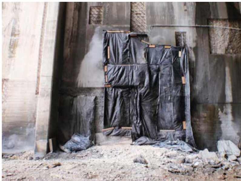
Fig. 3: Blankets and thermometers were placed on the concrete surface to monitor the temperatures through the cool night and curing period
