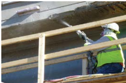
Fig. 2: Shotcrete repair under a bridge
