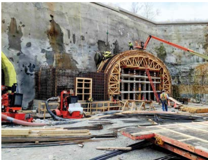
Fig. 8: Formwork for tunnel entrance
