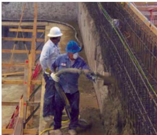
Fig. 3: Steady output with minimal surging makes for fatigue-free hose work thanks to the fast sequencing valve of the Schwing shotcrete pumps
