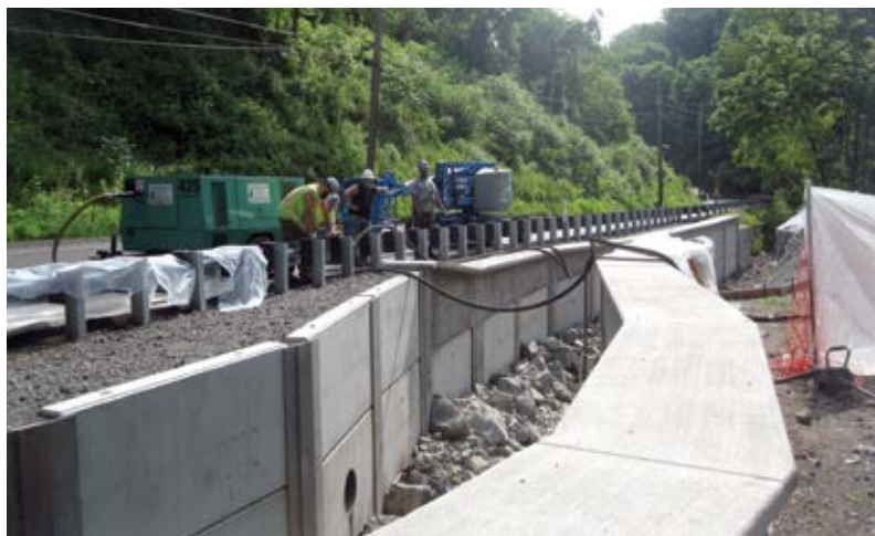
Fig. 4: On two-lane roads, when it is necessary to set up shotcrete operations on the roadway, a lane closure with advanced signing and flagmen becomes necessary
