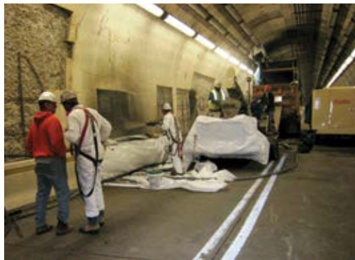
Fig. 2: Shotcrete being installed in the Liberty Tunnels by ACI Certified Nozzlemen using a predampener and a sufficiently sized air compressor. No damage to the tunnel was done by dust
