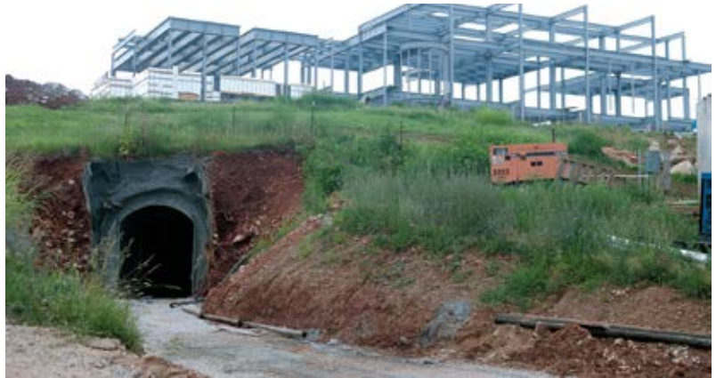
Fig. 3: Exterior portal leads to 150 ft (45 m) long tunnel and various chambers to create a wine cave 45 ft (14 m) under the owner's new home
