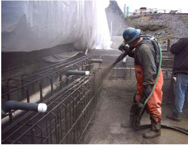
Fig. 3: Shotcrete sprayed at proper velocities results in compacted material with well-encapsulated steel reinforcing bar
