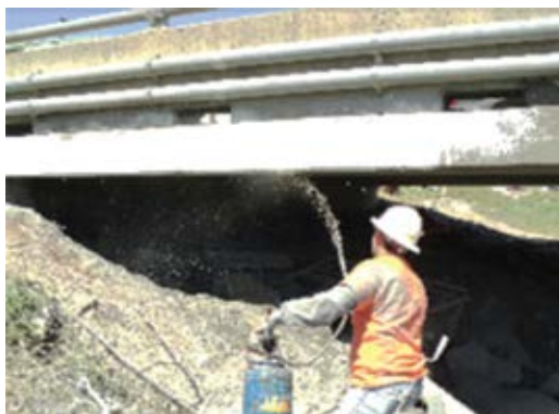
Fig. 3: Proper curing is a critical part of shotcrete placement
