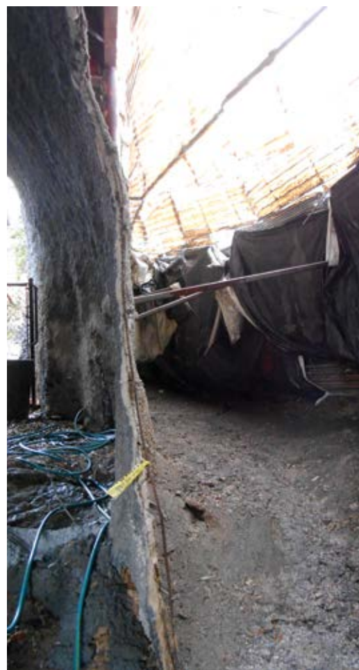
Fig. 4: Winter protection for the Volcano skin repair. Temperatures were kept between 47 and 50°F (8 and 10°C) on both sides of the shell. Concrete blankets were placed as added protection. Compression Strengths exceeded the specification for 7 and 28 days. Kings Dominion (Doswell, VA,) November 1, 2015 to March 15, 2016
