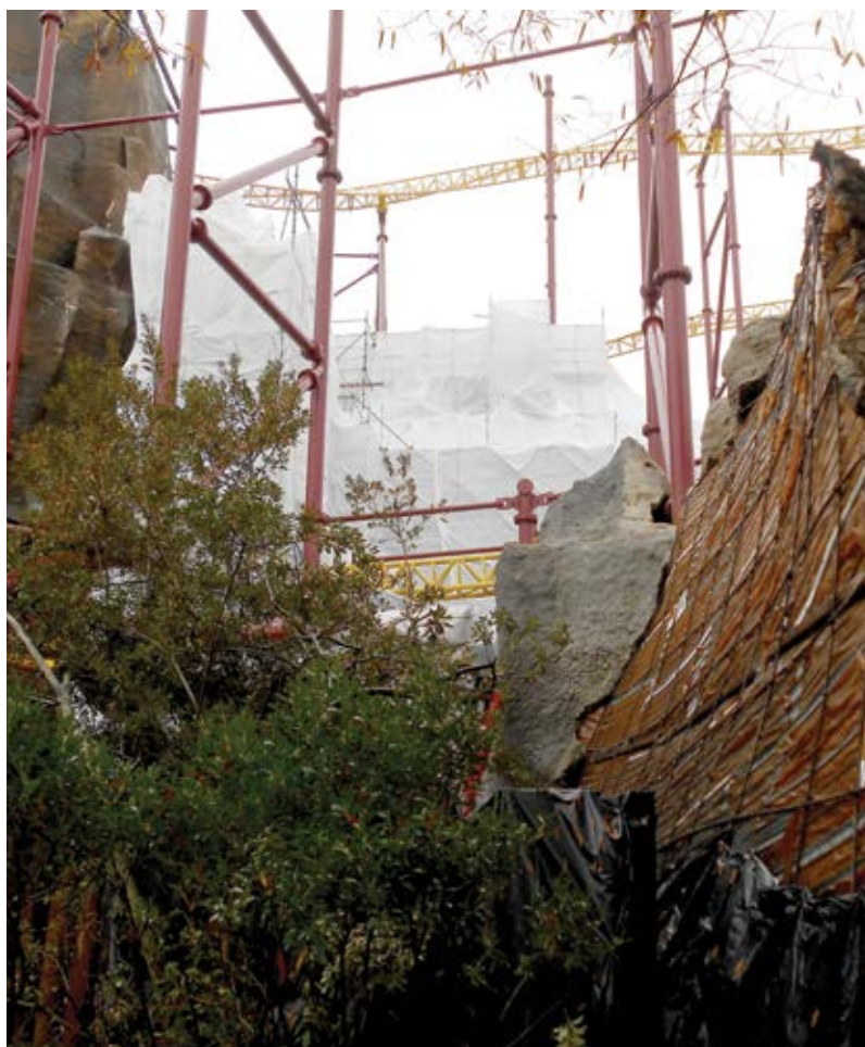
Fig. 4: Winter protection for the Volcano skin repair. Temperatures were kept between 47 and 50°F (8 and 10°C) on both sides of the shell. Concrete blankets were placed as added protection. Compression Strengths exceeded the specification for 7 and 28 days. Kings Dominion (Doswell, VA,) November 1, 2015 to March 15, 2016
