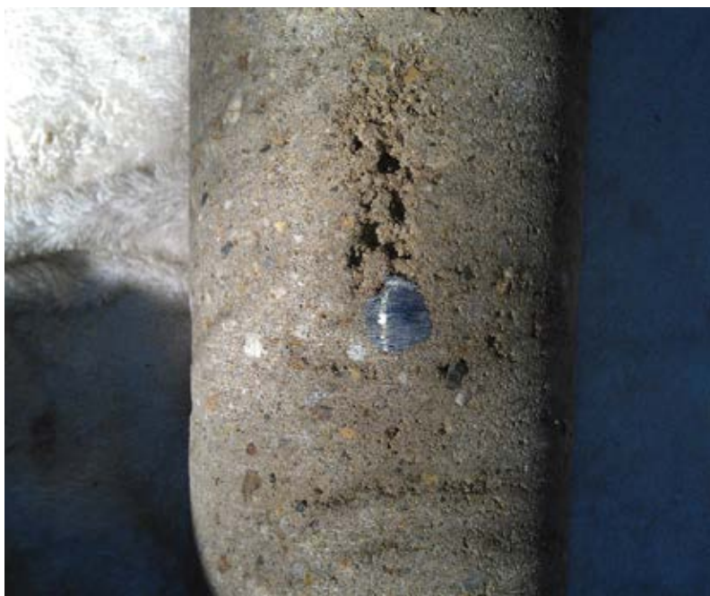
Fig. 1: Improperly compacted concrete behind steel
