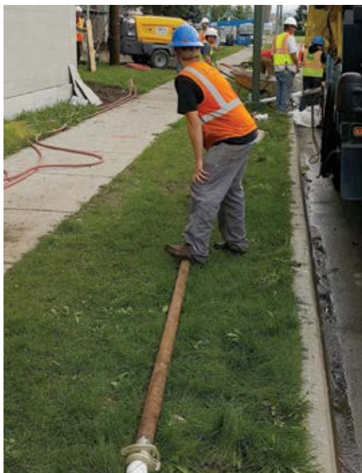
Fig. 4: The pump operator monitors the pipeline during priming. Using steel pipe enabled this mixture to be pumped at lower pressures
