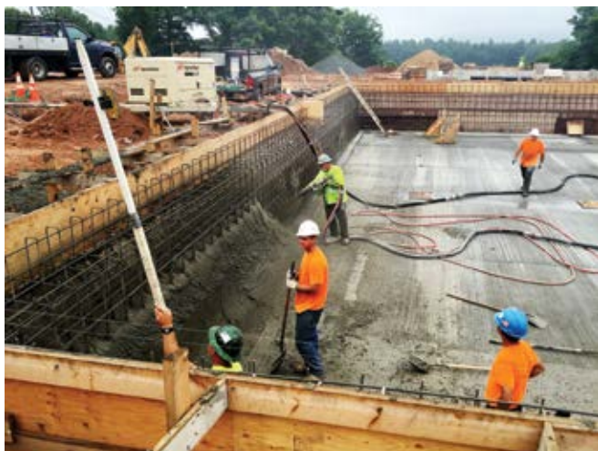
Fig. 1: Floor cast with installed keyway
