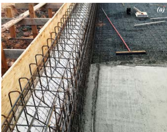
Fig. 1: Floor cast with installed keyway
