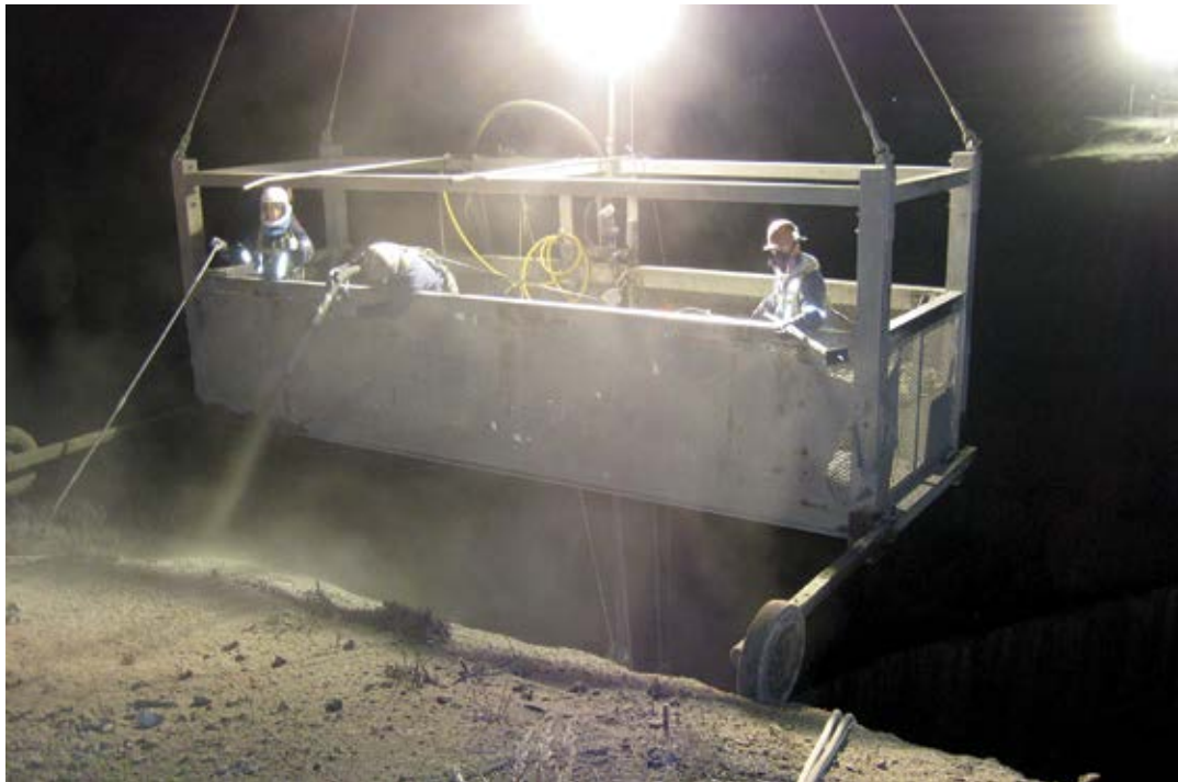
Nighttime shotcrete operations for slope stabilization
