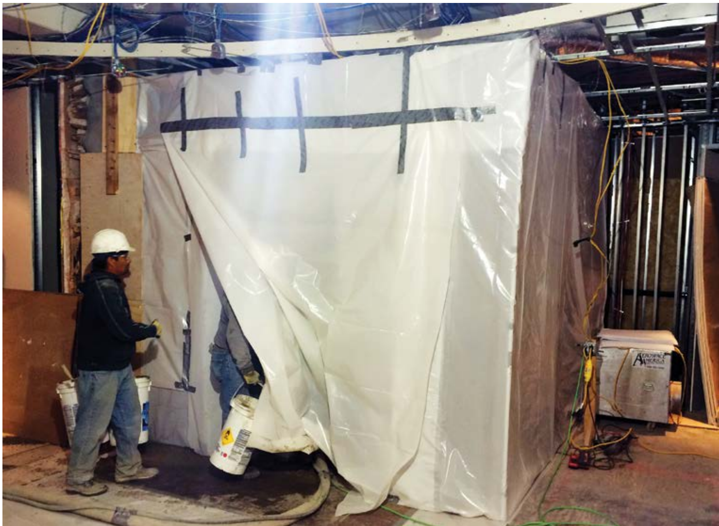
Fig. 1: This image shows an asbestos-like containment room to contain concrete repair work to its own area so that other trades could safely work around them
