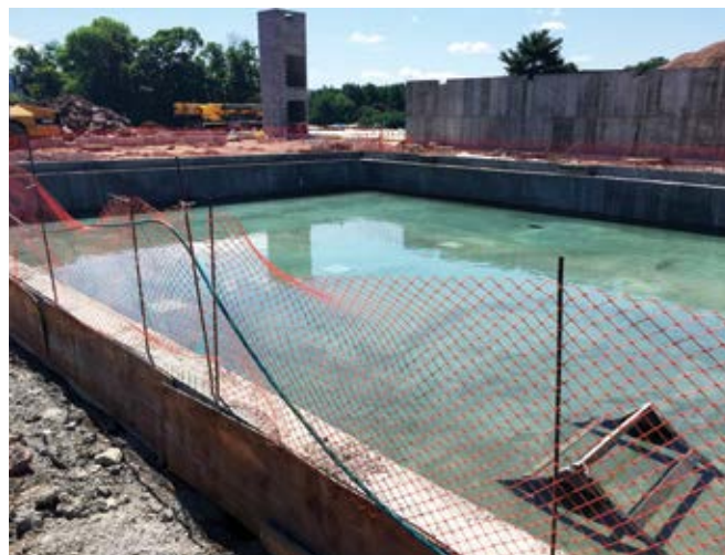
Fig. 3: Watertight tank test
