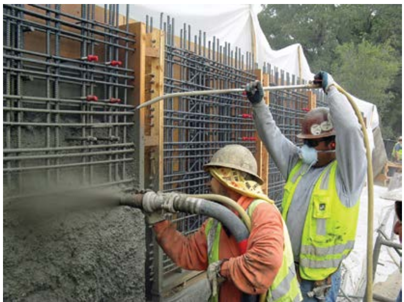
Fig. 4: Wet-mix shotcreting of structural wall
