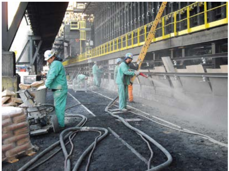
Fig. 3: Modern dry-mix shotcreting
