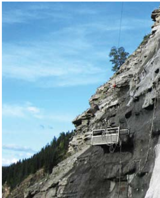
Basalite Microsil Shotcrete applied for slope stabilization, as shot by LRutt Contracting
