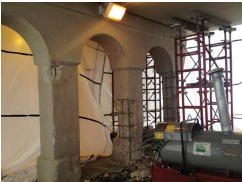
Fig. 5: Large propane heaters kept temperatures inside enclosure within specifications during cold winter months
