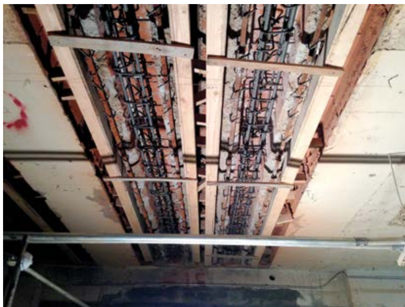
Fig. 2: This is a prepped area prior to shooting; sound existing reinforcing bar was left in place and reinforced with new reinforcing bar and dowels. The edge form was set to bind the sides of the joist infill
