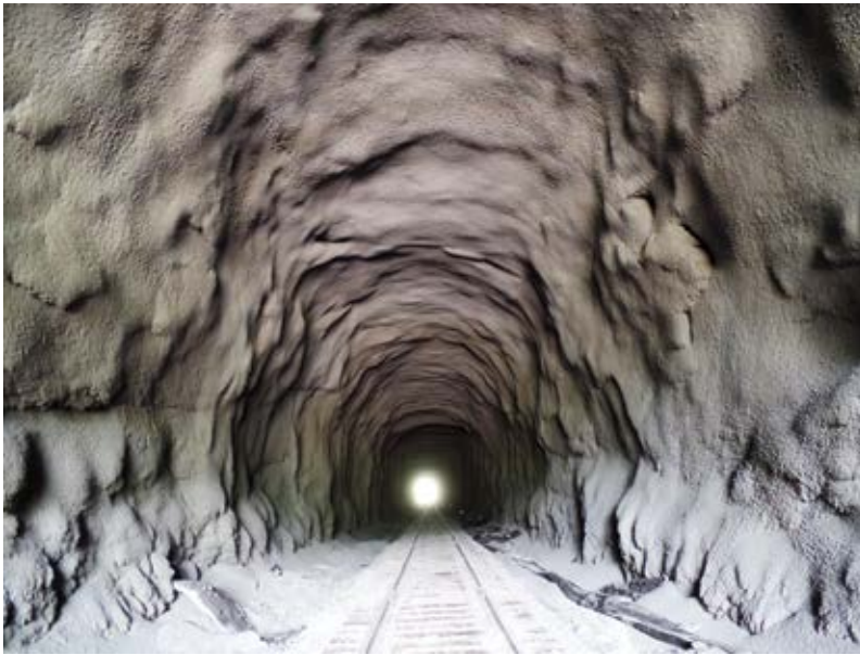
Fig. 6: View of final liner from west portal
