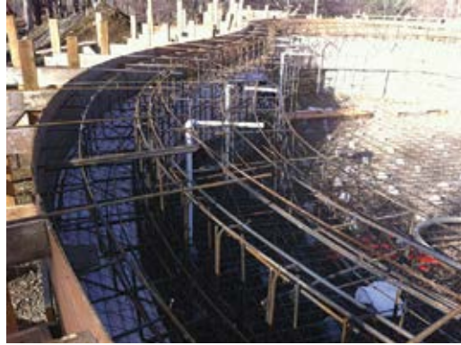
Fig. 4: Steel reinforcement on radius steps
