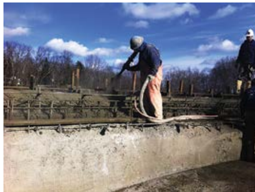
Fig. 6: Wall shotcrete and gutter detail
