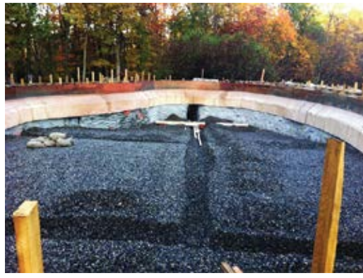
Fig. 3: Plumbing system under shotcrete shell
