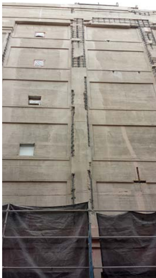
Fig. 5: The exterior façade that has been chipped back to sound material and reinforcing bar installed
