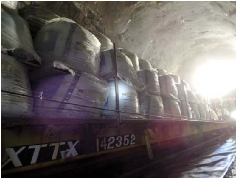
Fig. 5: Fifty bulk bags loaded on a flat car for final liner installation
