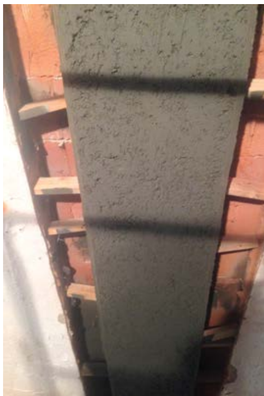
Fig. 3: The final shotcrete rod finish minimized the amount of work at the face
