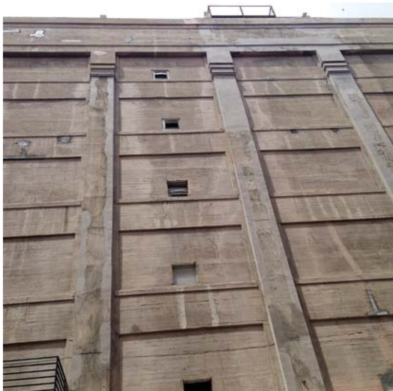
Fig. 7: The exterior façade after shotcrete operations were completed
