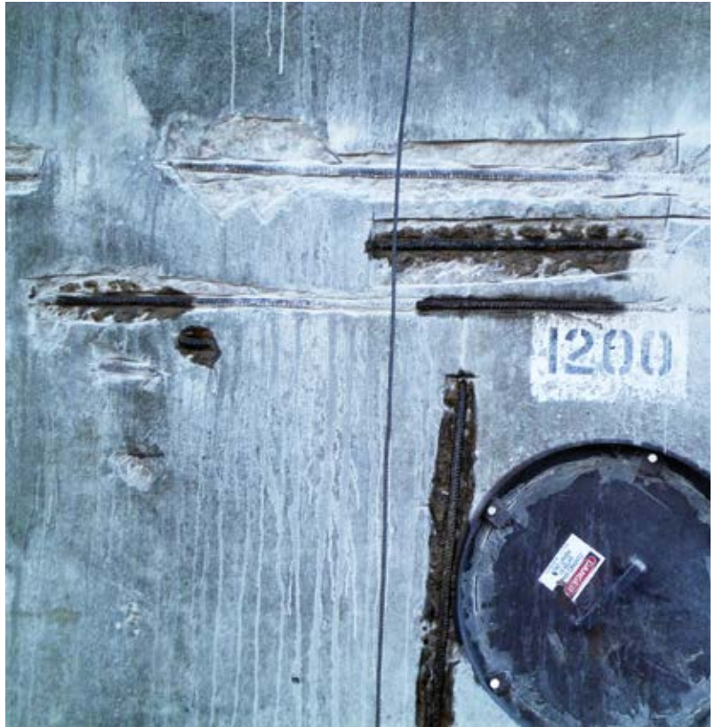
Concrete crack and spalling repair
