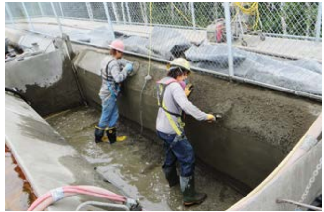
Fig. 8: Shotcrete crew cutting and doing the rough finish using mechanical trowel
