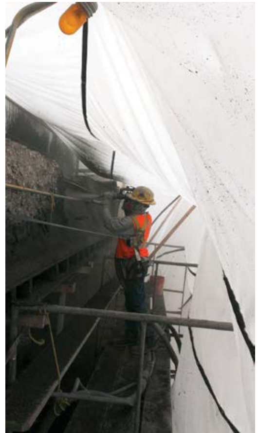
Fig. 6: Shotcrete placement inside a heated bridge enclosure
