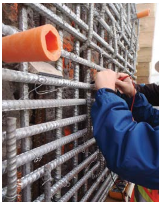
Fig. 3: Reinforcing bar sentinel tie-in
