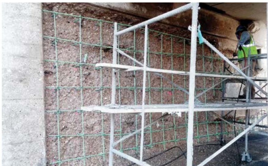
Fig. 1: Repair areas were found to be not only much larger in the field but also deeper than was called out on the plans and also lacking any reinforcing bar
