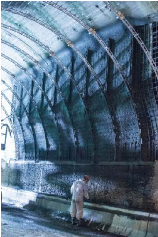
Fig. 9: Construction sequence Step 4—curved and vertical sidewall sections are shotcreted
