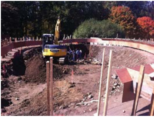
Fig. 1: Beam profile and edge forming
