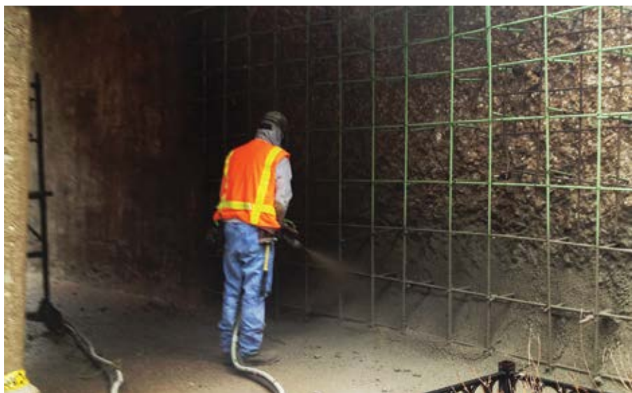
Fig. 3: ACI Certified Nozzleman shotcreting newly-reinforced repair areas
