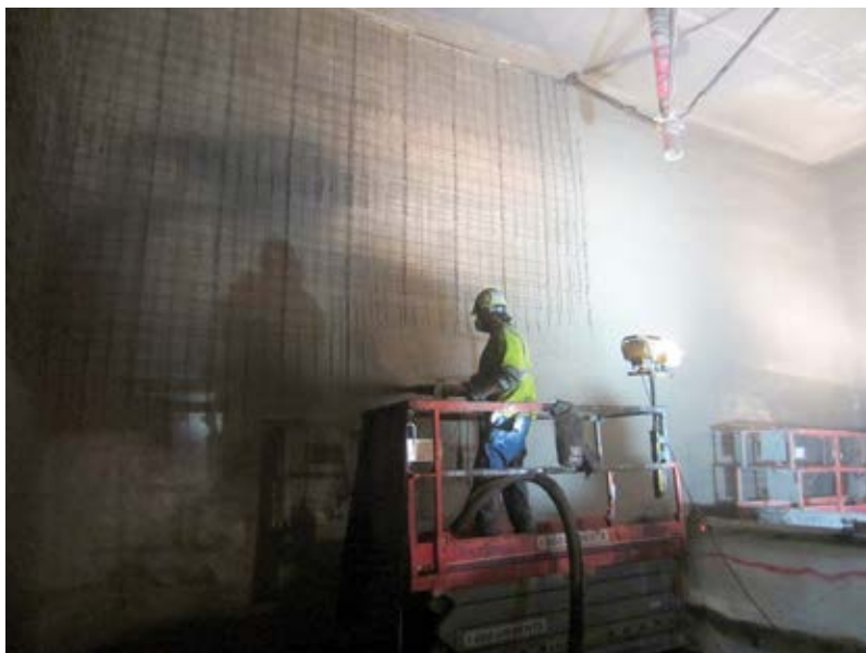
Fig. 4: Shotcrete placement
