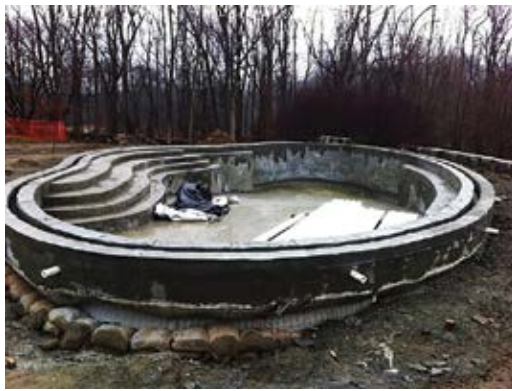
Fig. 7: Curing process for maximum strength gain
