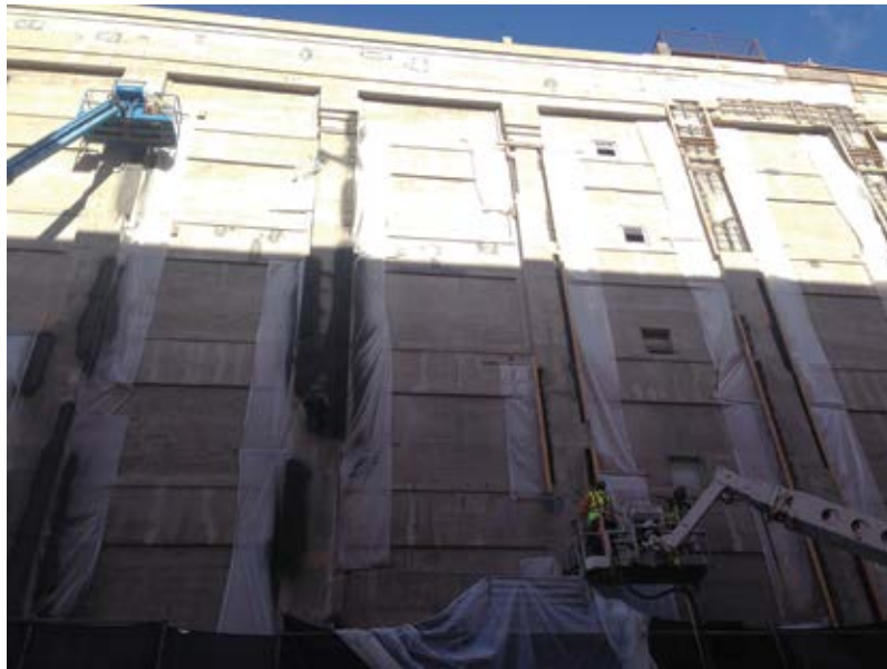
Fig. 6: The exterior façade during the shoot—several aerial man lifts were needed to properly reach the work spread over a wide area. This area was given a rubber float finish
