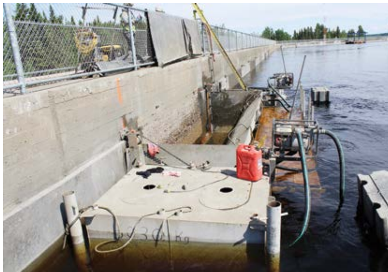
Fig. 5: Mobile cofferdam set up
