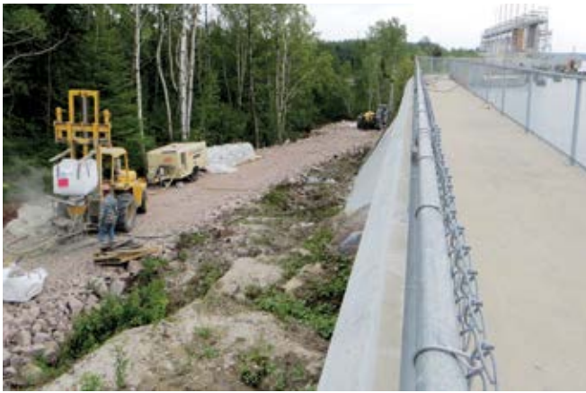
Fig. 7: Shotcrete equipment setup
