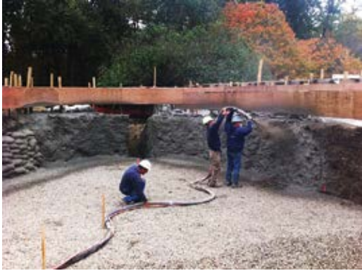
Fig. 2: Application of sacrificial shotcrete layer for soil containment
