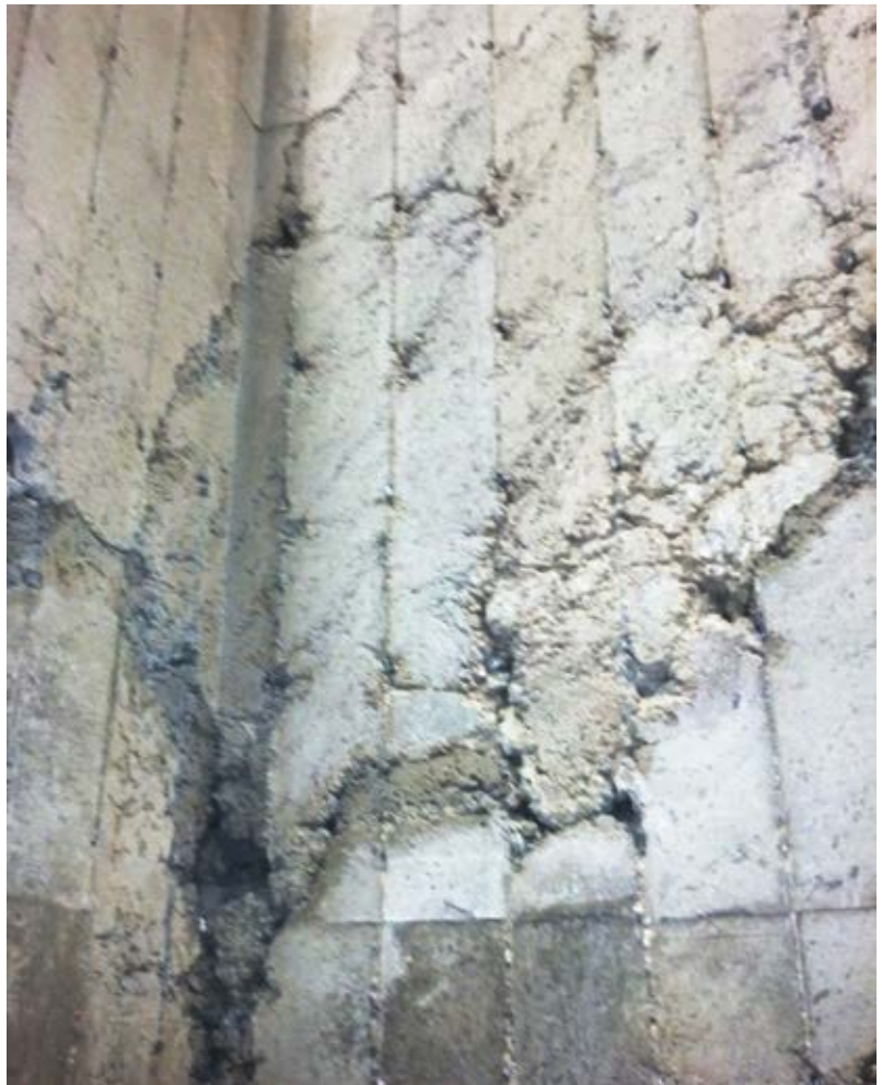
Fig. 2: Poorly consolidated concrete
