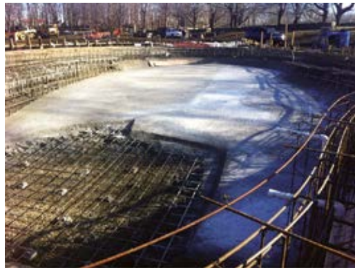
Fig. 5: Floor shotcrete (placed in stages)
