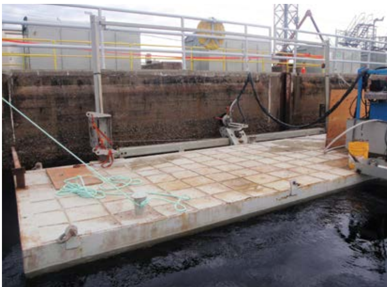
Fig. 2: Mobile hydrodemolition rig
