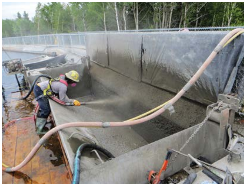
Fig. 6: Nozzleman shooting in mobile cofferdam system
