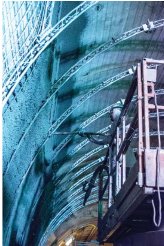
Fig. 9: Construction sequence Step 4—curved and vertical sidewall sections are shotcreted
