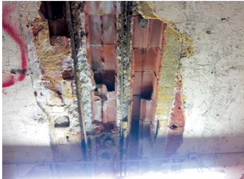
Fig. 1: An opened area showing the tile insulation and exposed existing reinforcing bar at the joists
