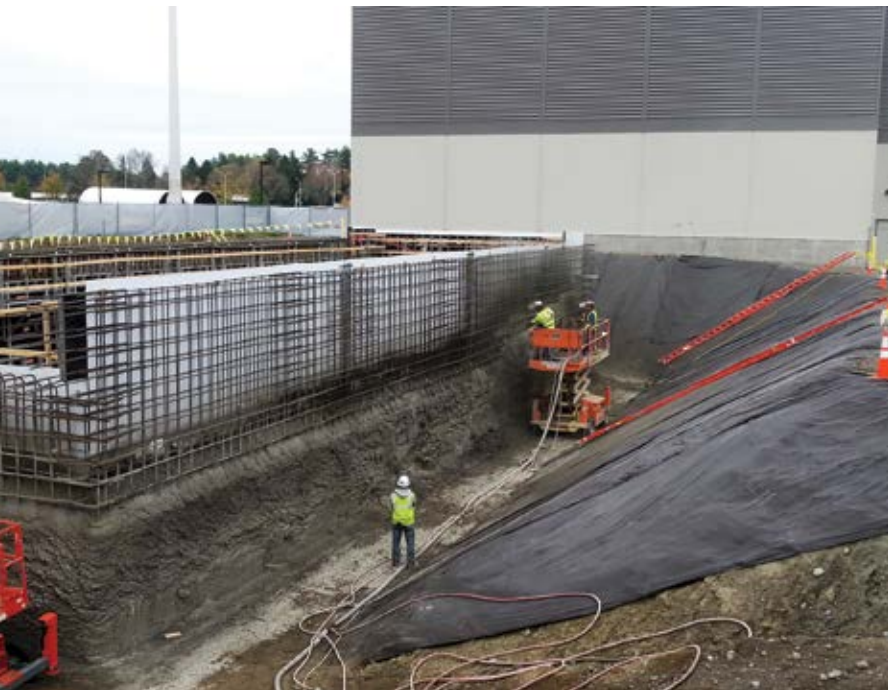
Fig. 2: Nozzlemen using scissor lift instead of scaffolding to gain access to the 270 ft (82.3 m) perimeter research tank project
