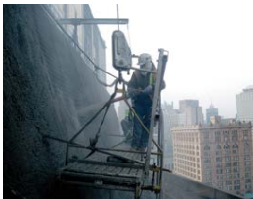
Fig. 4: Nozzleman on suspended swing stage, turning to his side, to get enough distance from the wall to get a good spray pattern
