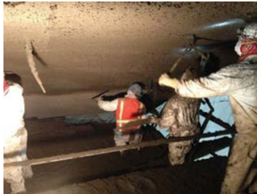
Fig. 8: Cutting of guides and finishing
