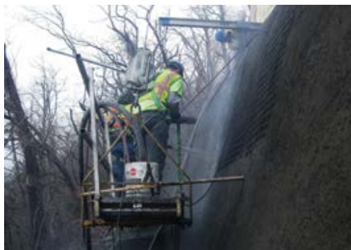
Fig 5: Nozzleman and cutdown man working together to complete upper areas of the eastern wall
