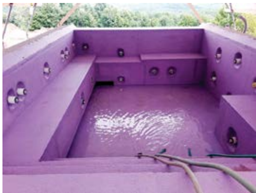
Fig. 1: A spa with a purple-colored waterproof membrane, undergoing a flood test prior to tile installation
