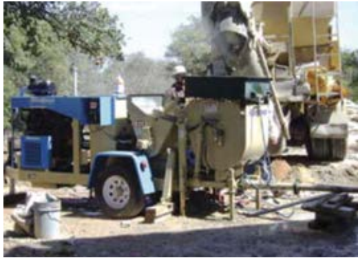
Fig. 12: An Allentown Powercreter 20 is shown with a hydraulic mixer attachment. The attachment is being used as a remixer for concrete supplied by a mobile, or a volumetric mixer for site batching to achieve a consistent mixture for pumping operations. A vibrating screen was installed to reduce the risk of plugging the 1.5 in. (38 mm) hose due to randomly occurring large aggregate particles. The electronic control technology produced a continuous flow of concrete material that allowed the nozzleman to apply a uniform shotcrete layer to the walls with very little line surge. The unit can pump concrete containing up to 1 in. (25 mm) stone mixes through a 4 in. (100 mm) hose
