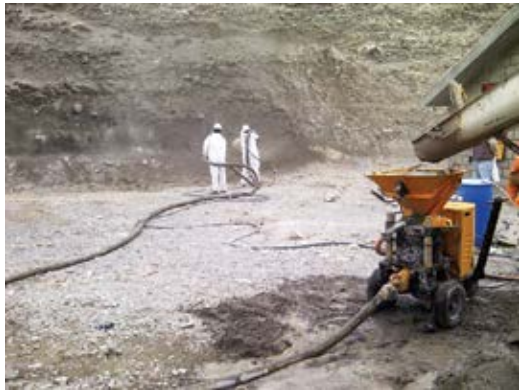
Fig. 1: Practicing slope stabilization with wet concrete in Arequipa, Perú, with an Aliva-257
