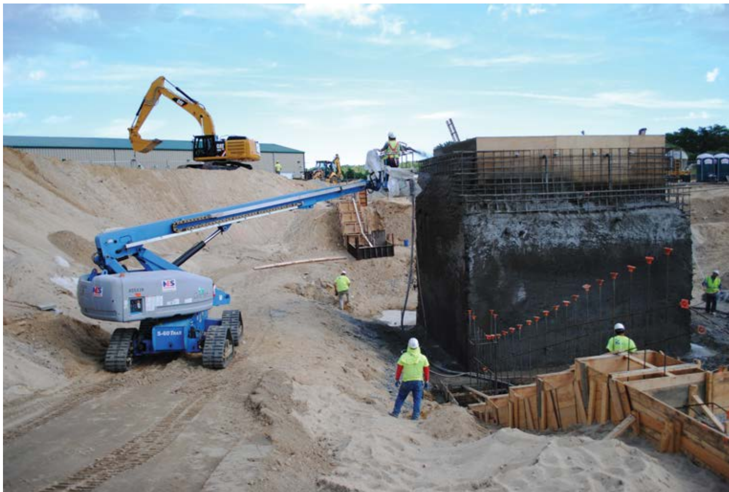
Fig. 1: Nozzlemen shooting a research tank from a lift. The site had terrible soil, which required an all-terrain lift with tracks instead of wheels to give safe access for nozzling and finishing
