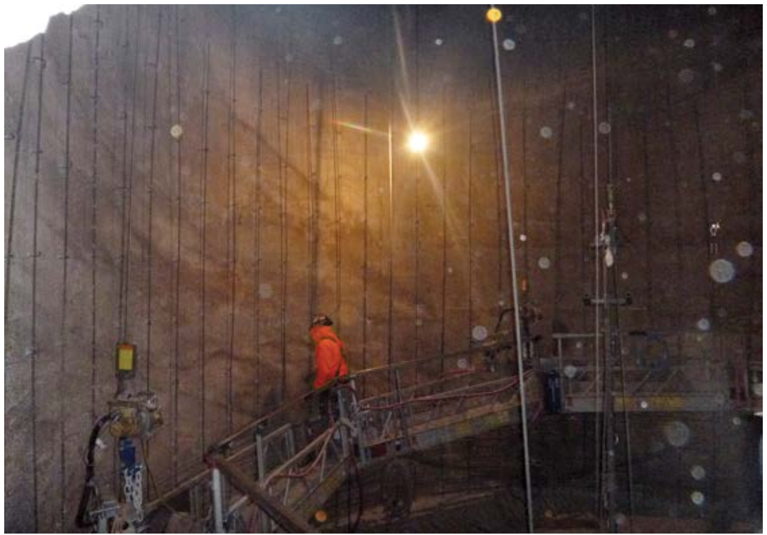
Fig. 2: Crews work to tie reinforcing bar on the interior of the grain silo to help support the new 5 in. (127 mm) shotcrete liner that will be installed
