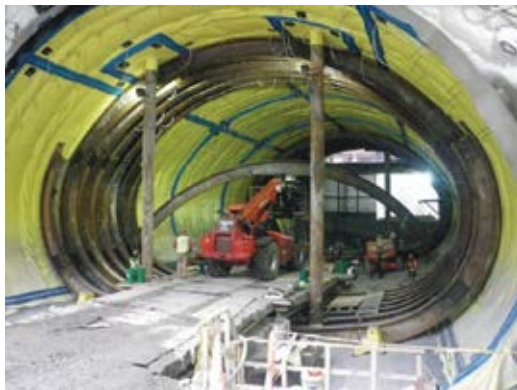
Fig. 4: Waterproofing and ring girders being installed
