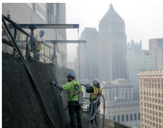
Fig. 3: Shotcrete is placed with Pittsburgh landmarks the Gulf Tower and Koppers Building in the background
