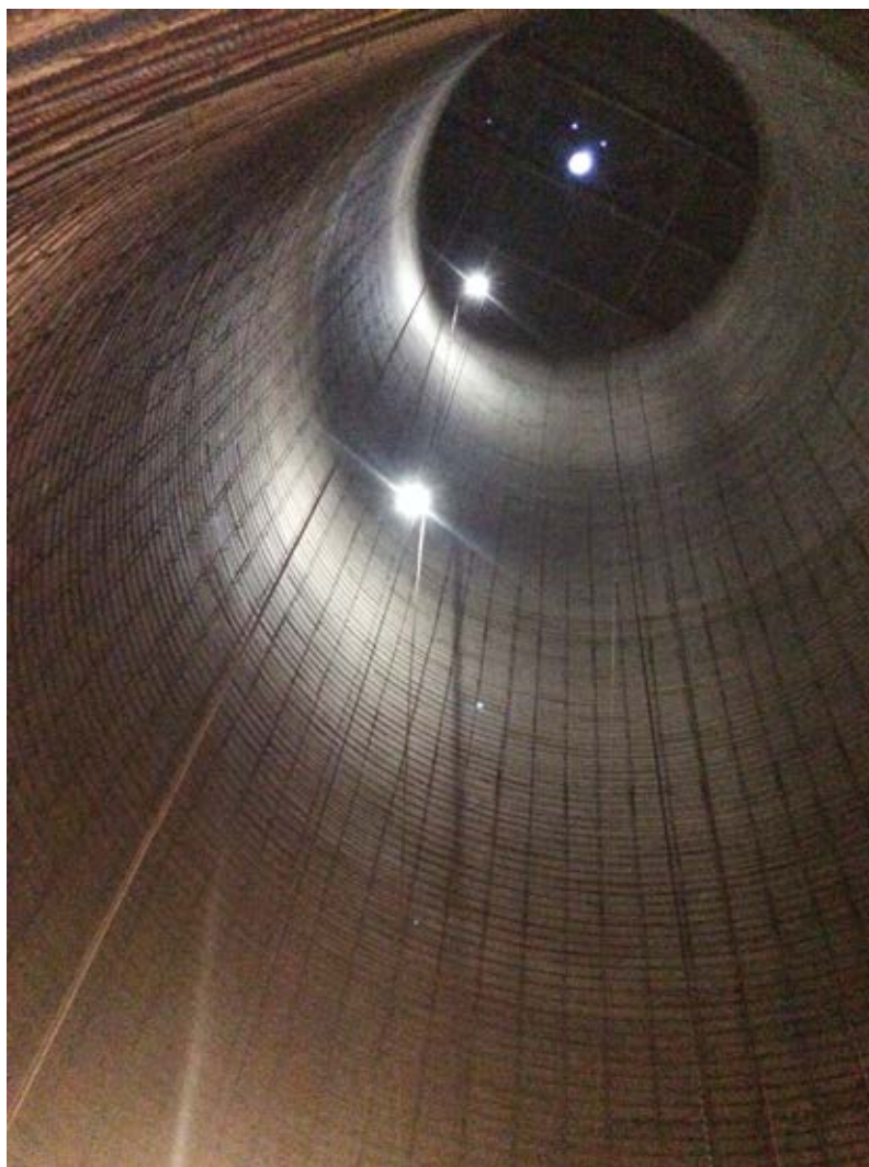
Fig. 1: Working on the 30 ft (9 m) diameter grain silo requires special equipment. McGill Restoration had to use specialized, blast-proof lights to generate enough light for their crews to safely complete their work
