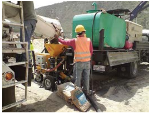
Fig. 2: Slope stabilization with Aliva-257 in Quito, Ecuador. One of the new roads leading to the new airport
