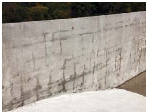
Fig. 2: A pool with shadowing of the reinforcing bar cage, indicating a non-watertight situation
