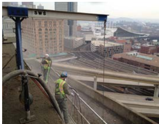
Fig. 2: Due to restricted access and nothing above to suspend cables from, outriggers were used to hang swing stages for the shotcrete rehabilitation work
