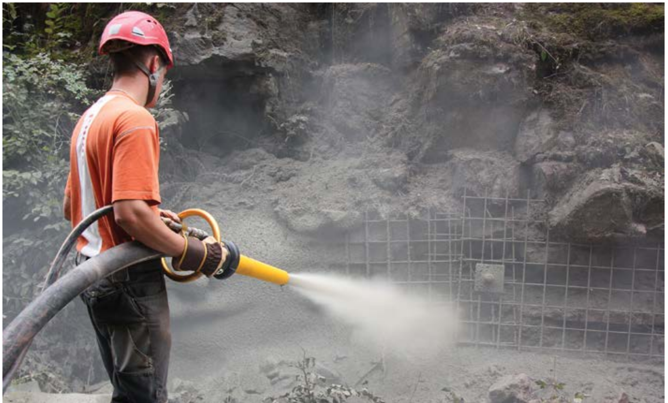
Fig. 3: Stabilizing rocks with wet concrete with Aliva-257. Here, the new Converto manual spraying gun is used
