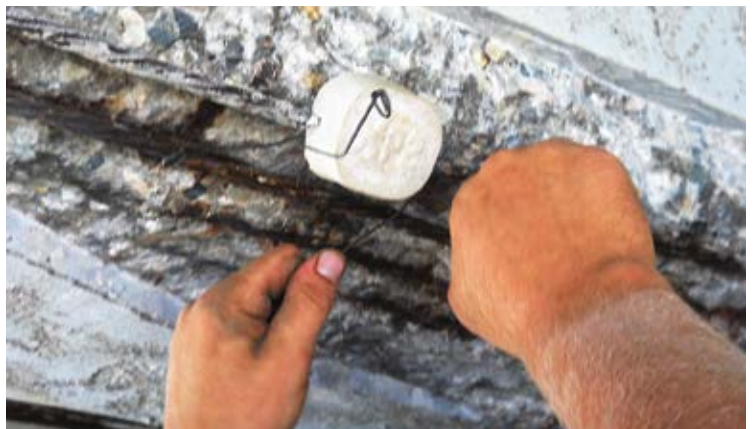
Fig. 3: Galvanic anode for concrete repair
