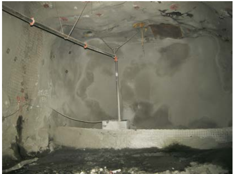
Fig. 3: A completed backfill barricade in a northern Ontario mine was constructed using the shotcrete process (note drainage pipes that allow water to drain from the backfill material)
