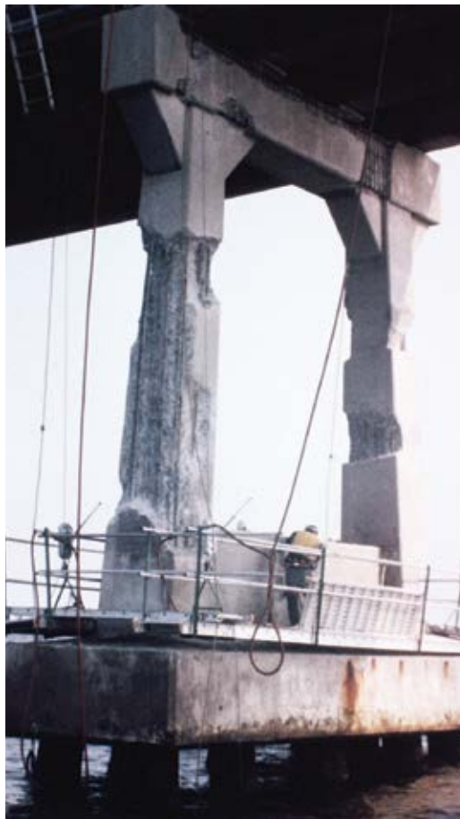
Fig. 3: Unsound concrete removed
