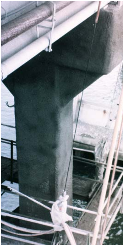
Fig. 4: Freshly shot pier column
