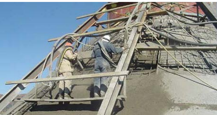
Nozzlemen shooting the base of the lighthouse
