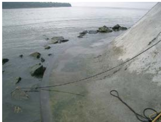
Completed shotcrete application at low tide
