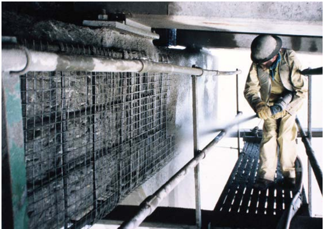
Fig. 5: Shotcreting pier cap
