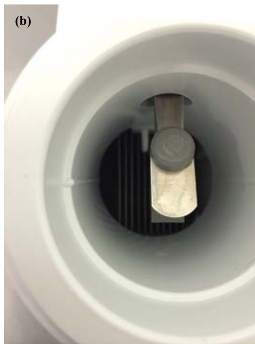
Fig. 3: Close-up views of a residential salt cell: (a) information it provides and the adjustments that can be made; and (b) close-up of the flow sensor which shuts the cell off when there is insufficient flow. Also shows the fins that provide the charges that separate the ions as the salt water passes through
