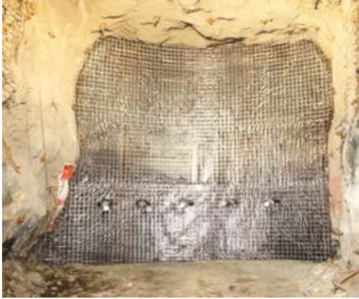
Fig. 1: Construction of original shotcrete backfill barricades involved the use of panels constructed using two layers of welded wire reinforcement, separated with spacers to act a vehicle for the shotcrete. Fabrene was usually fastened to the back of the first layer of mesh to provide a receiving surface for the shotcrete
