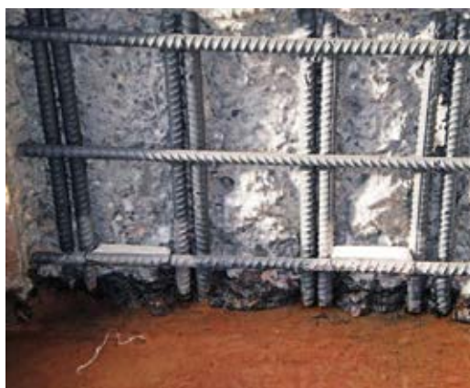
Fig. 10: Thin elongated anodes installed prior to shotcrete repair. Installation behind the reinforcing bar further reduces cross-sectional area
