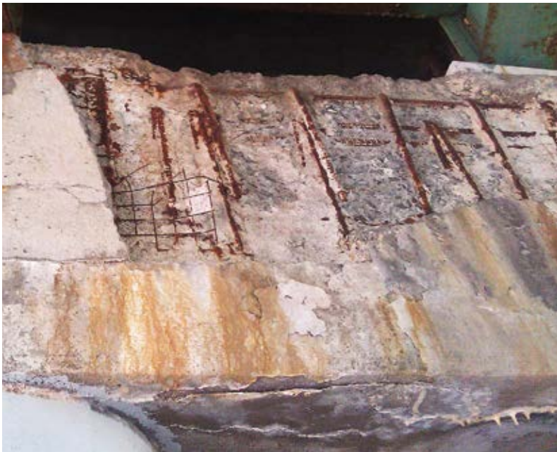
Fig. 1: Corrosion damage on concrete bridge pier
