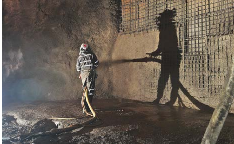
Fig. 2: Reduced manpower, reduced cycle time, and improved water retention soon made the shotcrete process the preferred method for constructing backfill barricades
