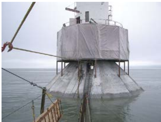
Completed shotcrete application at low tide
