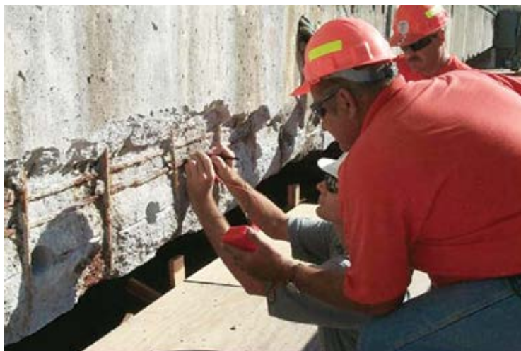
Fig. 6: Type 2 anodes placed into holes drilled into the parent concrete and connected to the steel in the repair
