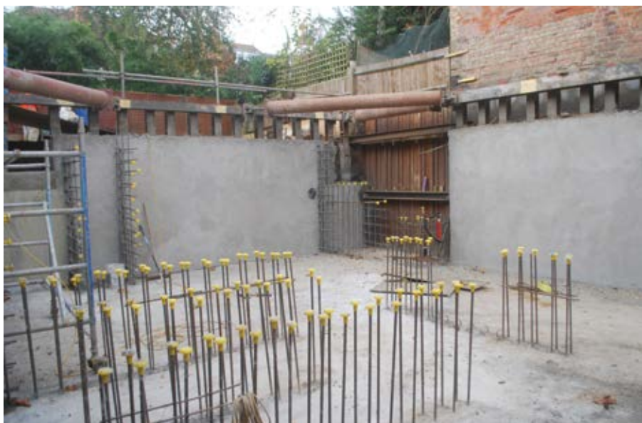
The integral crystalline waterproofing method also improved the shotcrete mixture's workability and gave the finished product a smoother architectural appearance (Photo courtesy of Abbey Pynford—Basement Engineering Specialists)
