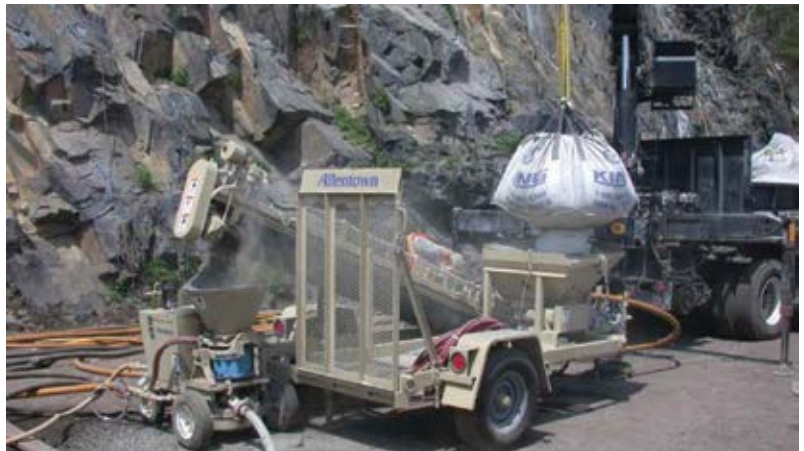
Fig. 3: Use pre-dampening equipment to reduce the amount of airborne dust at the machine and at the nozzle
