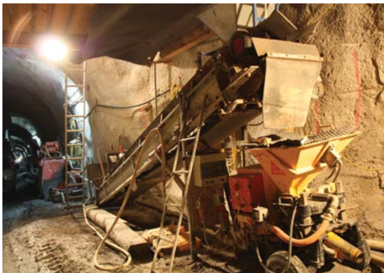
Spraying machine Aliva 257 with on-site conveyer belt
