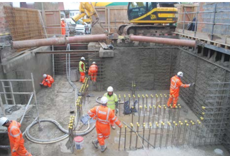
After a unique piling system was developed and implemented for this project, shotcrete containing KIM crystalline waterproofing admixture was applied to the slab and walls of the basement (Photo courtesy of Abbey Pynford—Basement Engineering Specialists)
