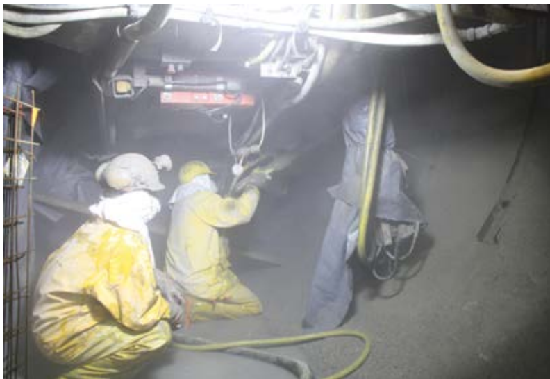
Spraying device for dry-mix shotcrete spraying (behind the drill head)
