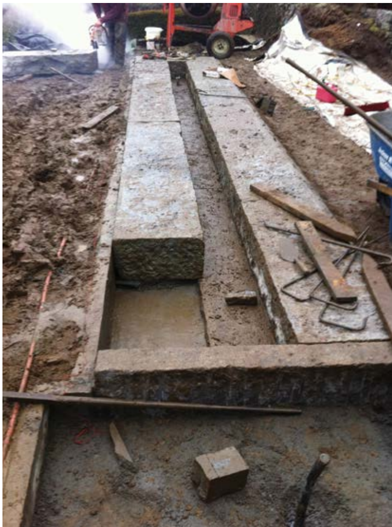
Fig. 3: Shotcrete trough with reclaimed granite installed. Notice the shotcrete step support for granite stones
