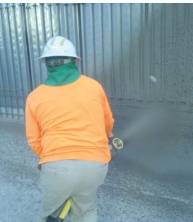
Fig. 2: Exterior shotcreting from the ground
