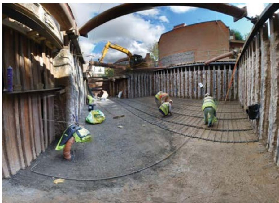
Using shotcrete and KIM together allowed the basement to be constructed right to the property line without affecting the neighboring homes (Photo courtesy of Abbey Pynford—Basement Engineering Specialists)
