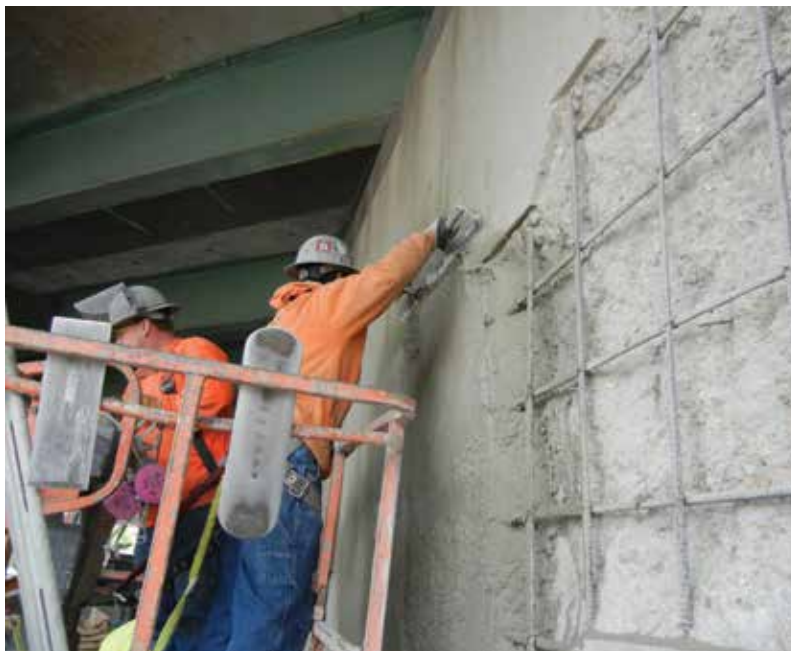
Crew finishing Rapid Set shotcrete over reinforcing steel
