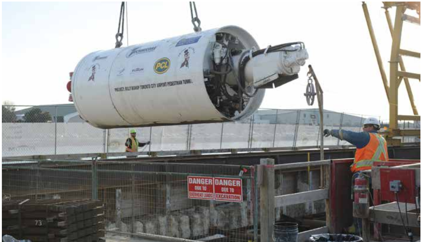
Fig. 2: Two purpose-built, Canadian-made tunnel-boring machines, dubbed “Chip” and “Dale,” were launched to bore the seven interlocking “tunnel drifts,” forming the unique arched crown design of the main tunnel
