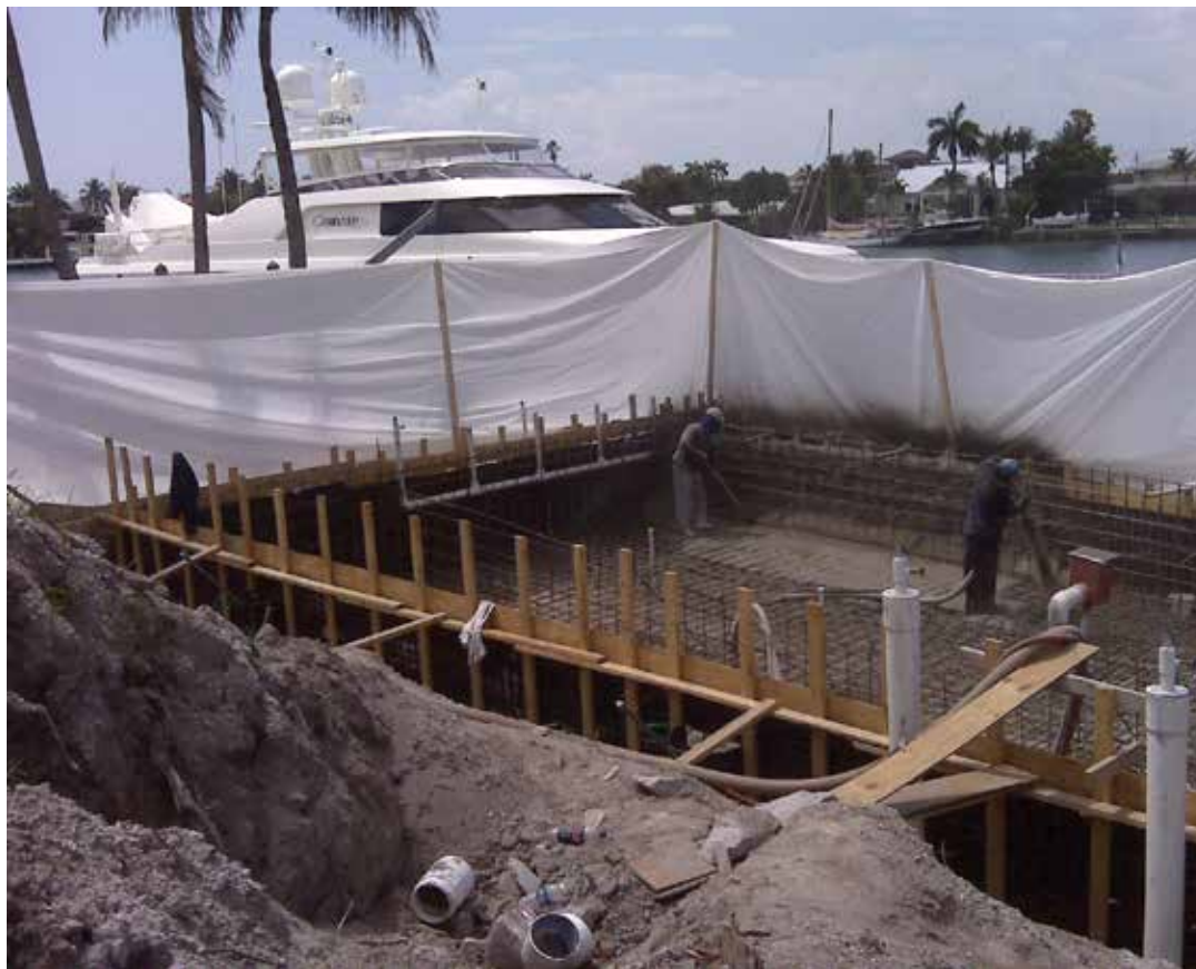
Fig. 1: Typical formwork for pool construction
