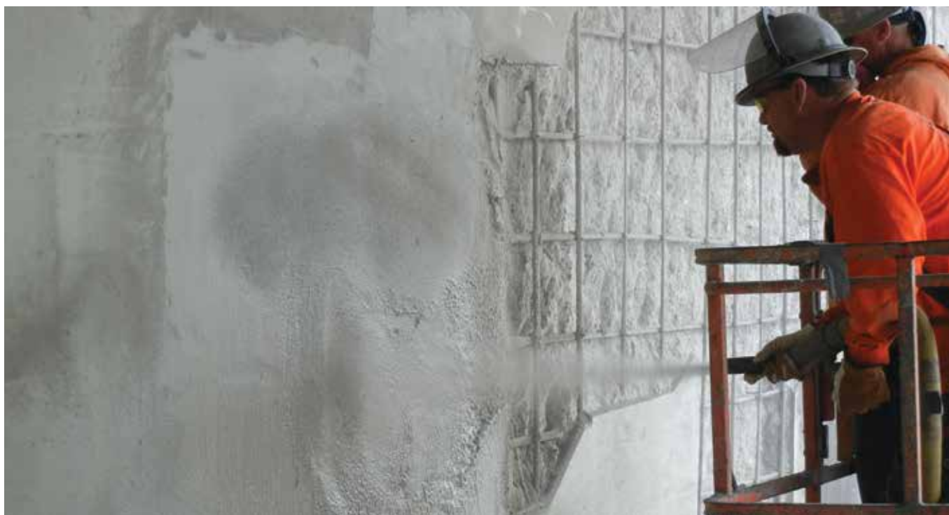
Application of Rapid Set shotcrete on a repair of a highway overpass
