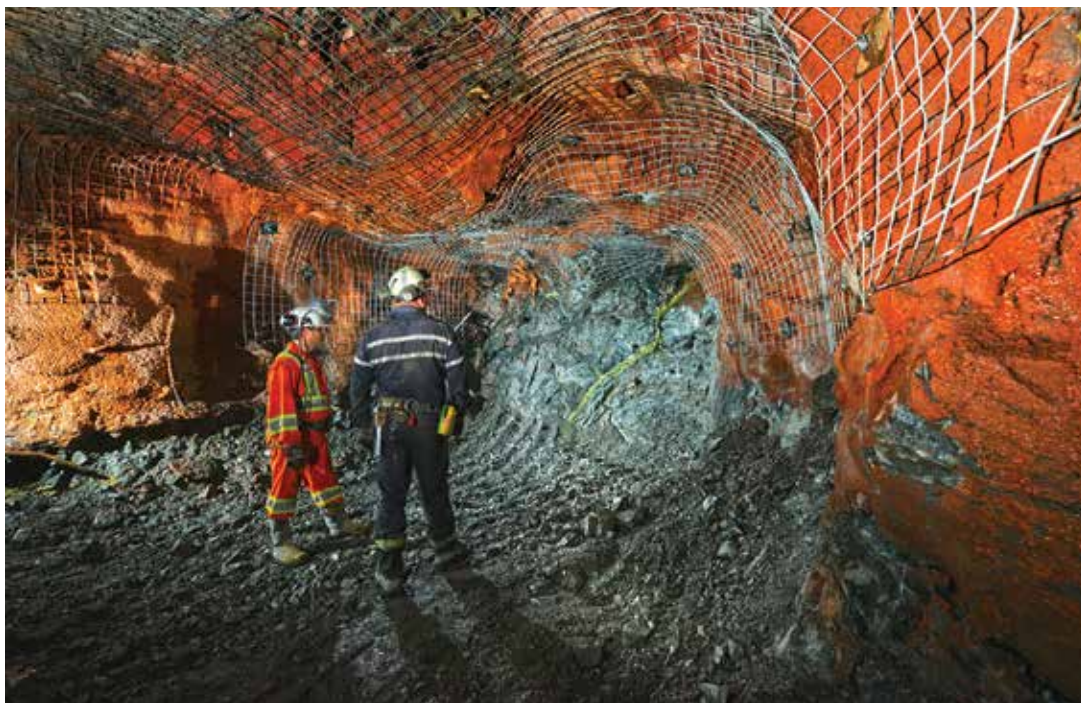
Rapid-setting dry process shotcrete with red pigment for underground and tunneling applications Photo courtesy of King Packaged Materials
