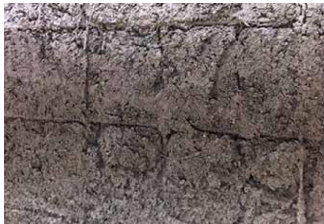
Fig. 2: Uneven flow (slugging) has displaced in-place shotcrete. Note signs of sagging below the wire reinforcement
