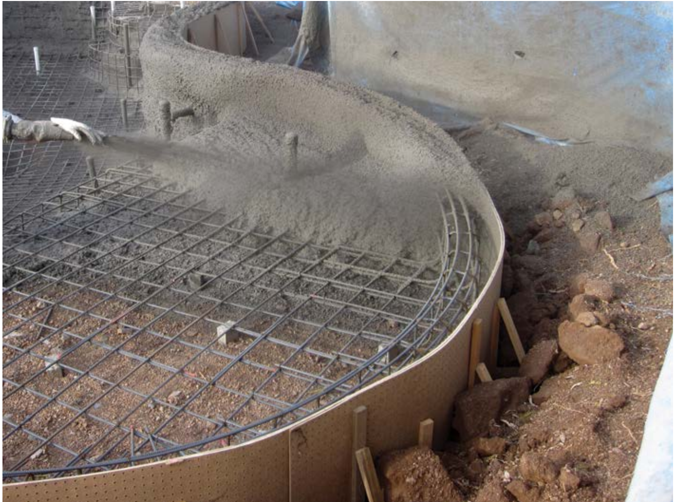
Fig. 4: Short pegboard forms poorly supported with undersized staking allows for movement at the top of forms during shotcreting
