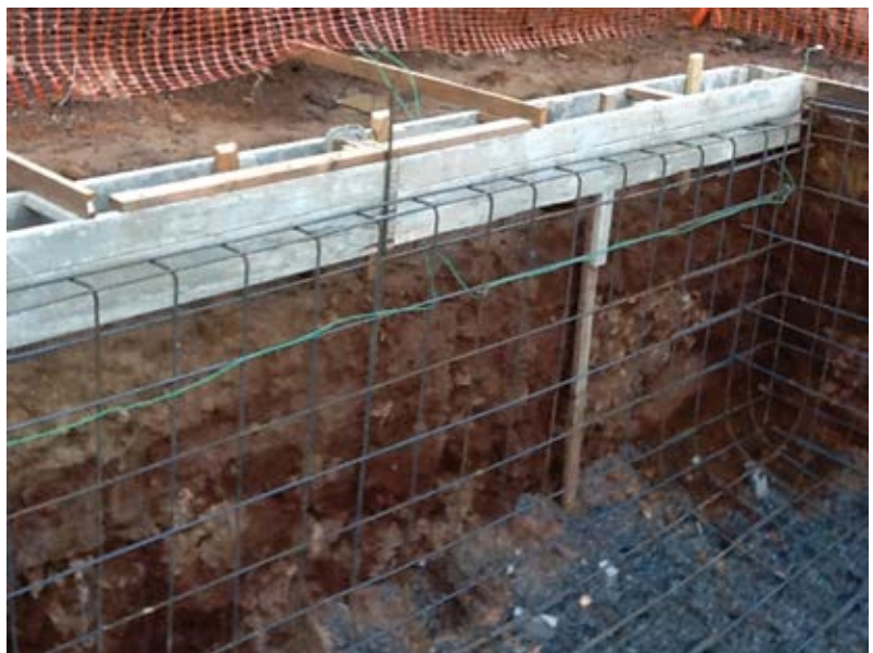
Fig. 2: The rocky soil has been trimmed to accept the shotcreted pool shell
