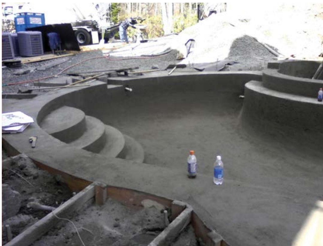
Fig. 7: Proper Steeltex forming allows the shotcrete crew to focus on their placement and finish details
