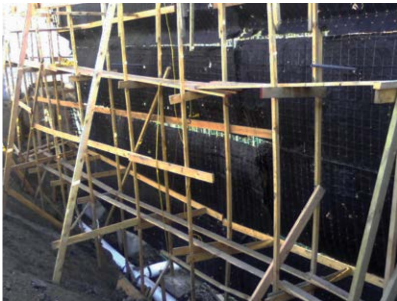
Fig. 5: A 13 ft (4 m) tall pool wall with Steeltex® hung haphazardly, with a terrible lack of support by undersized and insufficient wood forms
