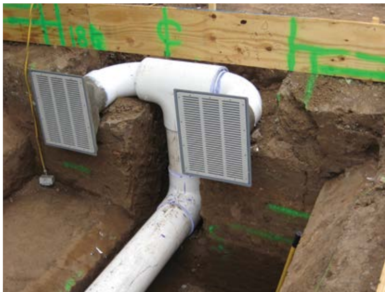
Fig. 1: The subgrade has been carved to the profile required, including trenching of plumbing lines beneath the future pool shell
