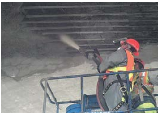
Fig. 9: Nozzleman using anti-static dry-mix hose
