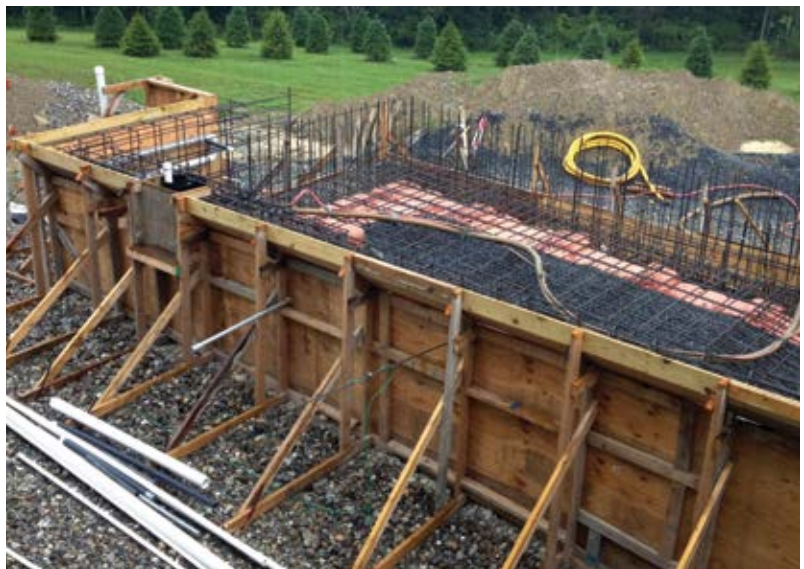
Fig. 3: A significant set of wood forms, well-reinforced, for a negative-edge pool being built above grade
