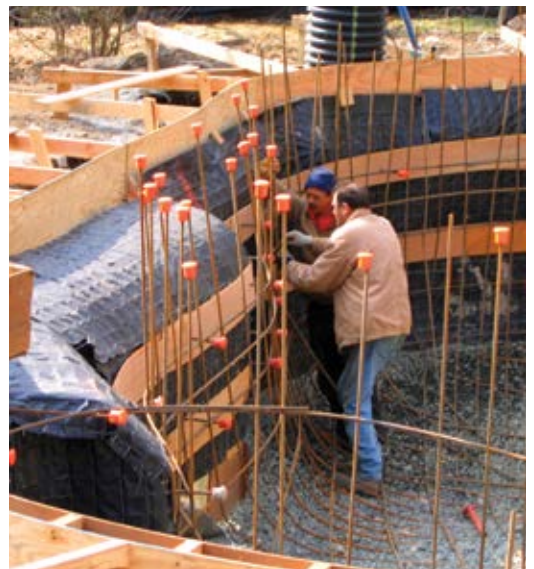
Fig. 6: Steeltex forms properly set with overlaps, wood staking behind, and plywood ribs attached to the front
