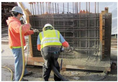
Fig. 1: A typical preconstruction test panel with congested reinforcement
