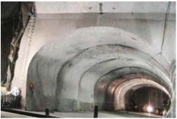
East Side Access, New York, NY: Elevator inclined shaft final lining for tunnel
