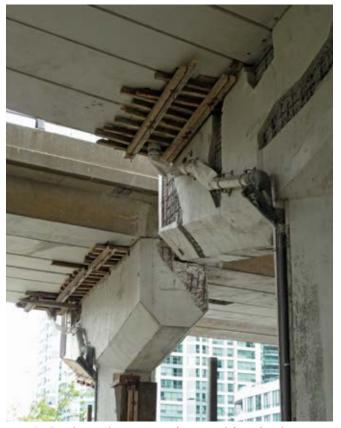
Fig. 3: On elevated structures, forms and form hardware must be lifted into place and removed several days later
