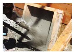
Fig. 2: Nozzleman initially places material into the panel's lower corners while close in
