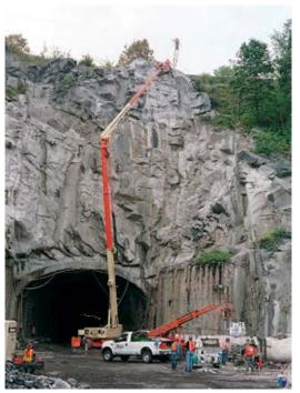
Fig. 2: Properly placed shotcrete is a team effort: the pump, mixer, and nozzlemen are pictured here
