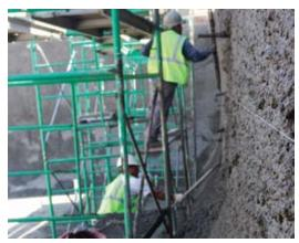
Fig. 3: Pre-job toolbox talks should identify daily risks. Inform workers of the safe operation and use of required tools, such as job-specific scaffolding, before work commences
