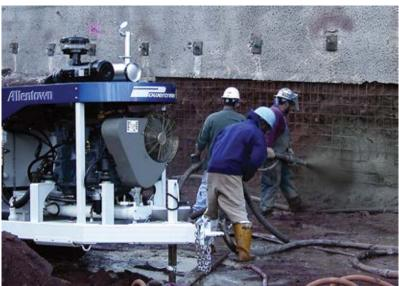
Fig. 3: Pump, nozzleman, and hose tenders
