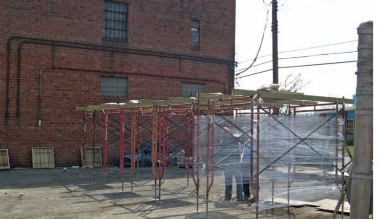
Fig. 1: Overhead panels prepared prior to the day of shooting, braced and set in an orderly fashion
