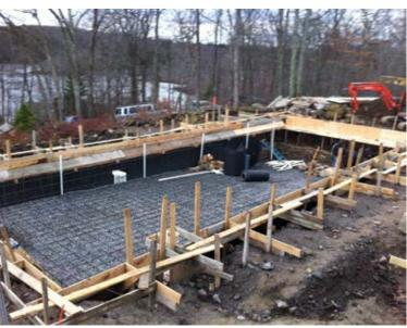
Fig. 1: Lightweight, one-sided form is all that's needed when using shotcrete
