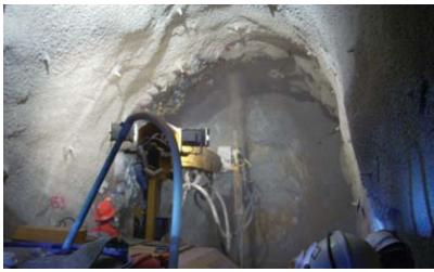
Fig. 2: Sprayer starts at bottom of wall on right and sprays up, over, and down the opposing wall—overspray is deposited on the left side wall
