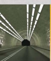
When Pittsburg's 80-year-old Liberty Tunnels needed structural repairs, QUIKRETE<sup>®</sup> Shotcrete MS got the job done. Crews were able to complete their work within tight time constraints using the dry process with a pre-dampener. In fact, our Shotcrete products were part of the American Shotcrete Association's "Outstanding Underground Project" for 2009 and 2010.
