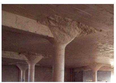
Fig. 3: Severe deterioration of the interior support columns prior to restoration
