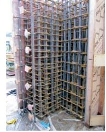
Fig. 2: Type 1 preconstruction test panel was composed of three curtains of No. 10 (No. 32M) and No. 9 (No. 29M) reinforcing steel with additional boundary reinforcing bar elements
