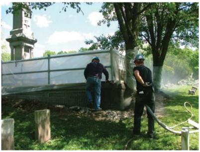
Fig. 4: After the deteriorated concrete was chipped out, the surface was prepared and meshed and the shotcrete was gunned in place
