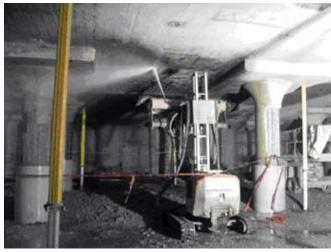
*Fig. 2: The majority of concrete removals were performed by hydrodemolition*
