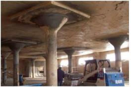
Fig. 4: Support columns are restored to their original rounded and flared condition using shotcrete
