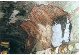
Fig. 4: Large repair area prior to shotcrete
