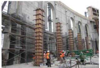
*Fig. 5: Application of 40 ft (12.2 m) tall shotcrete layer 36 in. (914 mm) thick over the existing historic perimeter wall*
