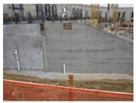
Fig. 7: Shotcrete shear wall after the forms were stripped. The right side of the wall is the stripped form side. The left side is the shotcrete steel trowel finish side
