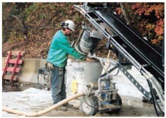
*Fig. 4: Dry-process equipment and operator during the shotcrete installation of an underground culvert*
