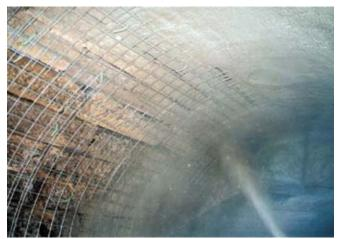
Fig. 5: Dry-process shotcrete being gunned overhead in an underground culvert. The roadway was opened the following day
