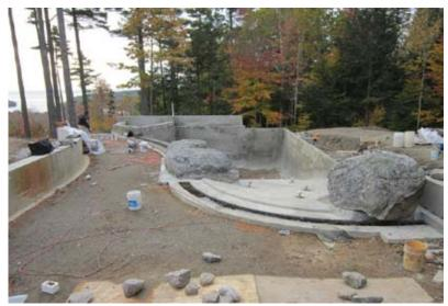
Fig. 4: Completed shotcrete with large rocks placed
