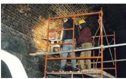
Fig. 3: Trailer-mounted core-drilling setup for drilling holes for drainage pipes. Also note the freshly repointed brick mortar joints
