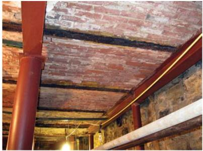
*Fig. 3: These brick arches are in one of the open sections of the supporting floor system*
