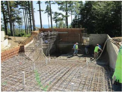
*Fig. 2: Elaborate reinforcing required by the pool design as we start the second phase of shotcrete*
