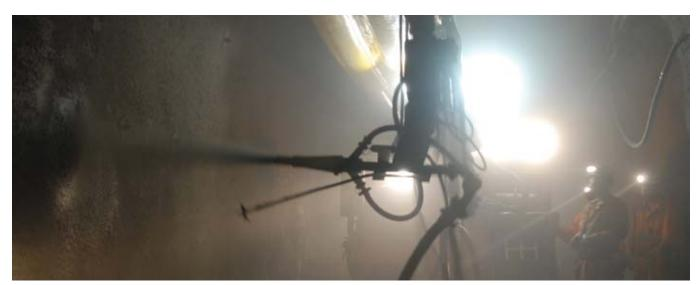
Fig. 1: Once the shotcrete has hardened, will its creep characteristics suit the degree of ground movement expected?
