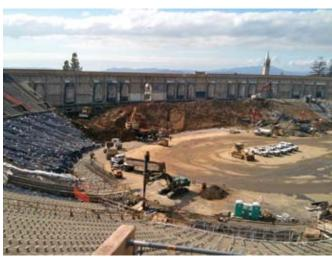
Fig. 1: Overview of the existing historic walls during demolition and excavation. A layer of shotcrete was later applied over the existing walls in various thicknesses from 5 to 36 in. (127 to 914 mm)
