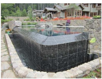
Fig. 6: Completed pool from the negative-edge side
