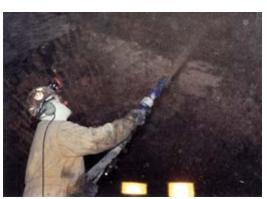
Fig. 5: Shotcrete being placed
