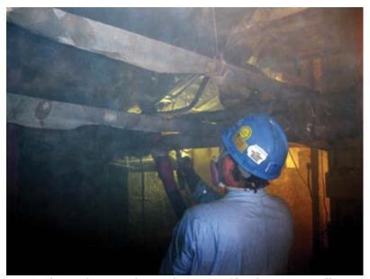
*Fig. 6: The nozzleman is placing shotcrete overhead in an especially congested area of the basement behind the elevator shaft*
