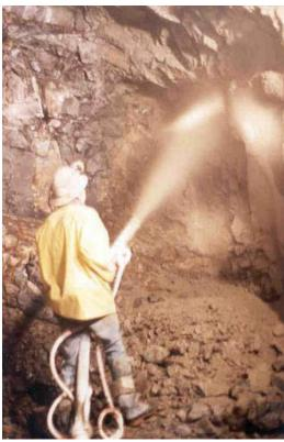
*Fig. 3: Even some hand nozzling is improperly sequenced*
