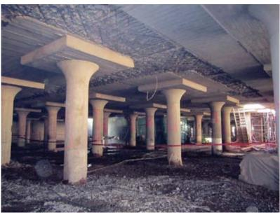
Fig. 4: Final stage of removals prior to shotcrete application
