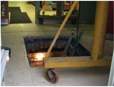
Fig. 2: In this access hole, which was cut to gain access into the building's basement, a side view of a supporting brick arch is visible
