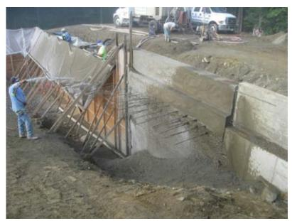
Fig. 3: Deep excavation required for forming and, subsequently, filling with free-draining stone to prevent frost heave. Also seen is the dowel reinforcing bar that was tied into the pool floor in the second phase
