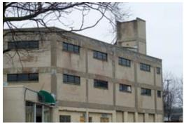
Fig. 5: Exterior of the structure showed signs of neglect with crumbling and deteriorating concrete
