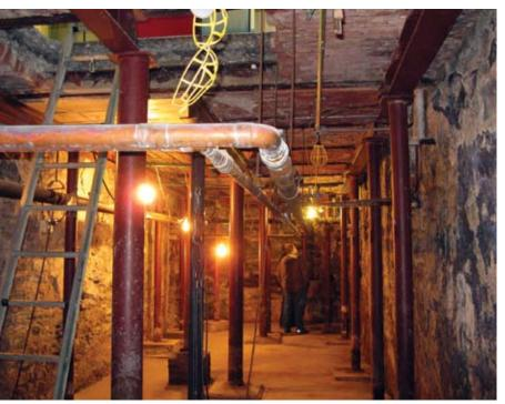
*Fig. 5: Working around the structural supports, piping, conduit, and other obstructions added to the difficulty of the overhead shotcrete placement*
