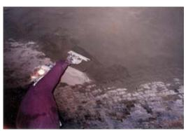
Fig. 6: Shotcrete being cut back to finish grade
