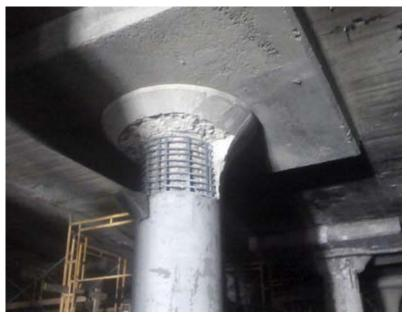
Fig. 5: Column prepared for shotcrete application
