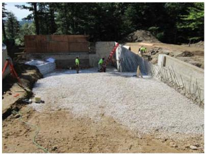
Fig. 1: Stone underlayment along with the reinforcing bars penetrating out of the first phase of construction so the second-phase pool section could be tied in correctly
