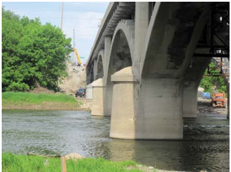
RAM's scope of work called for rehabilitation of abutment walls, wing walls, arch spans, and piers
