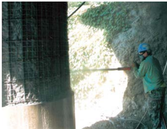
The shotcrete placement on this bridge pier is gunned to the full depth in one continuous pass. It is better to avoid gunning in layers whenever possible
