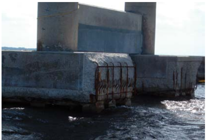
Pile caps after chipping and ready for shotcreting
