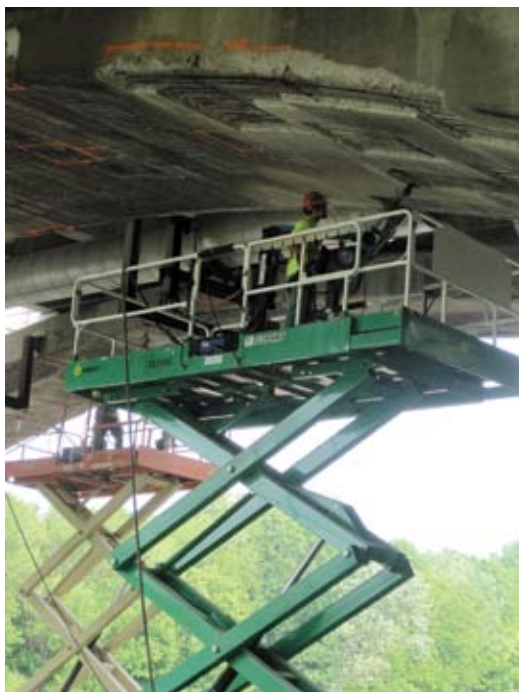
Repair access on the underside of the bridge spans using scissor lifts
