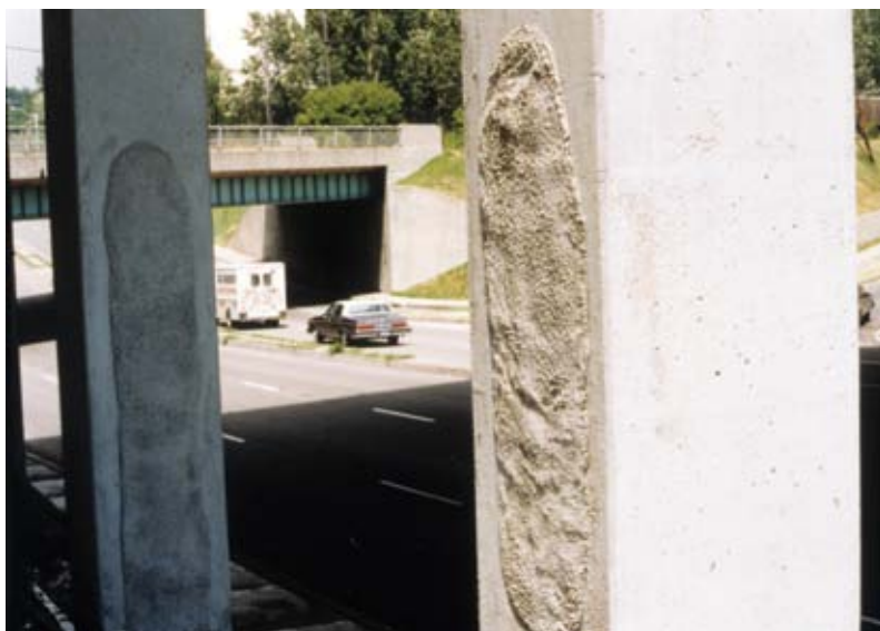
The specification for latex-modified shotcrete required that hand finishing be minimized, leaving the repair with a gun finish
