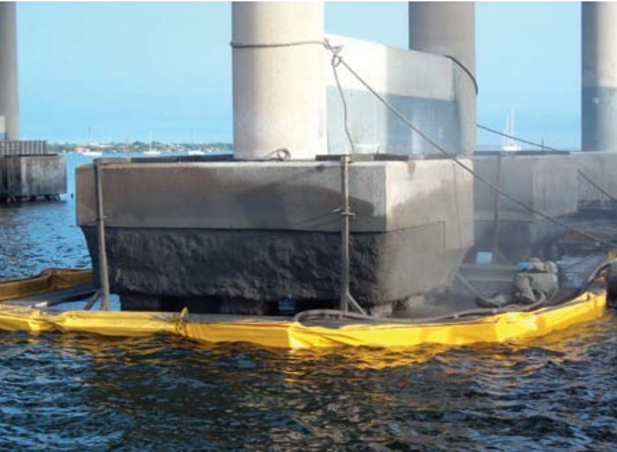
Shotcrete placement on low water pile caps
