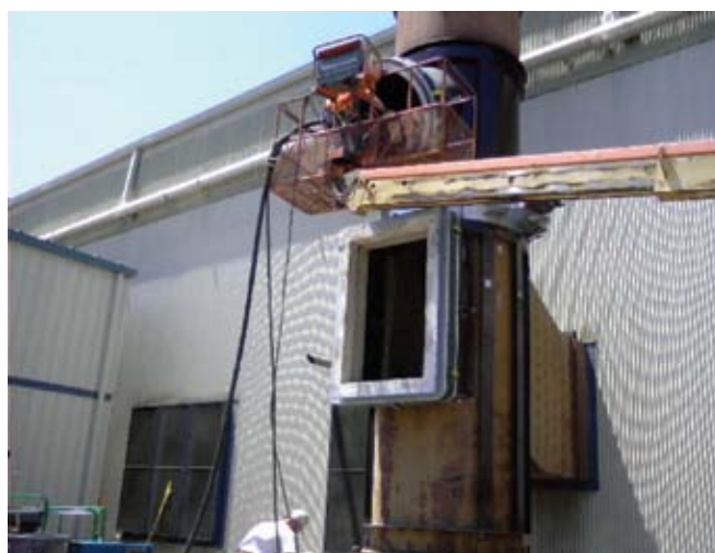
The shotcrete hose running up into the smokestack conveys the refractory material directly to the areas where it is sprayed in place. This can easily be accomplished without the double handling of materials that would have been necessary with the installation of refractory brick
