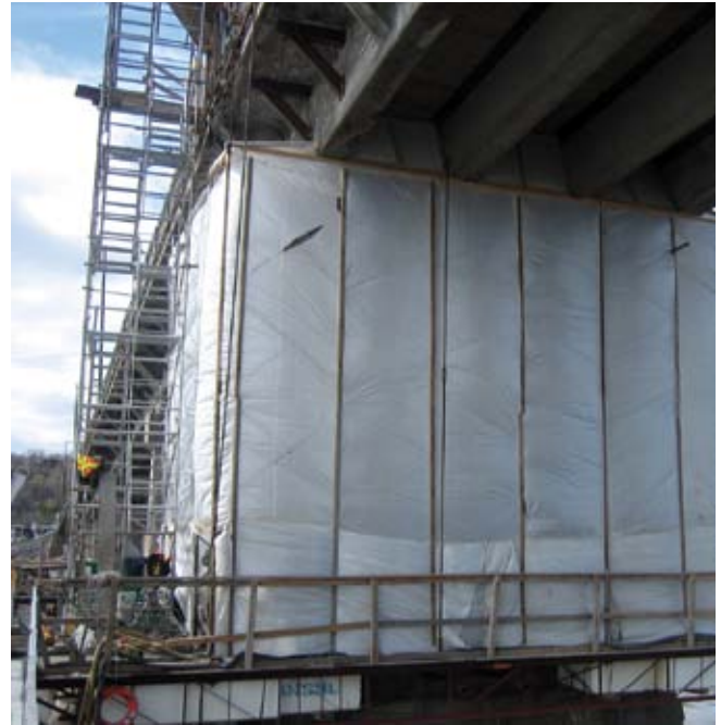
The shotcrete workspace was protected from wind, while also preventing dust and debris from falling into the river
