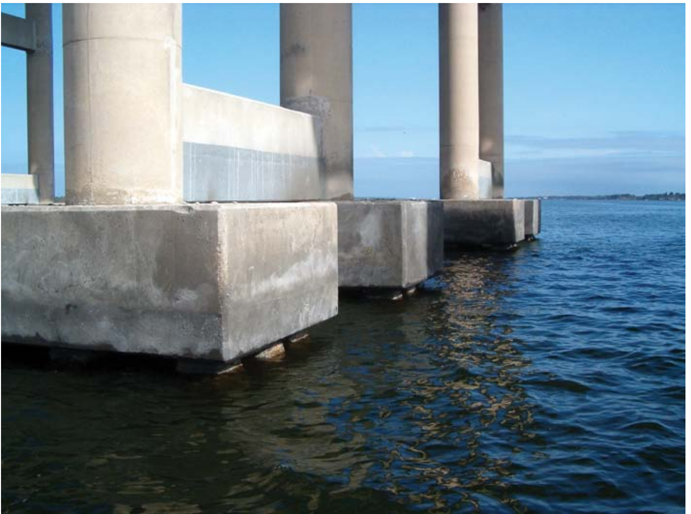
Completed low water pile caps
