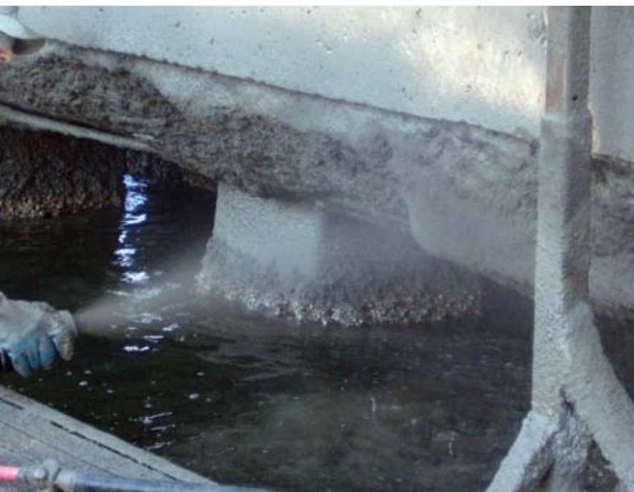
Dry-mix shotcrete can be placed slowly to reduce fallouts
