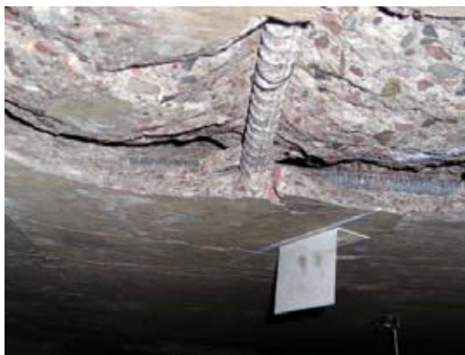
Crack in roof
