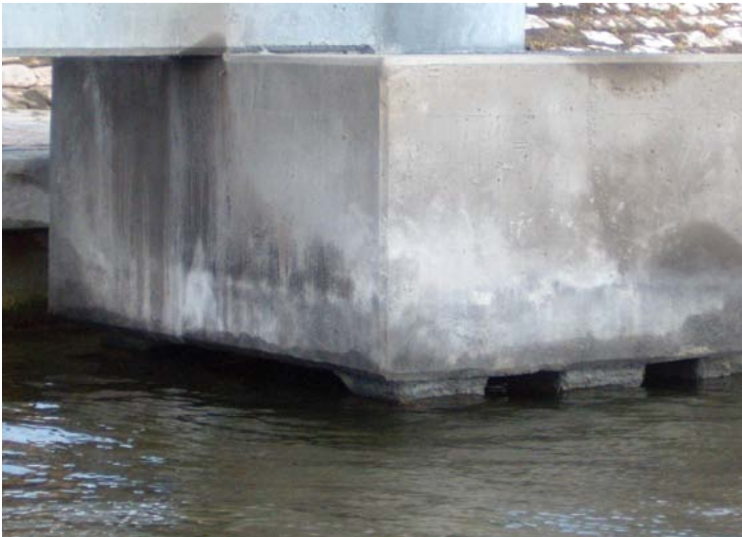
Close-up of reinstalled chamfers
