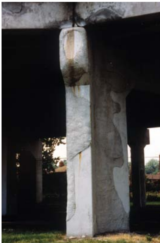
Until 1989, the MTO specification allowed for site mixing, which often led to inconsistencies in mixture proportions. Inconsistent cement contents would often lead to high shrinkage values, which contributed to cracking and debonding
