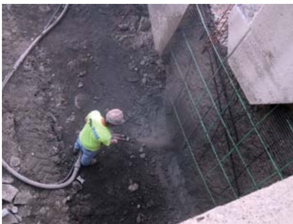
The structure required a significant number of repairs, some of which required up to 14 in. (356 mm) of concrete replacement
