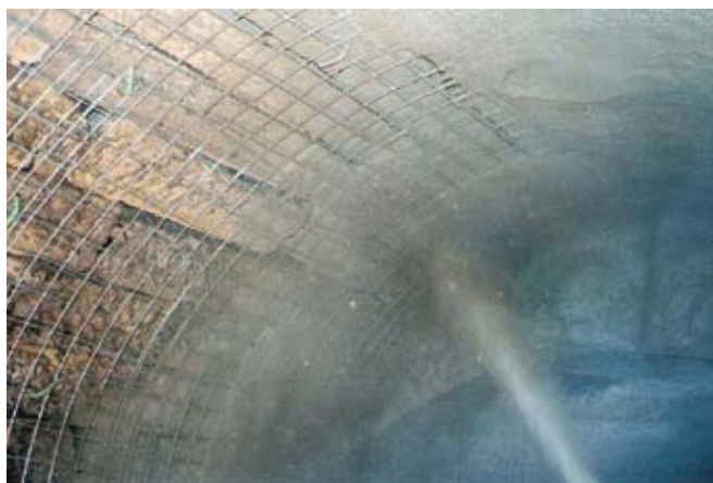
The dry-process shotcrete in this tunnel reline is gunned overhead to the full desired depth without layers
