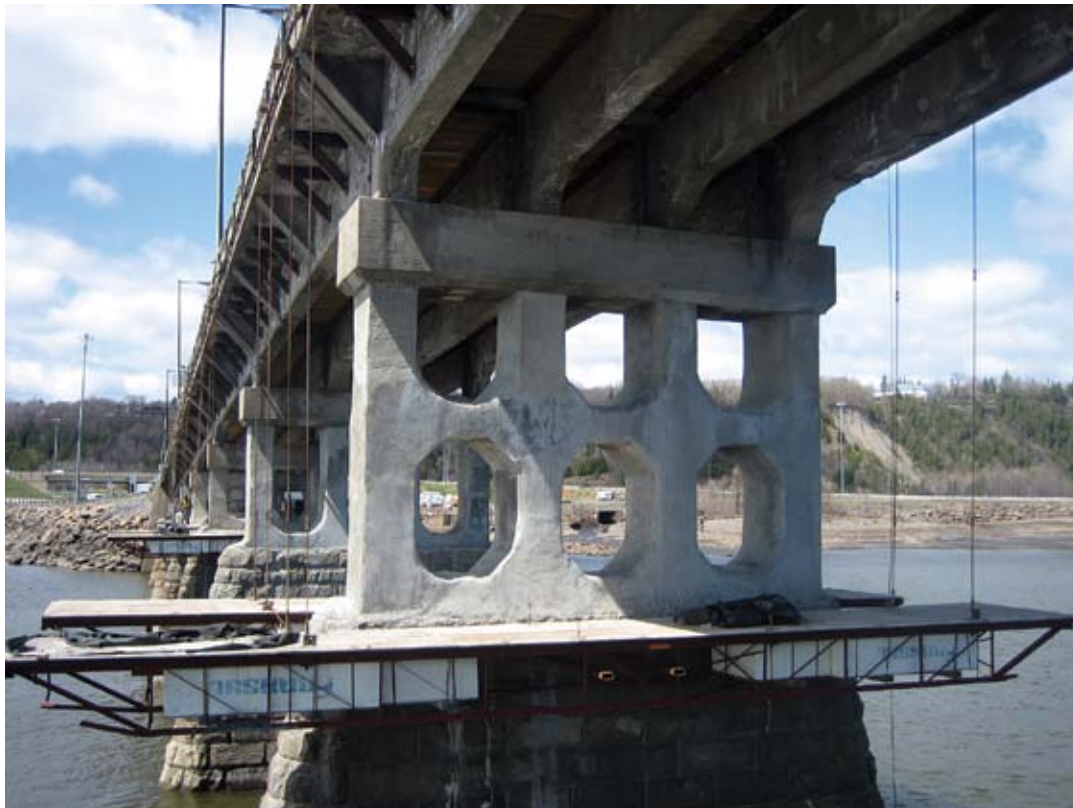
A finished repair is visible, with a support platform in place for final touches and inspection
