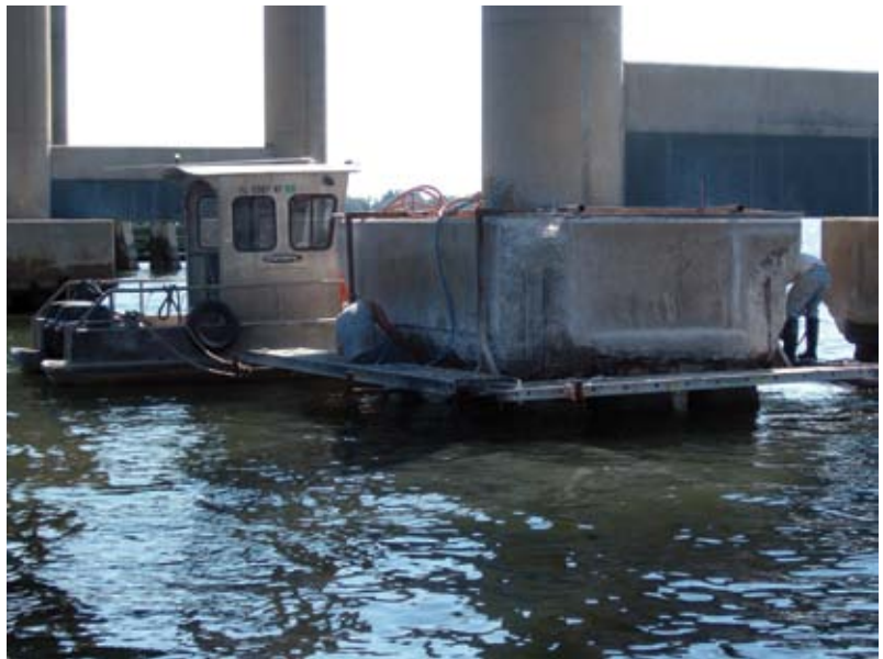
Removal of spalled concrete from pile caps
