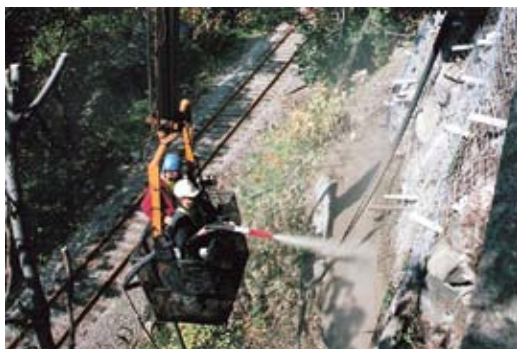
On this slope protection project, the dry-process shotcrete material is gunned to the full necessary depth in one pass
