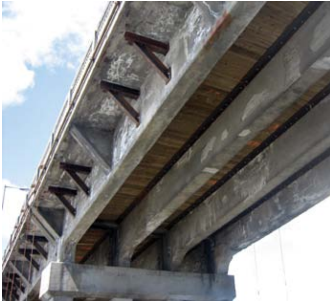
The concrete beams and timber deck are clearly visible, showing how various materials can work together. Some salt stains, corrosion, and freezing-and-thawing damages show how materials age
