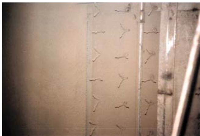
In this power plant ash hopper, the refractory, on the left, is gunned to the full 9 in. (229 mm) depth in one application. The ungunned area with the "V"-type refractory anchors is to the right
