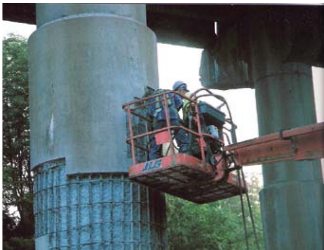
The deteriorated concrete on this bridge pier is removed to behind the first layer of reinforcing bar to allow the shotcrete to fully encapsulate the reinforcing bar
