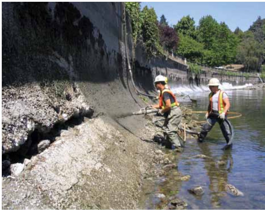
Fig. 5: Shotcrete repairs to damaged concrete faces rip-rap in the Devonian Park part of the Stanley Park Seawall in Vancouver, BC, Canada Photo courtesy of D.R. Morgan
