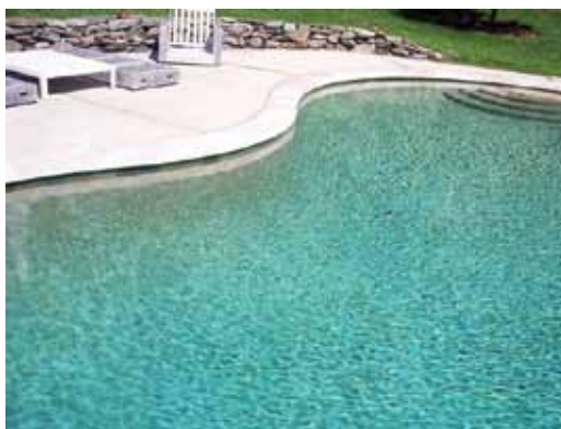
A dry shotcrete pool completed in the late 1960s with no proofing, sealants, or plaster (new tile and coping but original pool structure and surface)
