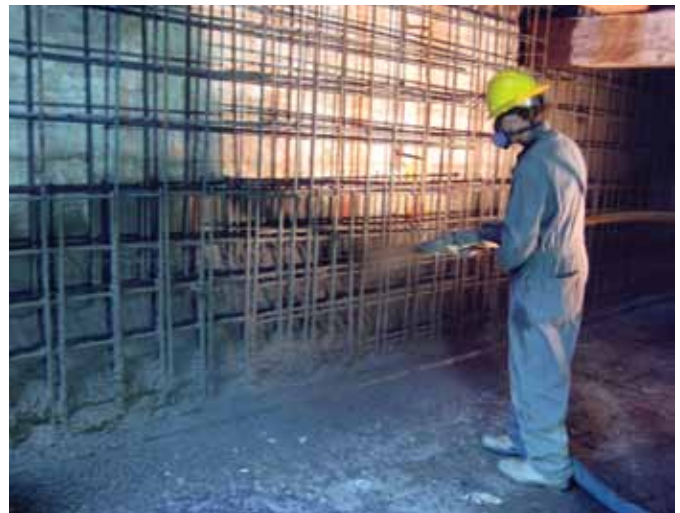
Fig. 2: Shotcrete applied to a masonry wall for seismic retrofit for a heritage building in Vancouver, BC, Canada
