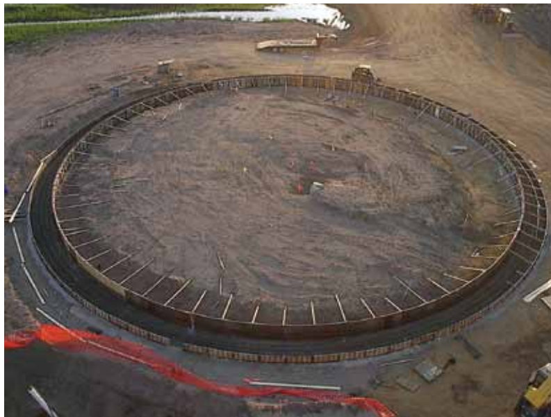
Fig. 1: Construction of a typical dome foundation
