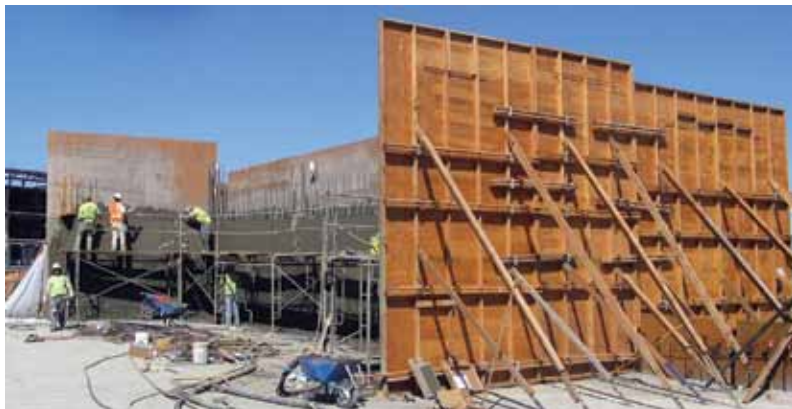
Fig. 1: Single-sided plywood formwork set up as a shotcrete receiving surface in California
