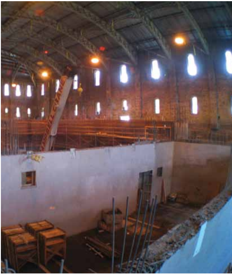
Fig. 5: Shotcrete after stripping forms
