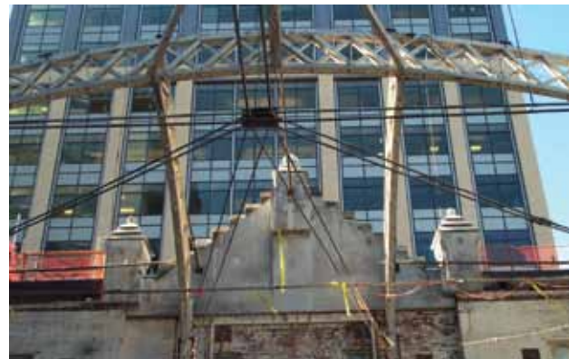
Fig. 2: Structure stabilization
