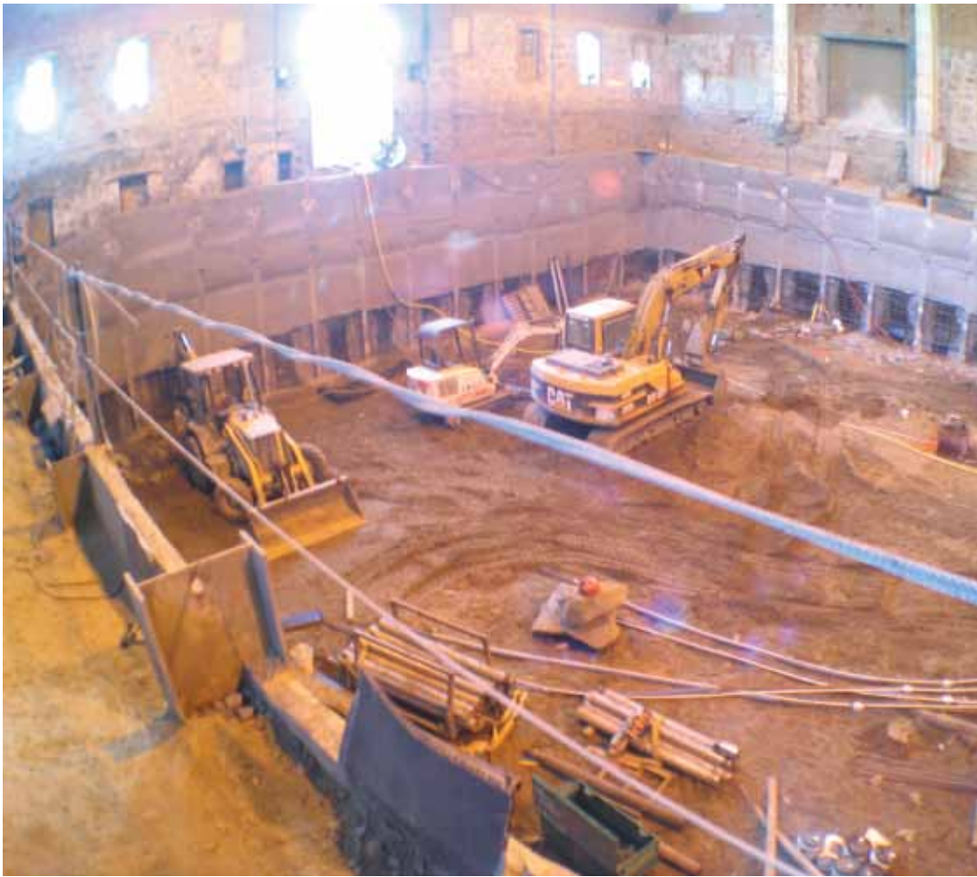
Fig. 3: Shotcrete soldier pile shoring
