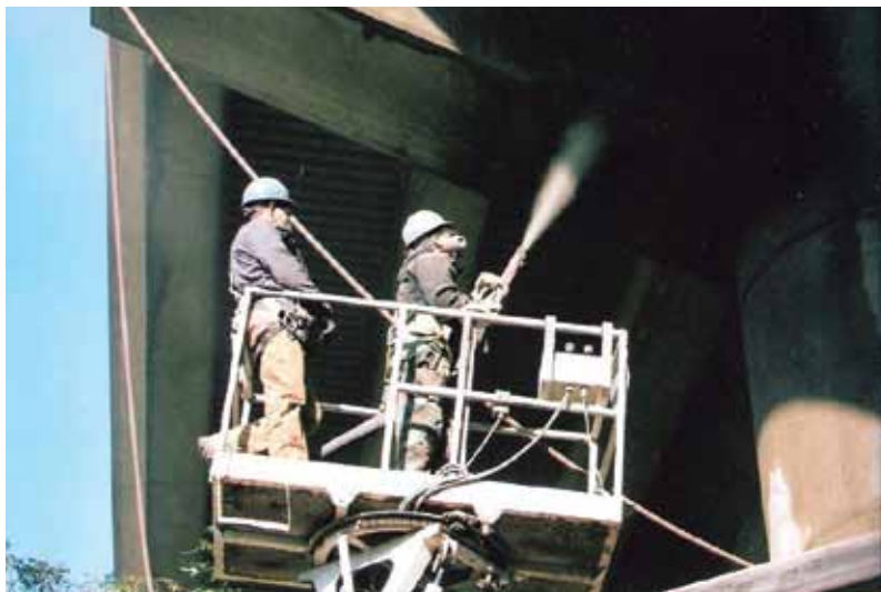
Overhead shotcrete repair on a bridge pier near Pittsburgh, PA, provides a cost-effective repair to existing structures that can prolong the life of the structure
