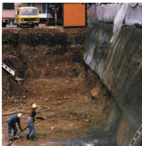
Fig. 2: Slope stabilization
