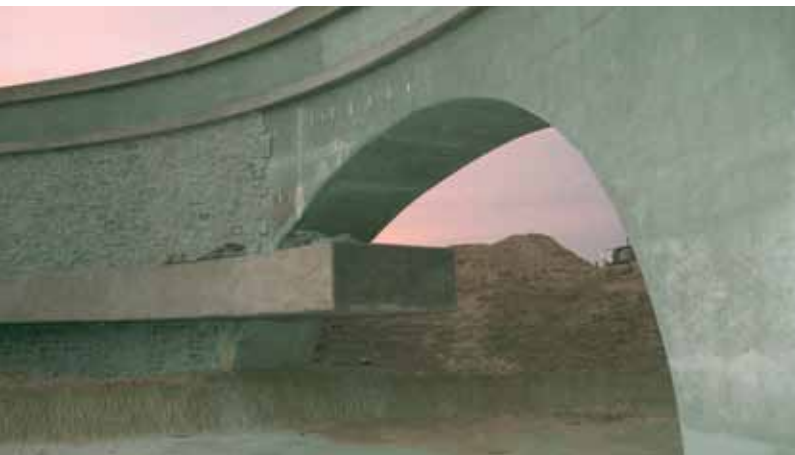
The sign wall with veneer being applied. Note the detail at the top with the sill, cap, and the 10 ft (3 m) long x 6 ft (1.8 m) wide x 2 to 4 in. (51 to 102 mm) thick cantilevered sill, all done with integral colored shotcrete
