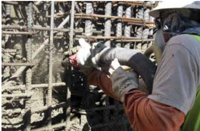
Fig. 4: Example of heavily congested reinforcement
