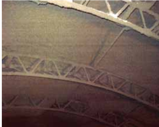
Lattice girder tunnel supports within the layers of fiber-reinforced shotcrete (initial layer)
