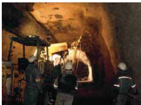
Fig. 1: Shotcrete application following contours of the tunnel
