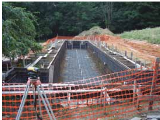
A residential pool prior to the shotcrete process. Pipes are capped and pressurized to ensure the system has no leaks
