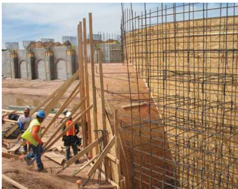
The two sign walls presented numerous forming challenges. This is a 6 ft (1.8 m) thick wall with an arched opening within a curved section
