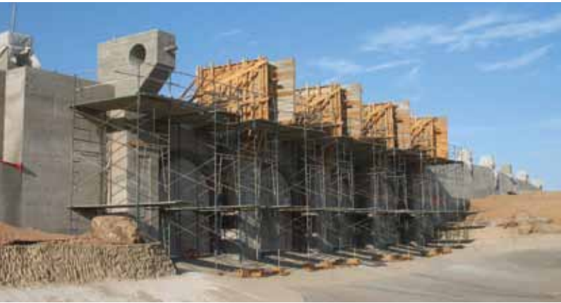
Access for forming the water column crowns was from scaffolding 20 ft (6 m) off the ground on both sides of the wall
