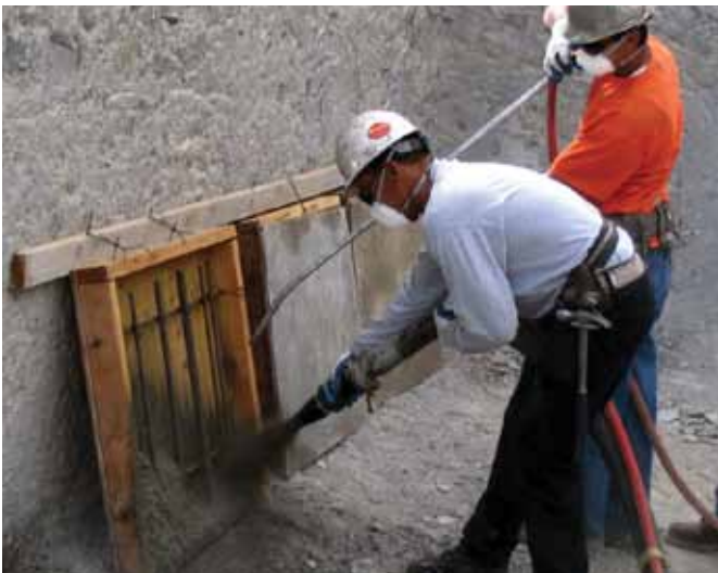
Fig. 1: The ACI vertical test panel contains a single mat of reinforcing spaced with noncontact lap splices at 3.5 in. (89 mm) thickness
