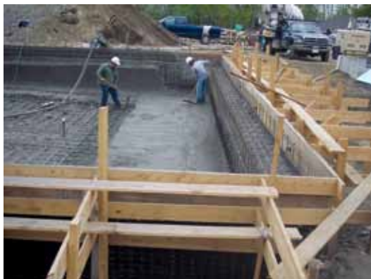
This is a straight, solid formwork and steel application of concrete being placed and is one of the items on the check list for proper placement
