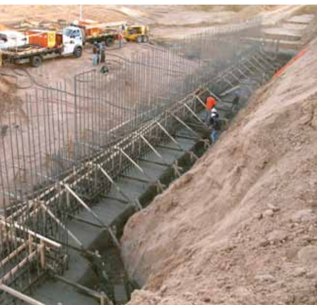
Shotcrete being placed for one of the faux bridge retaining walls. A total of 180 yd 3 (138 m 3 ) were placed in one shift for each of these massive footings
