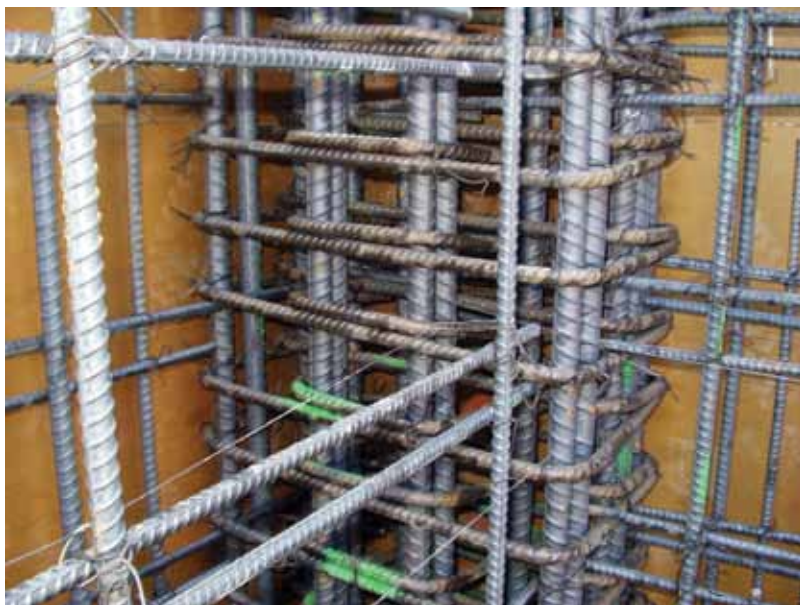
Noncontact splices used in open area boundary element done with contact splices for better access
