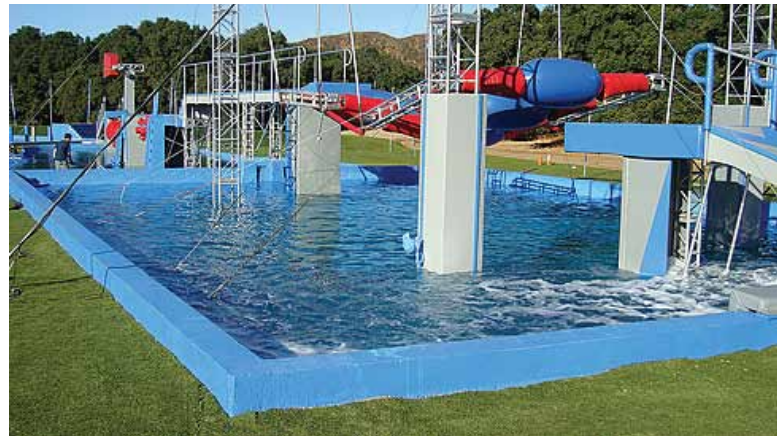
Pool shotcreted with vertical walls using no forms
