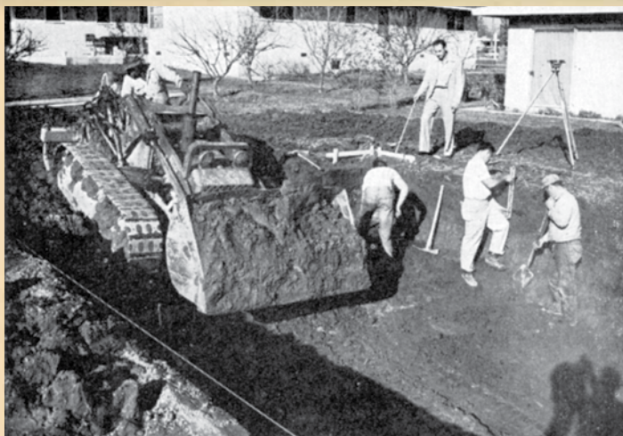
Excavation being done here with a Hough Payloader; which ramps out of shallow end of pool. Proper setting of forms and excavation are two crucial operations
