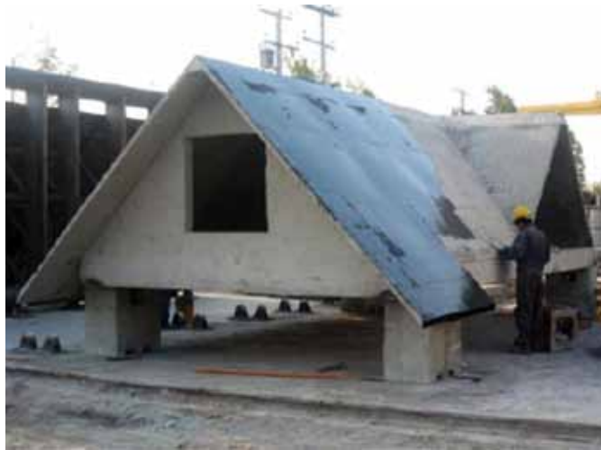
A Tekcrete™ roof module—a monolithic structure
