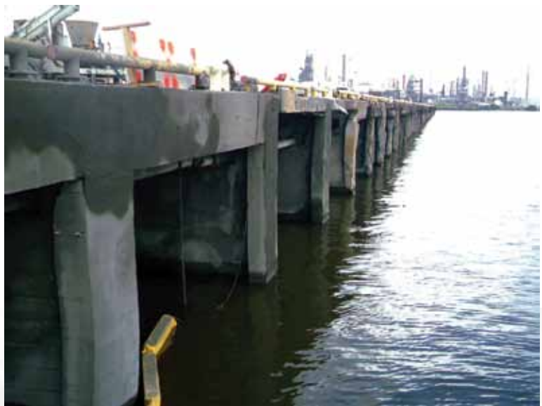
Manchester Terminals dock begins to find new life as shotcrete application progresses
