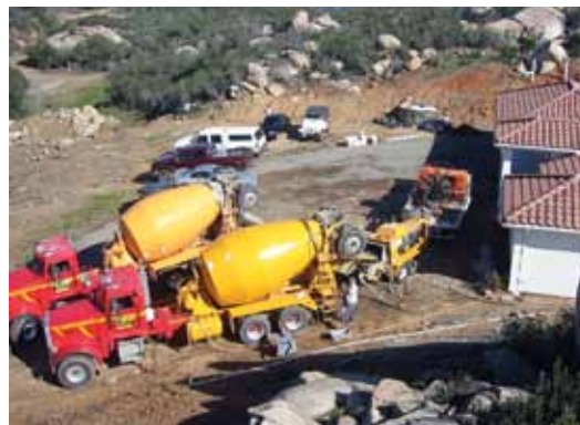
REED C50HP set up and wet-mix shotcrete being pumped for pool construction in Southern California
