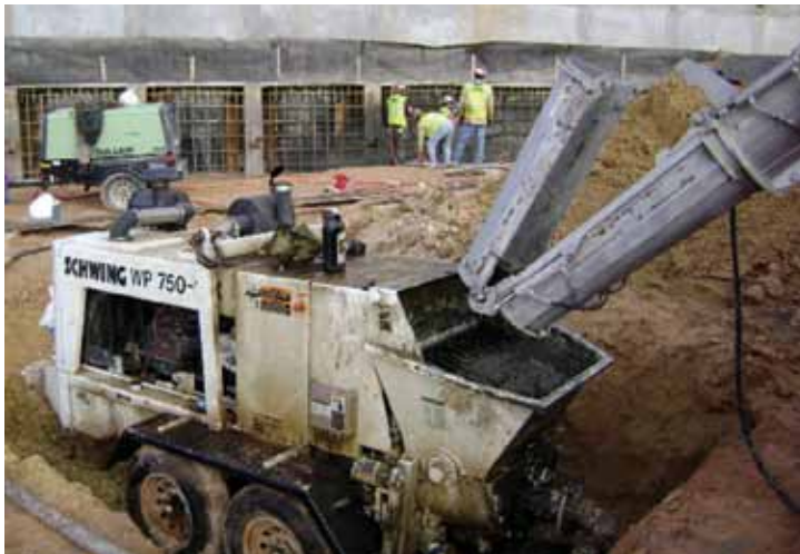
Fig. 5: A Schwing 750 trailer pump that was set up for easy maneuvering in and around the job site
