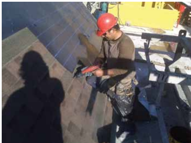
In-factory shingling of a Tekcrete roof module
