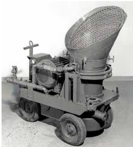
Fig. 5: Rotating-barrel gun (Meyco GM 57, No. 1)
