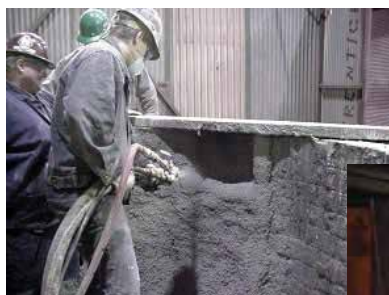
Stainless steel fibers are added to the dry-mix bulk materials to be used for refractory shotcrete
