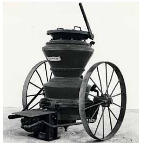
Fig. 2: Double-chamber gun (Cement-Gun, 1914)
