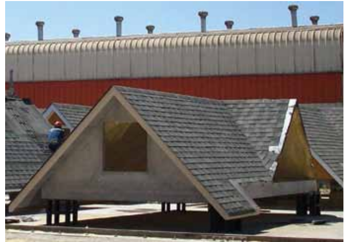
Shingled and insulated Tekcrete roof module ready for painting and window installation
