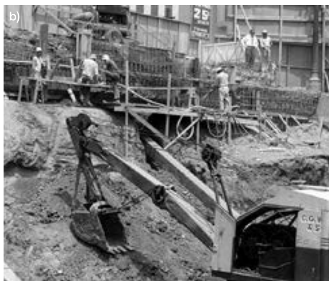
Shotcrete has been widely used for over a century: (a) a crew poses with their equipment in the 1920s; and (b) a crew places a foundation wall in the 1940s
