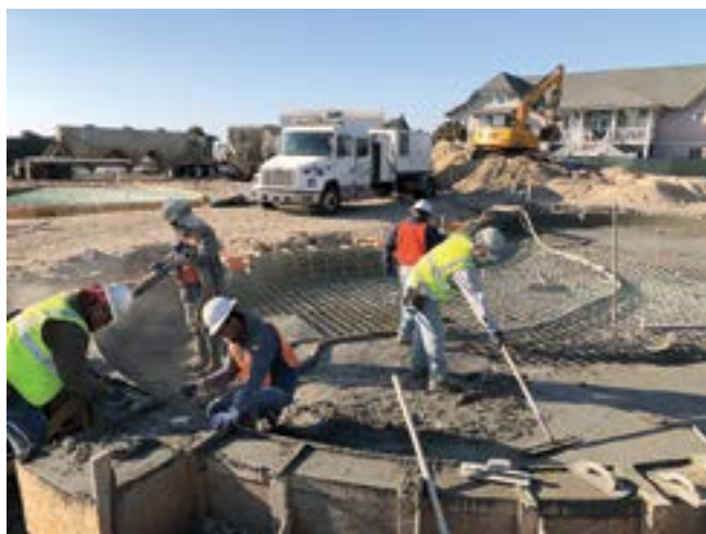
Fig. 2: Bald Head Island project: (a) transportation of Revolution Gunite's trucks, equipment, and materials; and (b) construction on the island
