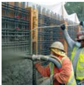
On the cover: A certified nozzleman and blowpipe operator constructing mockup panels for an enclosure wall. Photo courtesy of Joseph J. Albanese, Inc. Read the article on page 28, reprinted from the December 2019 issue of Concrete International.
