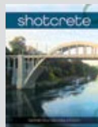
Repair and Rehabilitation
