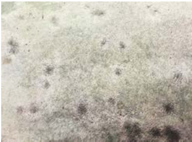
Fig. 8: Closeup view of shotcrete layer sprayed onto waterproofing membrane
