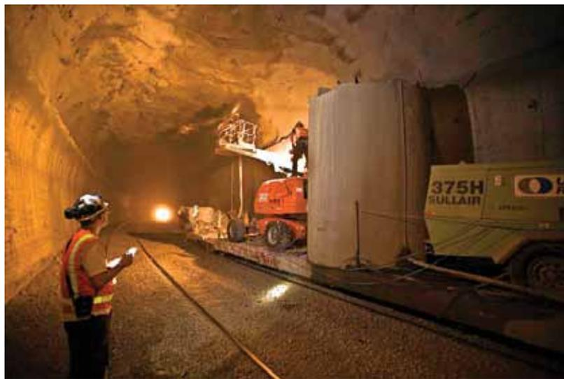
*Along the Heartland Corridor, Norfolk Southern has employed a number of methods to increase the clearance, including raising the roof and lowering the track. To expand the tunnels, workers must also transform the passageways' corners from rounded to squared, which allows the taller trains to pass*
