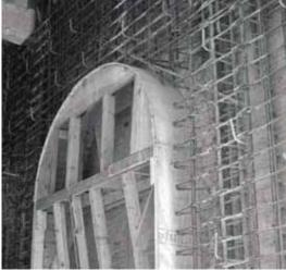
Wooden window form and reinforcement prior to receiving 12 in. (304.8 mm) of concrete
