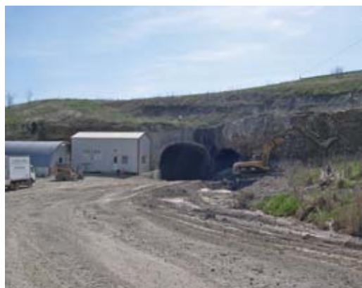
Fig. 6: Scaling loose rock from high wall
