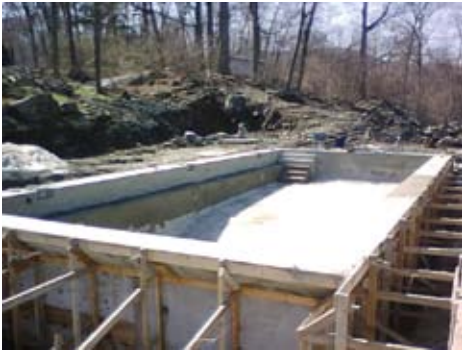
Pool shotcreted, waiting for forms to be stripped
