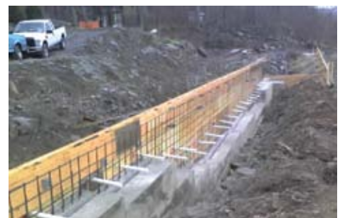
Wall footings with wall forming and steeling completed
