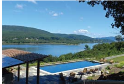
Finished pool and walls looking northwest across the Hudson River
