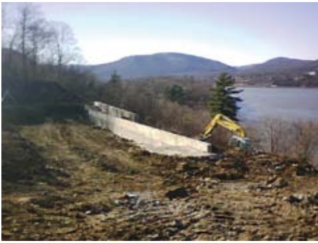
Shotcrete walls in place before being backfilled
