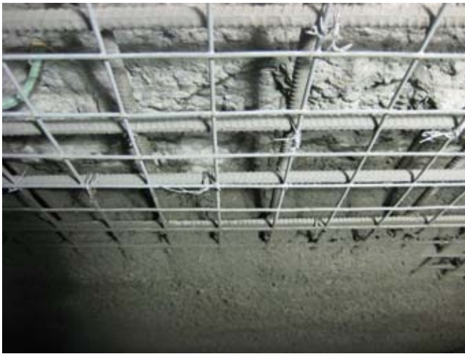
Shotcrete encapsulating the reinforcing bar
