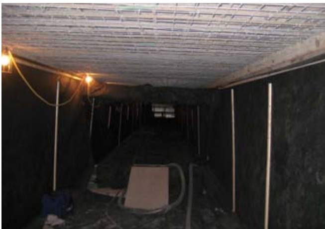
Underside of deck ready for shotcrete placement
