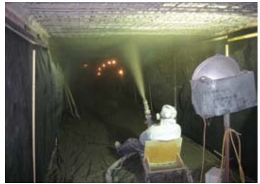
Nozzleman in cramped quarters
