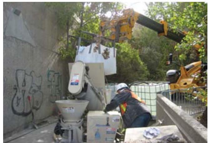
Equipment setup. Bulk bags were used
