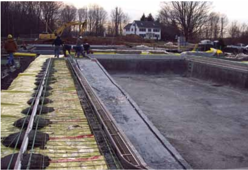
Stainless steel gutter installation
