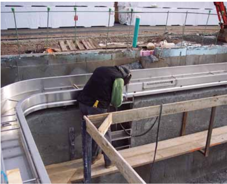
Radius gutter installation above radius shotcrete corner
