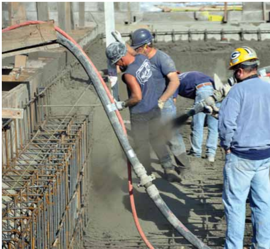
Shotcrete phase of the lap pool
