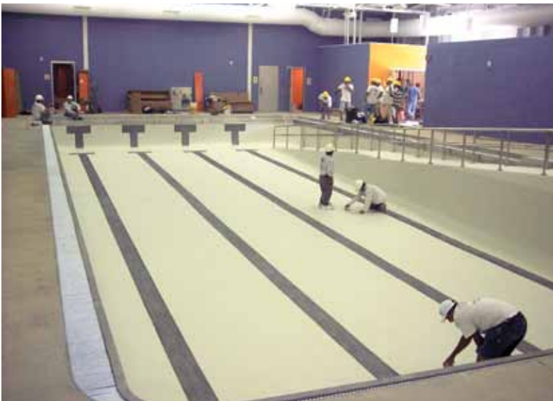
Tested plaster installation over watertight concrete
