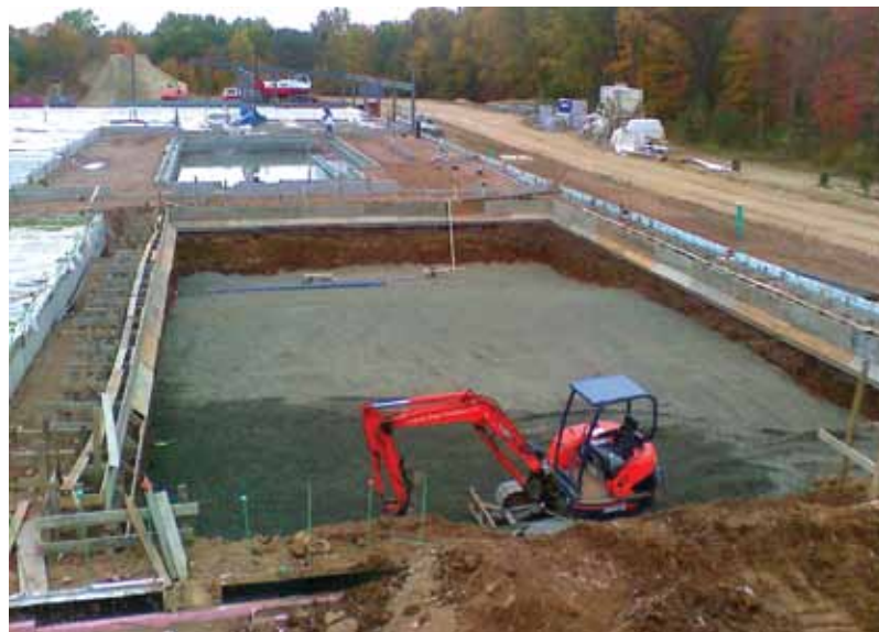
Foreground: competition pool using sustainable formwork in forming and excavation phase. Background: watertight lap pool in curing phase
