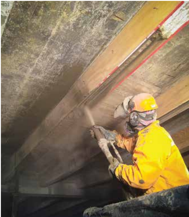
Fig. 3: Shotcrete application on the 18,000-bag Pickwick Condo project in Kansas City.
