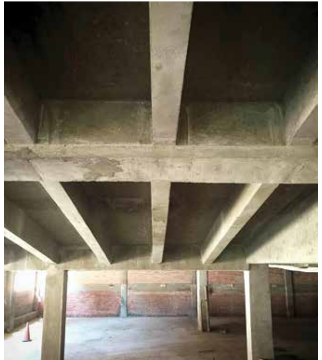
Fig. 4: The Pickwick Building parking garage, featuring SpecShot Plus
