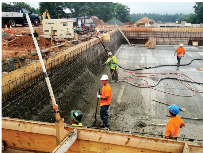
Fig. 1: Floor cast with installed keyway
