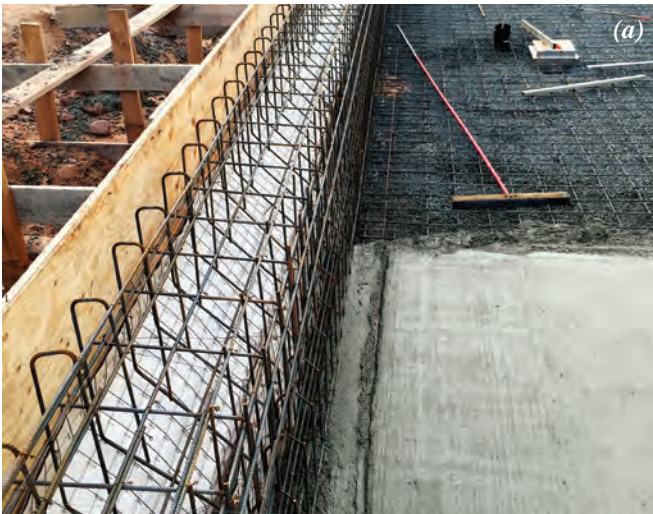
Fig. 1: Floor cast with installed keyway
