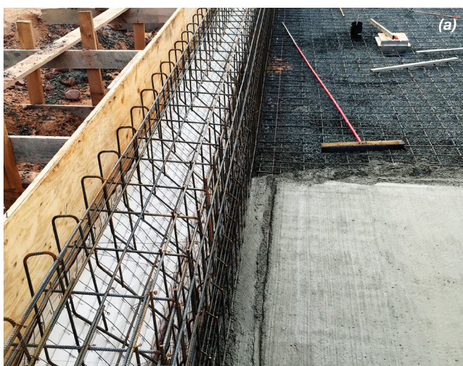
Fig. 1: Floor cast with installed keyway
