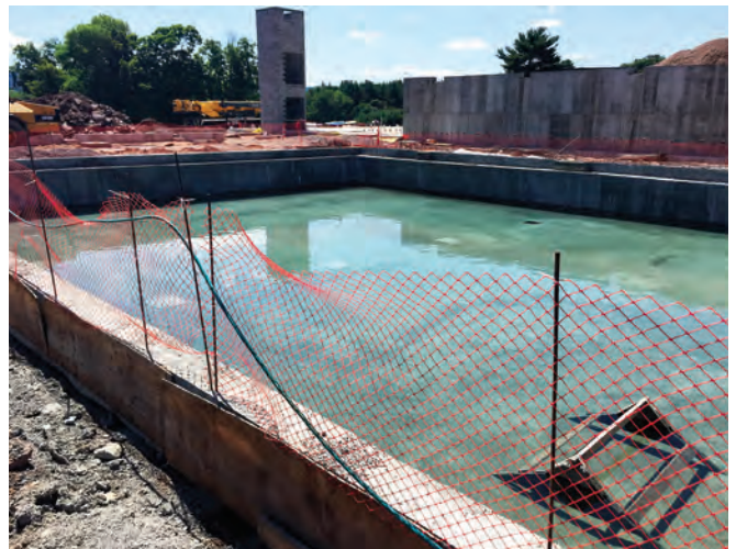
Fig. 3: Watertight tank test
