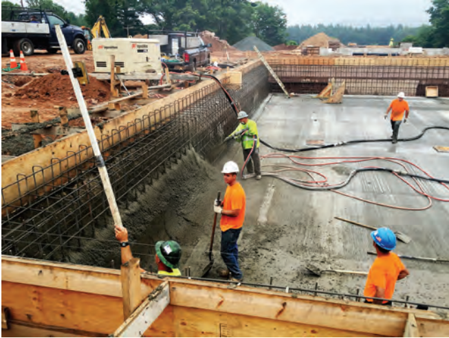
Fig. 1: Floor cast with installed keyway
