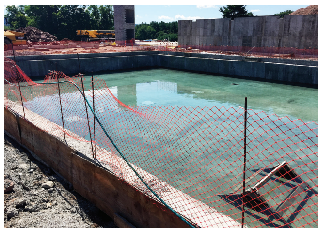
Fig. 3: Watertight tank test
