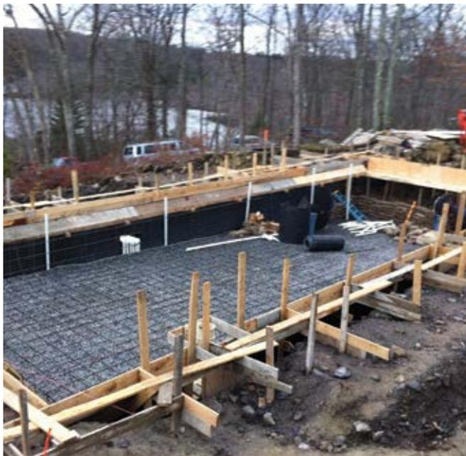
Fig. 1: Lightweight, one-sided form is all that's needed when using shotcrete
