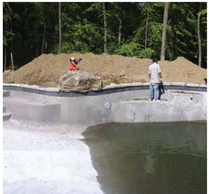
*Fig. 4: Using shotcrete makes curved concrete pool surfaces easy*
