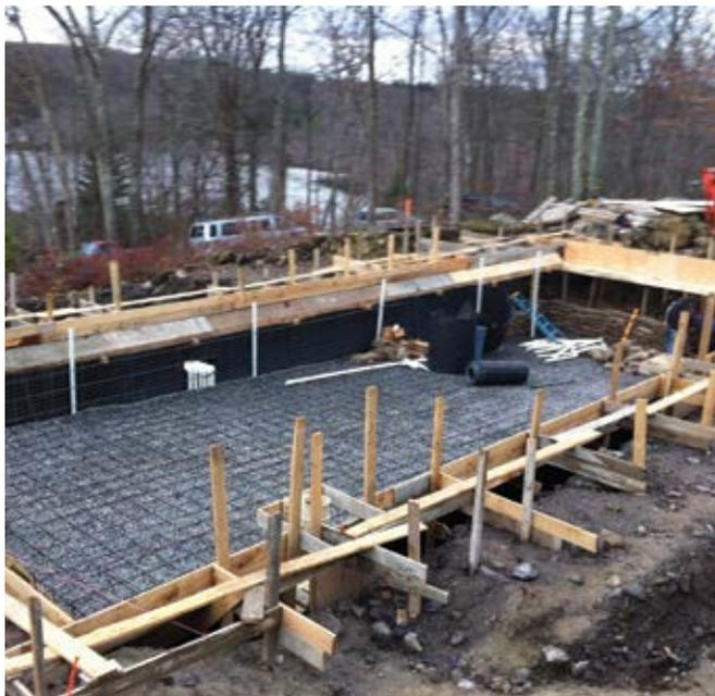
Fig. 1: Lightweight, one-sided form is all that's needed when using shotcrete
