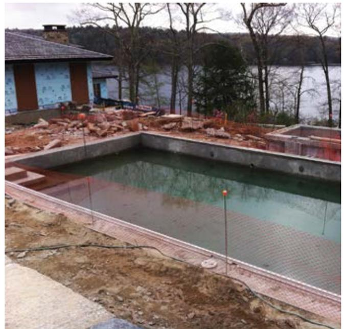
Fig. 2: Pool shell is in place. Ready for the pool deck
