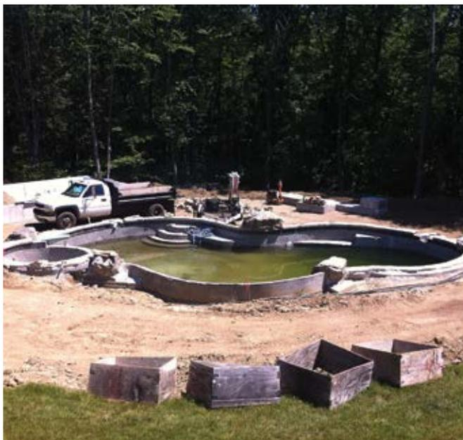
Fig. 3: Overview of a pool with extensive curves typifying shotcrete's flexibility
