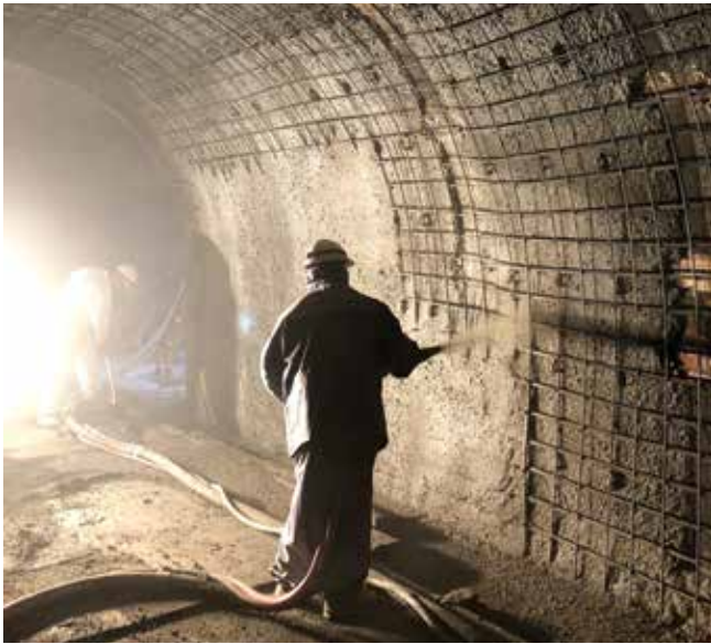
Fig. 9: Placement of second layer of shotcrete
