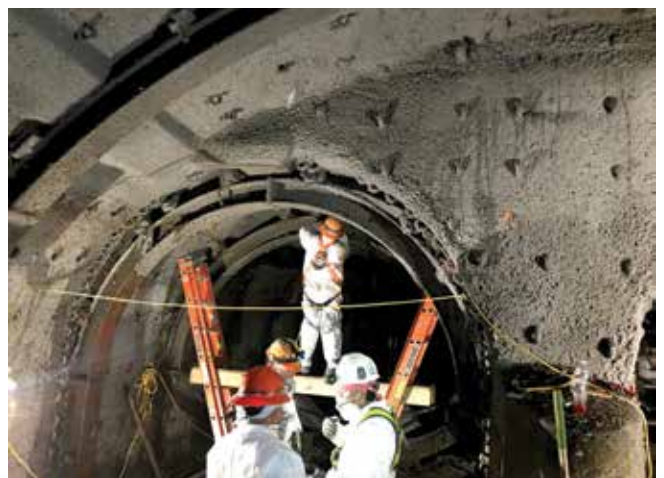
Fig. 2: Removing preexisting bents
