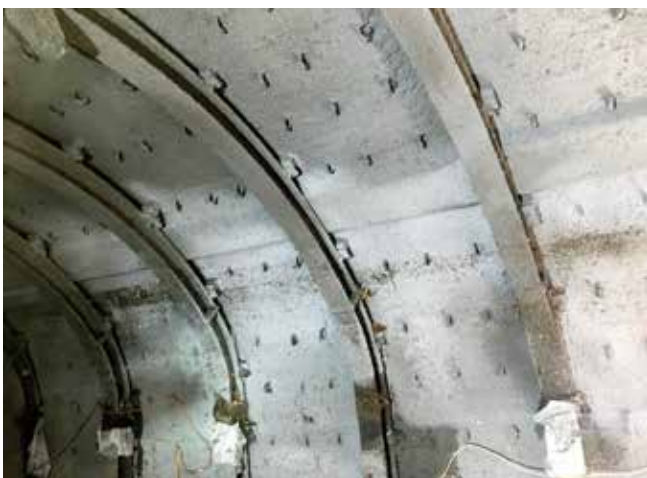
Fig. 1: Installing first shotcrete layer
