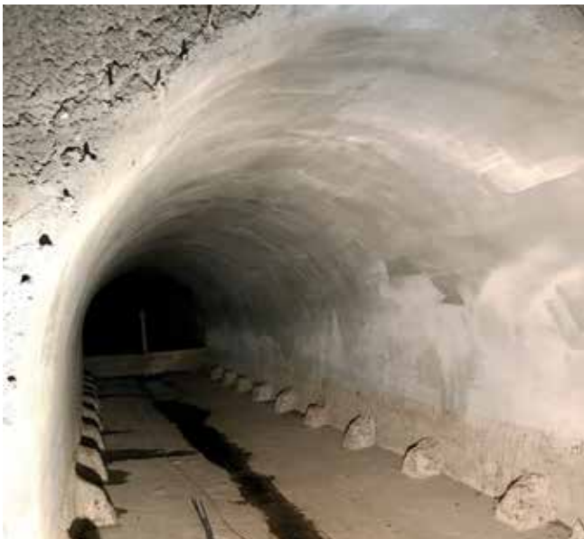
Fig. 10: One barrel of double barrel section completed
