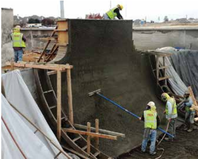
Fig. 7: Final shaping of transitional surface with pole tools
