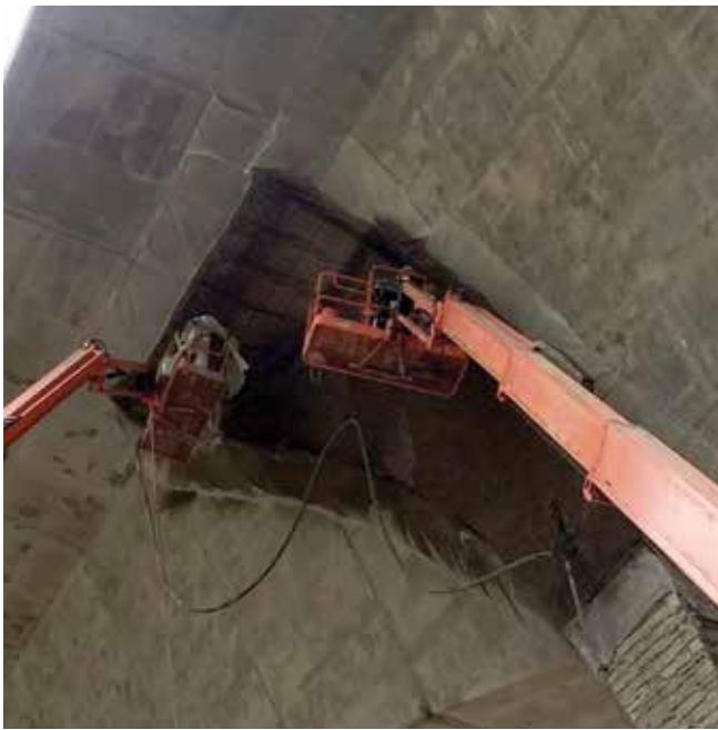
Fig. 5: First day shooting a fin, bringing shotcrete just past the reinforcing bar
