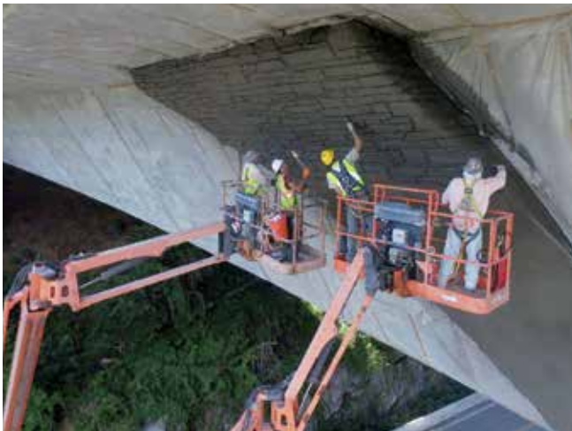
Fig. 6: Second day of shooting a fin, flash and sculpt the rock face
