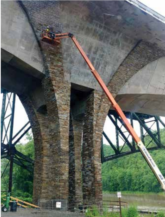
Fig. 8: Staining the piers
