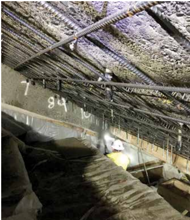
Fig. 23: Nozzlemans ready to begin shotcrete application to prepared concrete substrate
