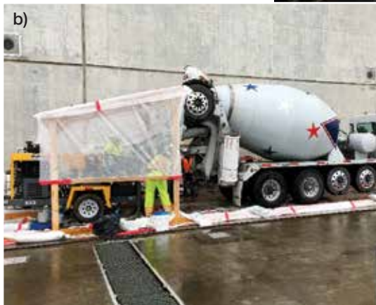
Fig. 14(a) and (b): Shotcrete pump and supply setup outside powerhouse
