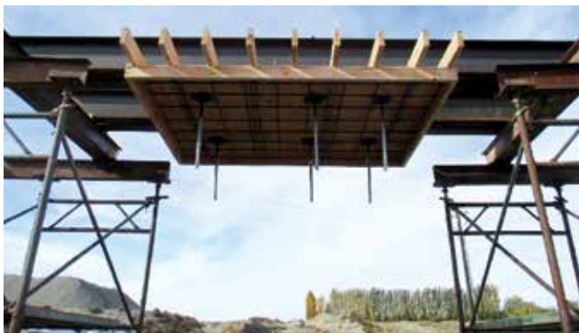
Fig. 6: Start of preconstruction mockup construction
