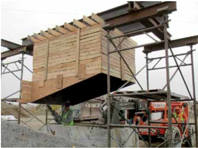
Fig. 9: Nozzleman shooting final lift of full-scale mockup
