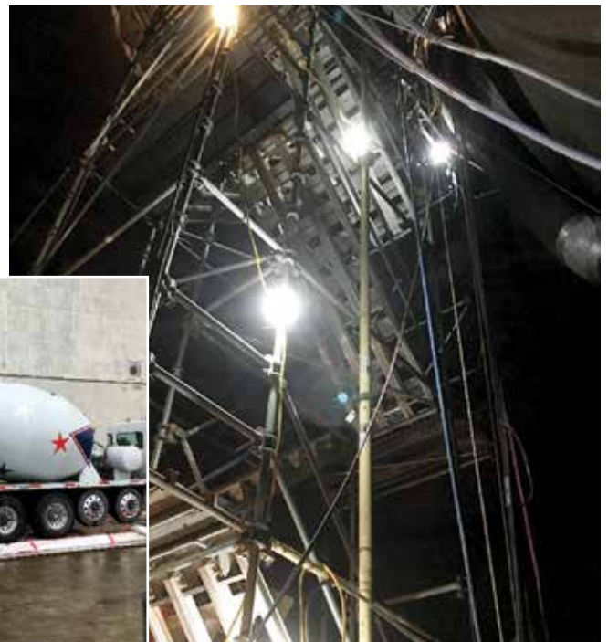
Fig. 16: Steel line entering shotcrete application area inside draft tube
