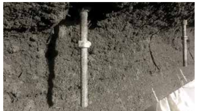
Fig. 21: A 1/2 in. anchor embedded in shotcrete
