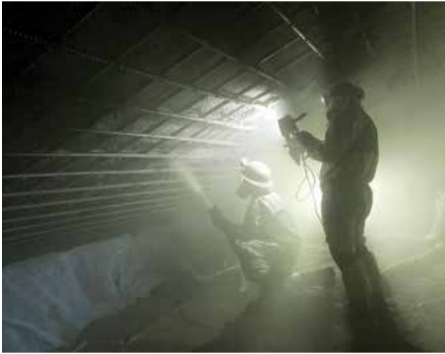
Fig. 24: Nozzleman shooting dry-mix shotcrete at the No. 9 reinforcing bar
