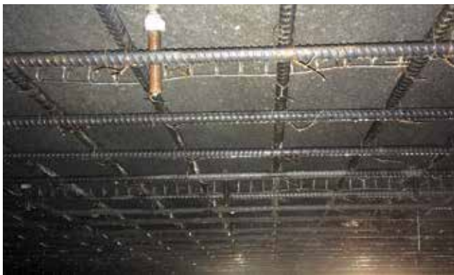
Fig. 22: Number 9 reinforcing bars installed and ready for shotcrete application
