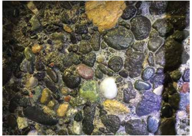
Fig. 18: ICRI CSP7 surface roughness profile
