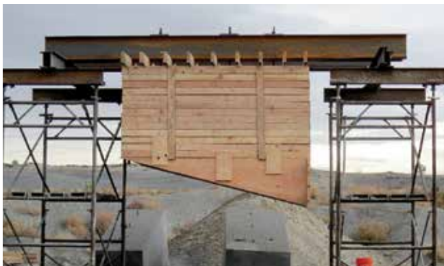
Fig. 8: View of preconstruction mockup after completion of installation of wood forms
