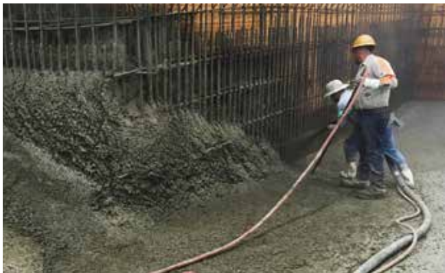
Fig. 3: Wet-mix shotcrete was used on this pool because of the congested reinforcing bar layout, as well as requiring about 300 yd 3 (230 m 3 )
