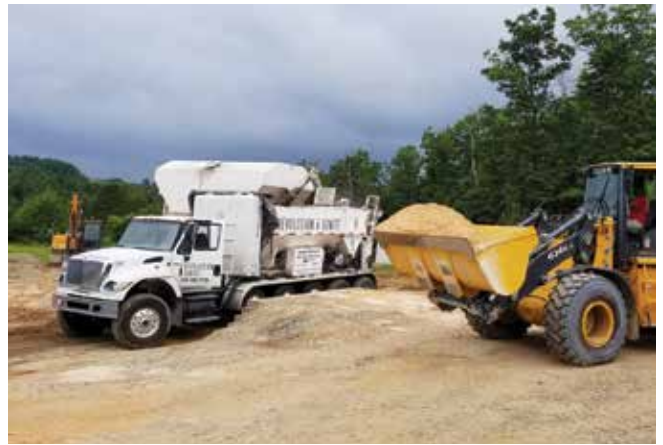
Fig. 1: Volumetric mixer truck on a pool shoot
