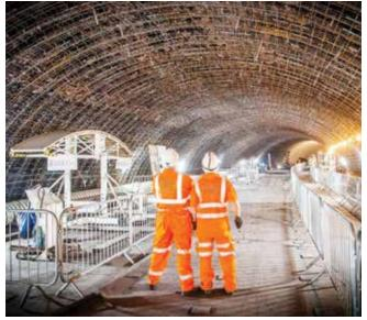
Fig. 5: 990 RAM Arch reinforcement units installed. Bespoke arch lifting machine shown to the left
