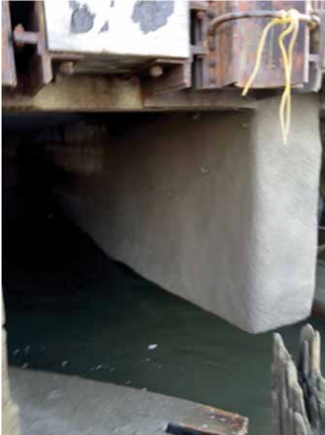
Fig. 6: A completed severe girder repair shot with a gun finish
