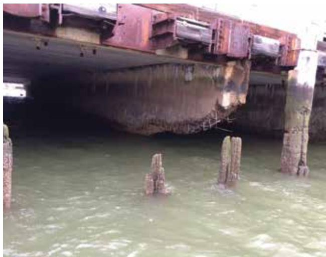
Fig. 1: An example of a moderate girder repair
