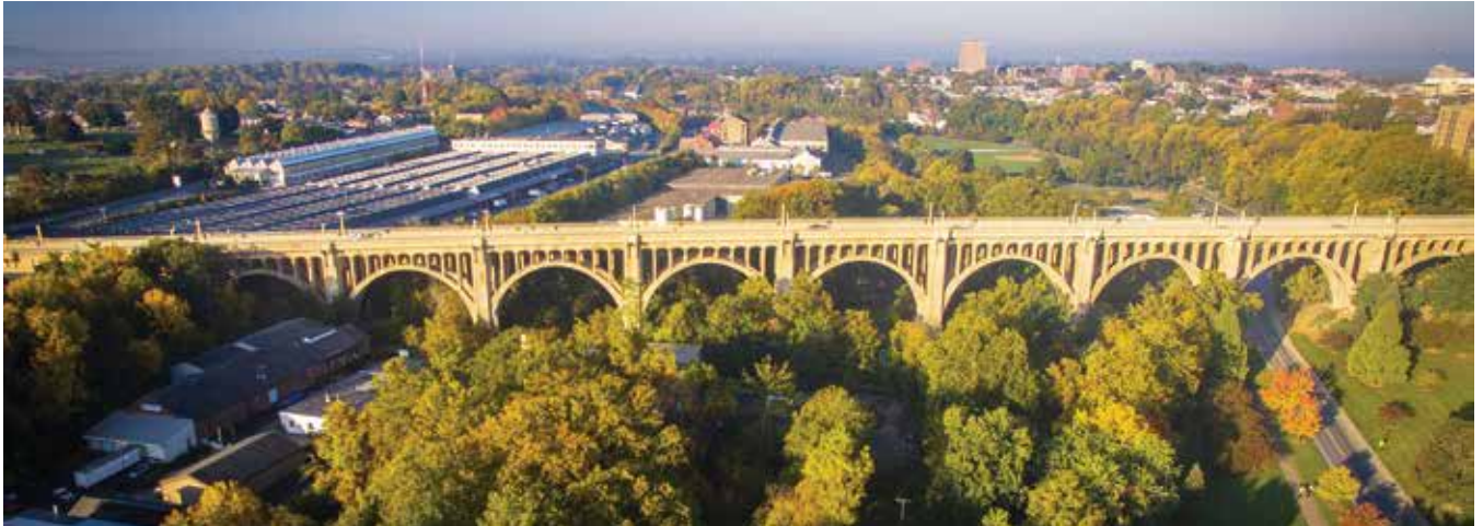
Fig. 1: November 2016—view of entire bridge after repairs were completed
