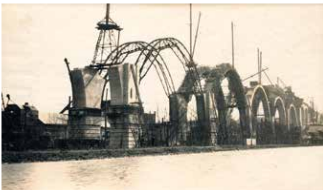
Fig. 2: January 1913 construction progress
