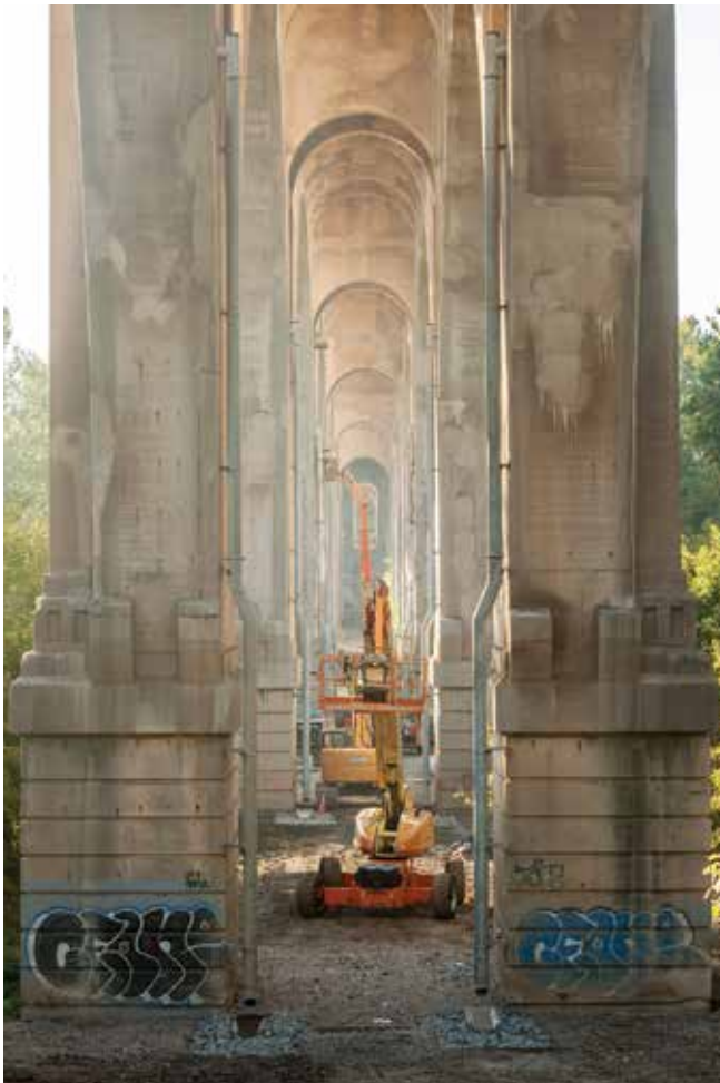
Fig. 7: Looking through piers—shotcrete on an arch rib
