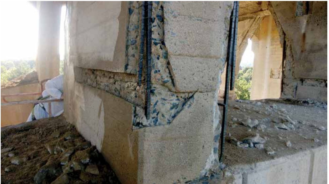
Fig. 6: Spandrel column repair with chipping complete
