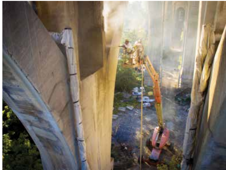
Fig. 4: Shotcrete in progress at a pier
