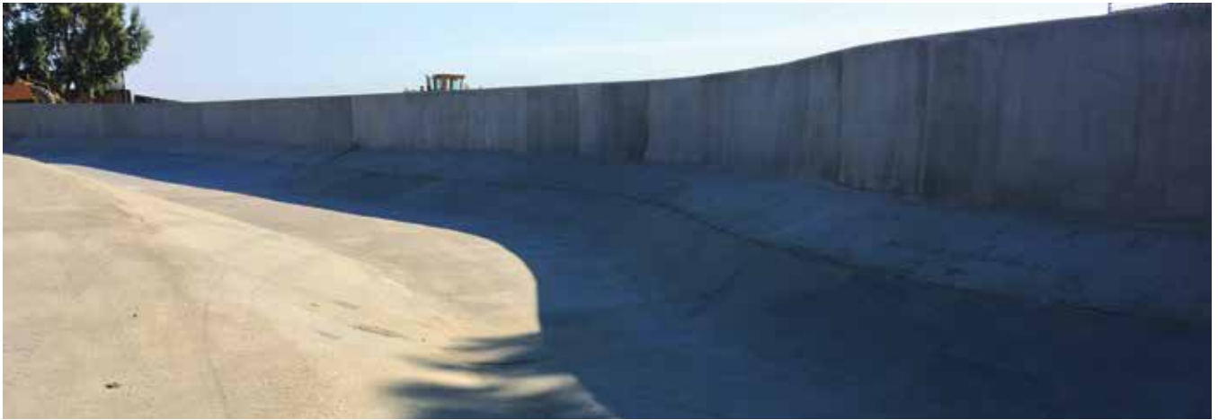
Fig. 3: Completed north wall
