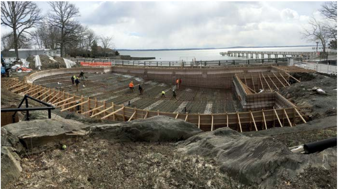
Fig. 2: 50 tons (45 metric tons) of reinforcing bar being installed
