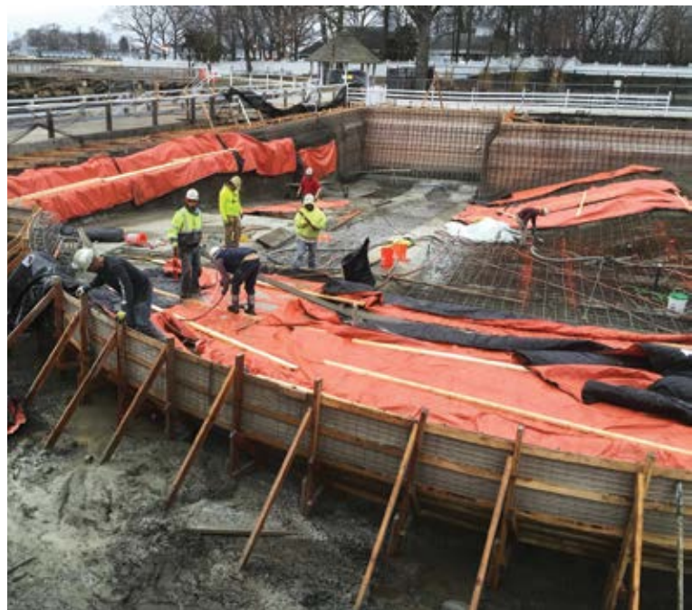
Fig. 4: Covering with thermal blankets to protect from freezing
