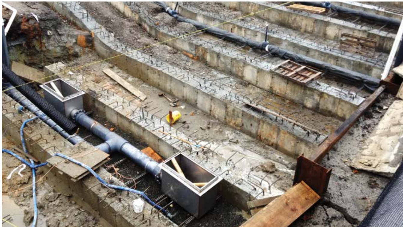
Fig. 1: Grade beams installed and under-pool piping being installed between grade beams
