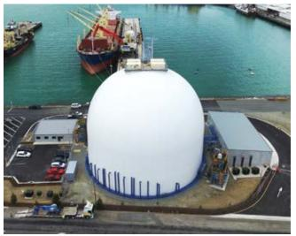
Fig. 2: Aerial view of Holcim Cement Terminal in Timaru, New Zealand. Dome is 118.1 ft (36 m) in diameter and 103.3 ft (31.5 m) tall and stores 33,000 tons (30,000 tonnes) of cement powder and used 1923 yd<sup>3</sup> (1470 m<sup>3</sup>) of shotcrete to construct
