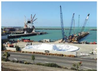
Fig. 6: Timaru dome air form ready for inflation. The DomeSkin™ air form is 38,350 ft<sup>2</sup> (3563 m<sup>2</sup>)
