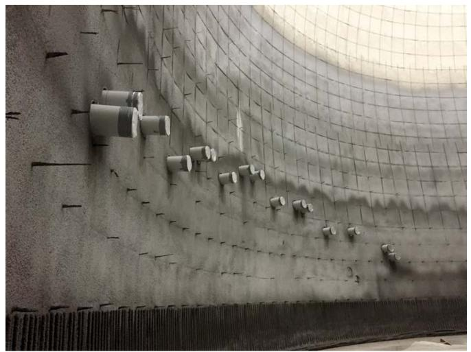
Fig. 7: First pass of shotcrete over first mat of structural bar. Both domes were completed on budget and ahead of schedule
