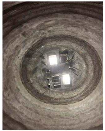
Fig. 4: View of dome apex from inside of dome. When completed, each apex was designed to support 150,000 lb (approximately 62 tons [68 tonnes]) without any interior supports
