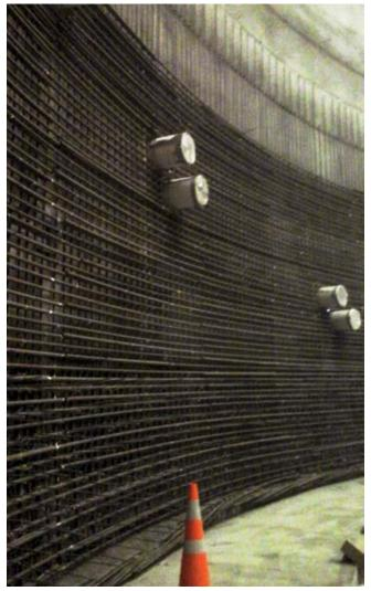
Fig. 8: Typical dome structural reinforcing bar mat; over 550 tons (500 tonnes) of reinforcing bar was used in the Timaru dome
