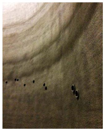
Fig. 5: Finished interior wall of dome. The dome used roughly 1923 yd<sup>3</sup> (1470 m<sup>3</sup>) of shotcrete
