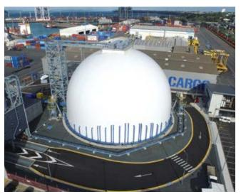
Fig. 1: Aerial view of Holcim Cement Terminal in Auckland, New Zealand. Dome is 135.2 ft (41.2 m) diameter and 90.2 ft (27.5 m) tall and stores 33,000 tons (30,000 tonnes) of cement powder and used 1400 yd<sup>3</sup> (1100 m<sup>3</sup>) of shotcrete to construct
