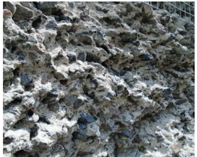
Fig. 2: Close-up of hydrodemolition concrete ready for shotcrete
