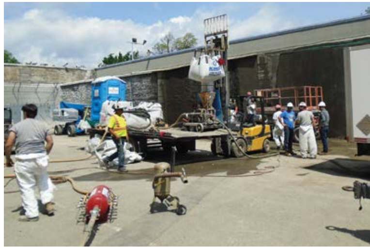
Fig. 8: Dry-mix shotcrete equipment setup on trailer
