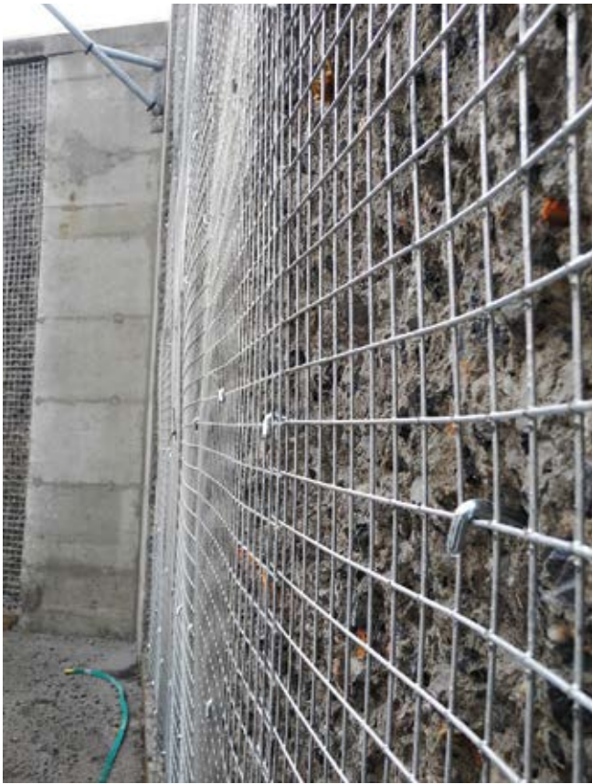
Fig. 4: Mesh installed using gunite hooks
