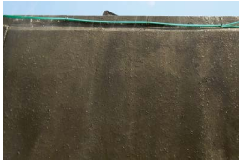
Fig. 6: Soaker hose used to cure the dry-mix shotcrete
