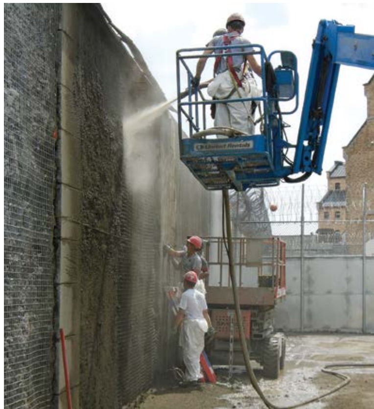
Fig. 7: Shotcrete application and finishers
