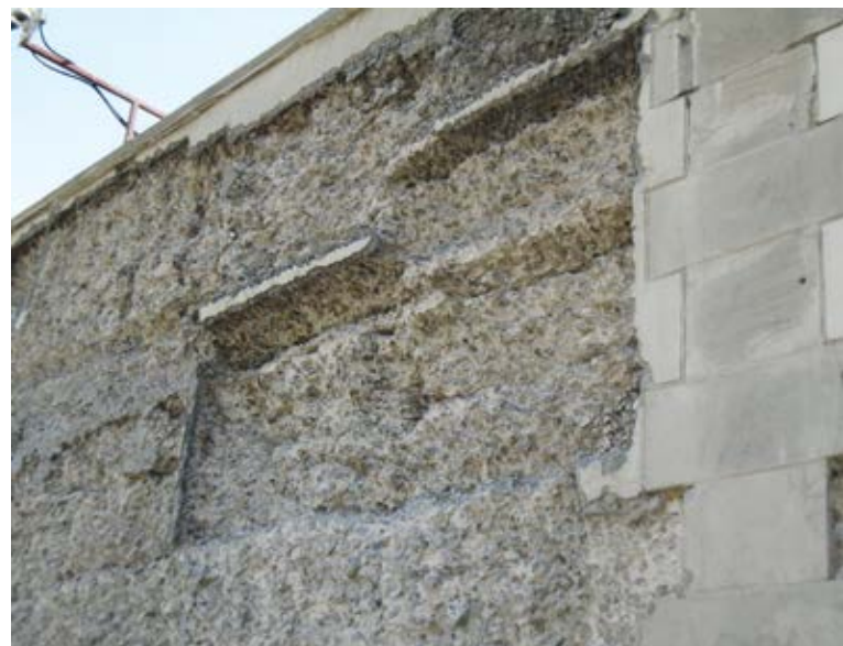
Fig. 3: Repairs ranging from 2.5 to 18 in. (64 to 450 mm)
