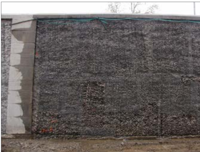
Fig. 5: Soaker hose creating a saturated surface-dry surface on area to be repaired
