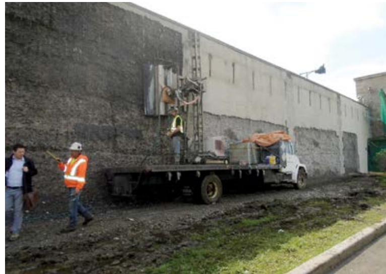
Fig. 1: Hydrodemolition machine setup
