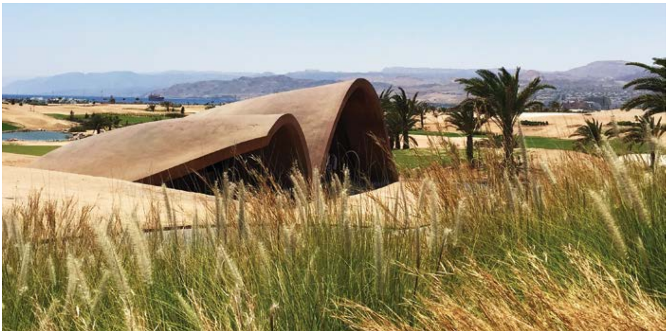
Completed Ayla Golf Comfort Station Photo credit: Oppenheim Architecture
