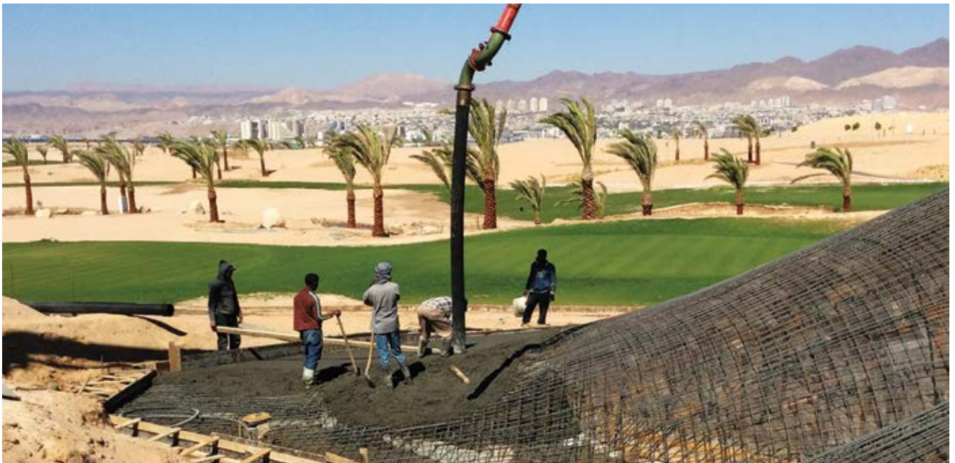
Ayla Golf Comfort Station shotcrete application Photo credit: Oppenheim Architecture
