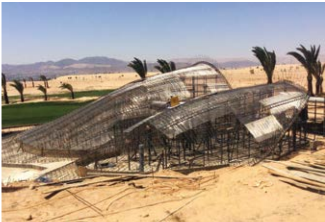
Framing the Ayla Golf Comfort Stations Photo credit: Oppenheim Architecture
